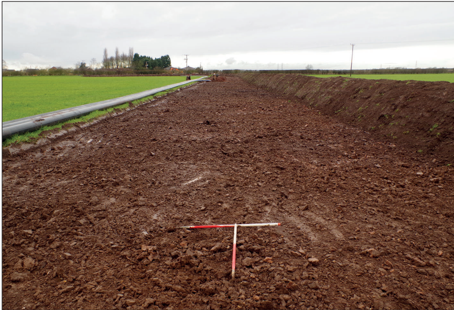
Figure 3: Trench 2, facing east, scales 1 m
