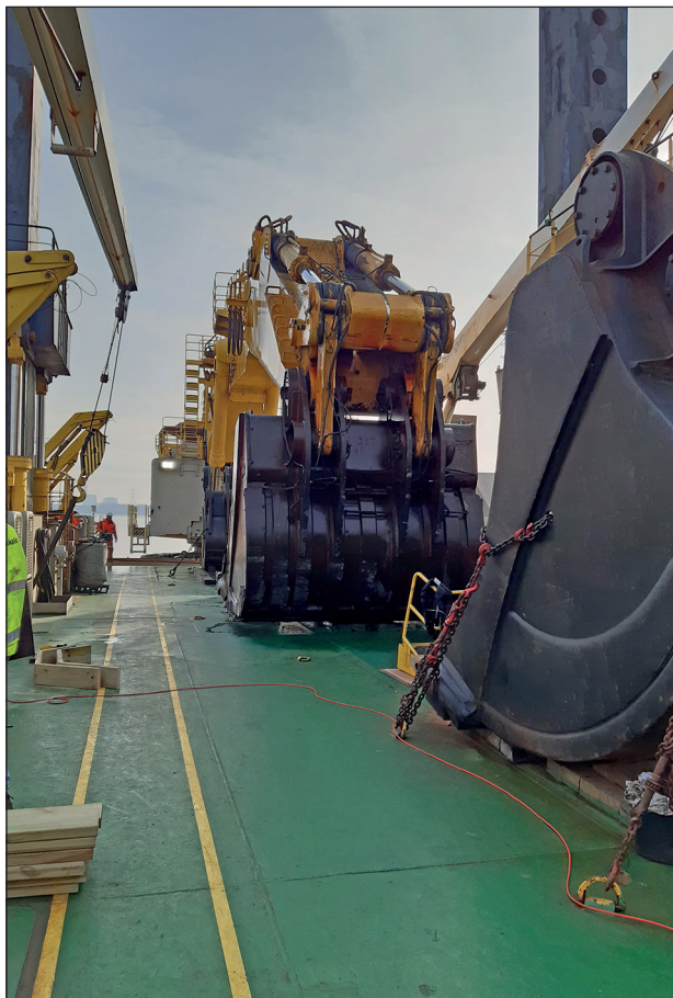
Figure 5: Working shot of the Dredger Odin crane
