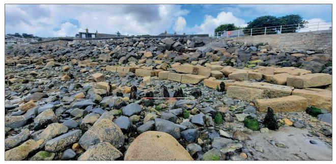
Figure 4: Wooden piles running broadly parallel with and to seaward side of granite kerb stones
