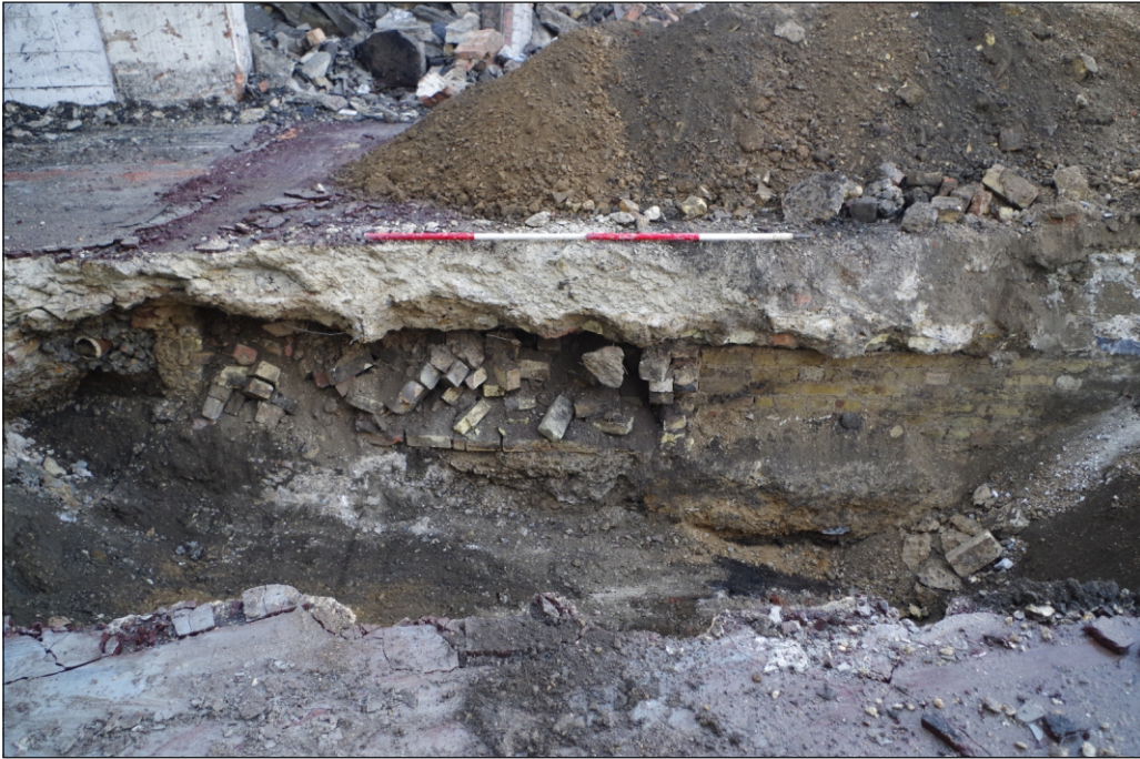
Plate 1: Southeast facing section of Trench 1, showing unstable made ground
