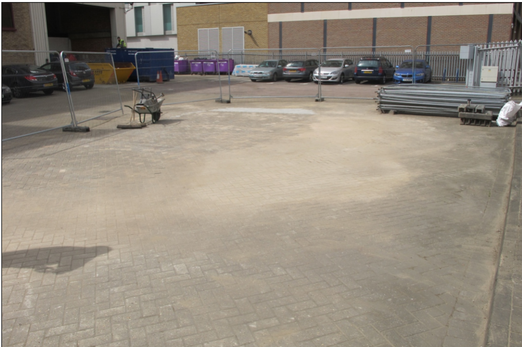
Plate 6: Reinstated car park
