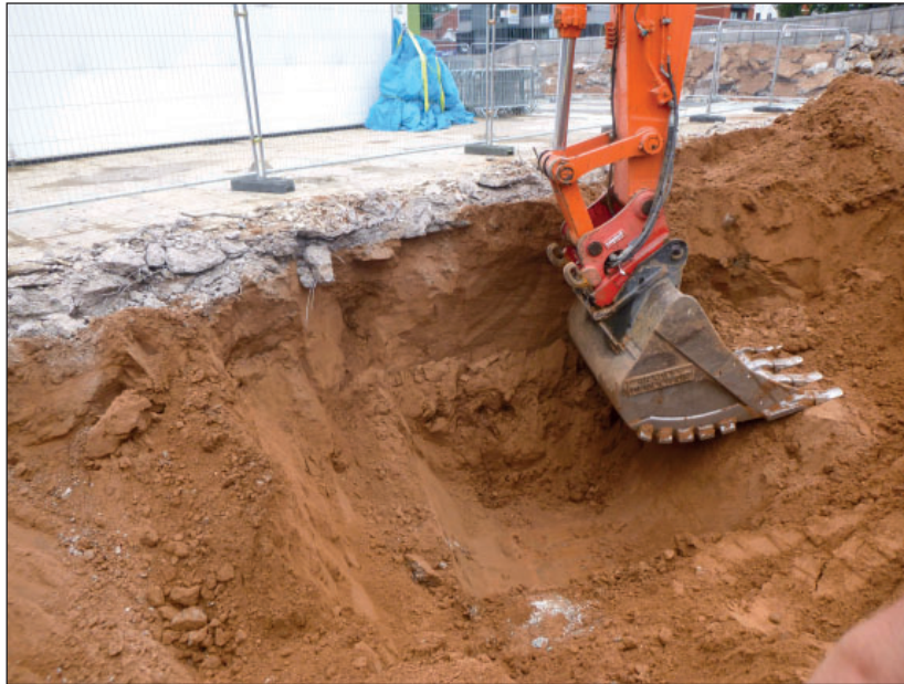
Figure 3: Photograph showing the depth of levelling layer 1005, view from east
