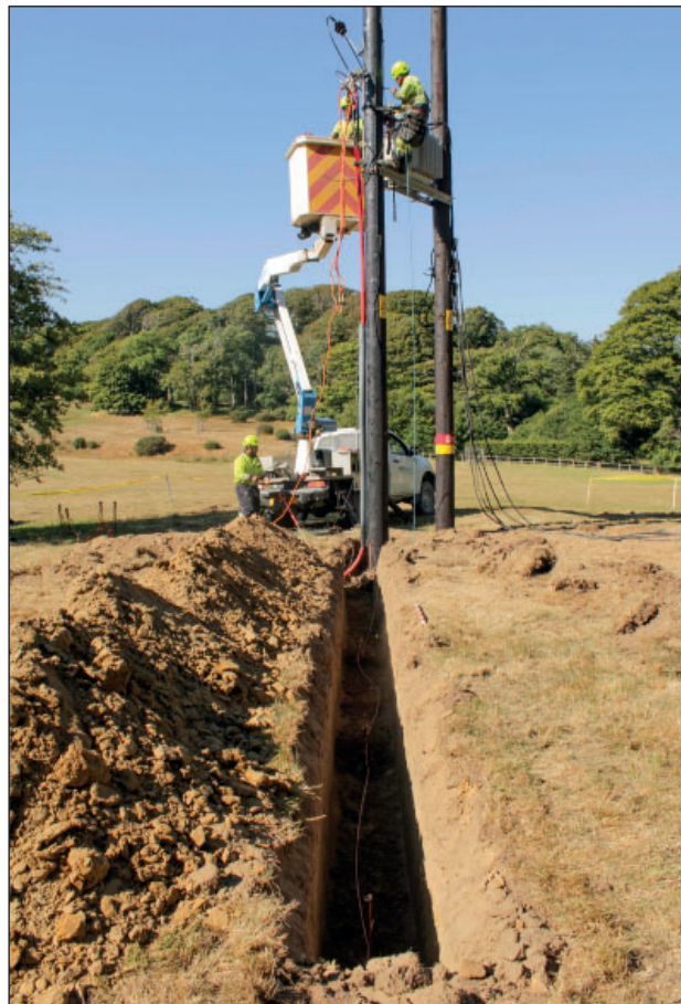
Figure 12: Extension of Trench 3 for earthing cable, view from the south west
