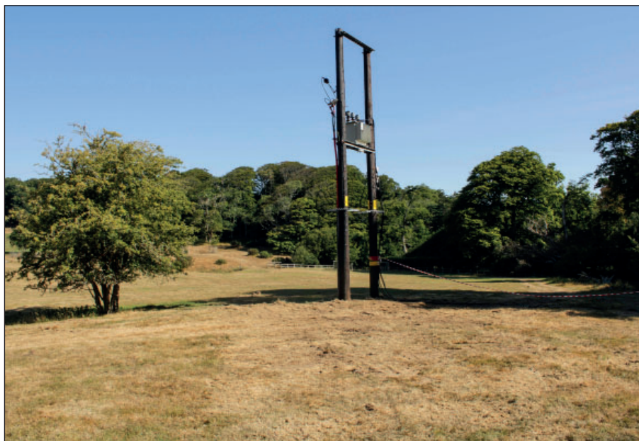
Figure 13: Completed works at Location 2, view from the south
