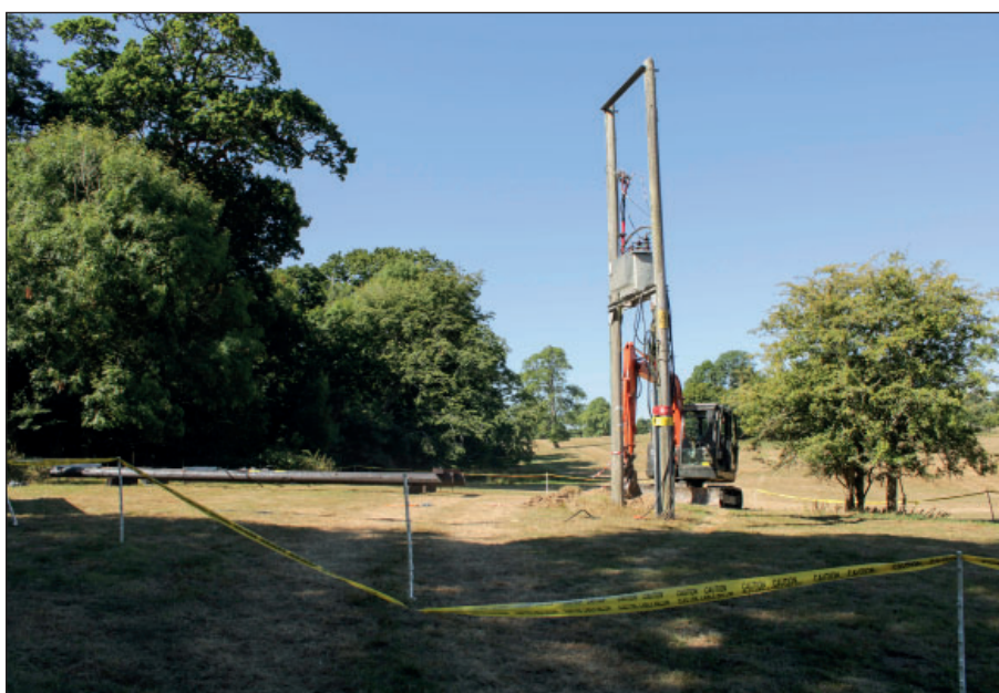
Figure 8: Pre-excavation of Location 2, view from the north-east
