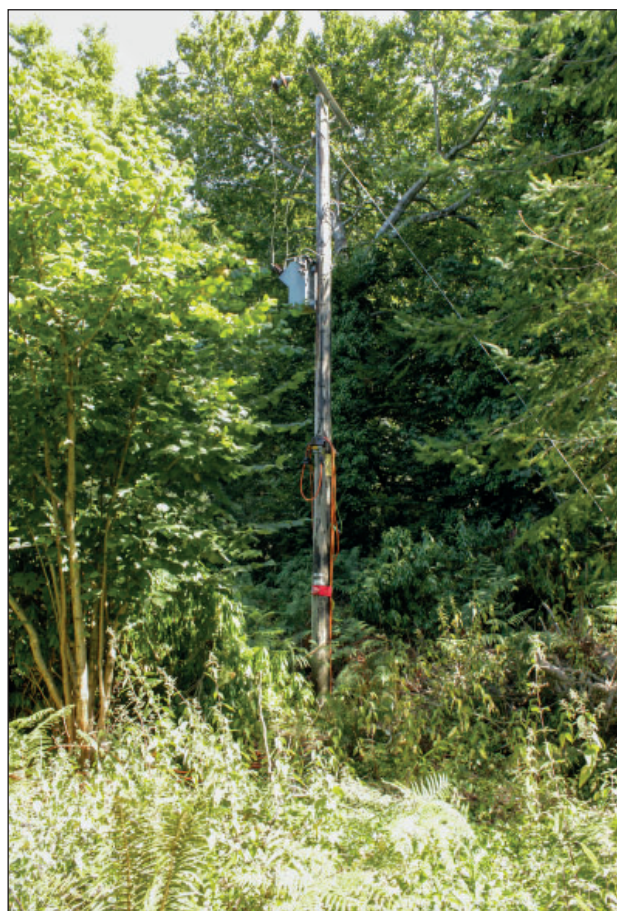
Figure 14: Pre-excavation of Location 3
