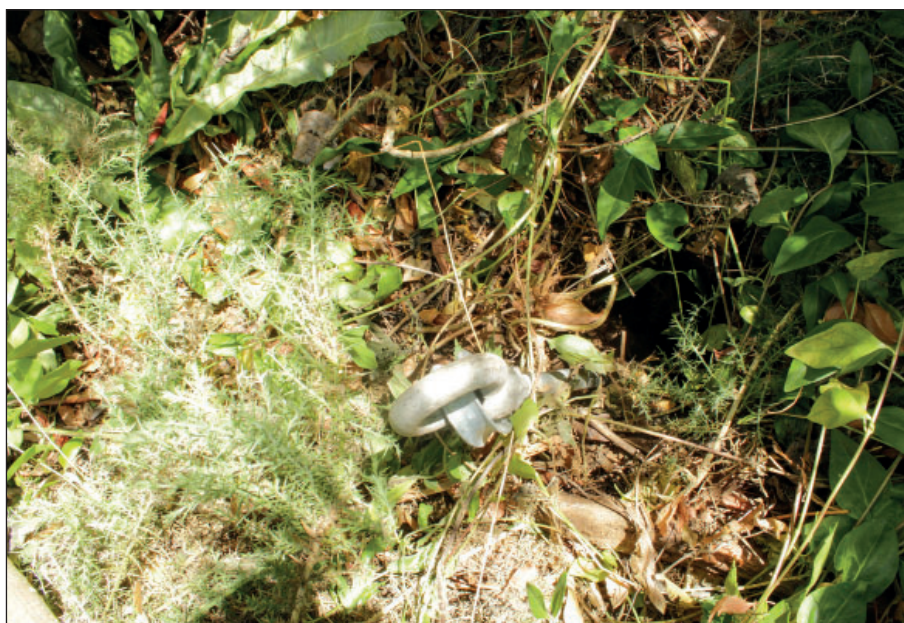
Figure 16: Installed helix screw in stay
