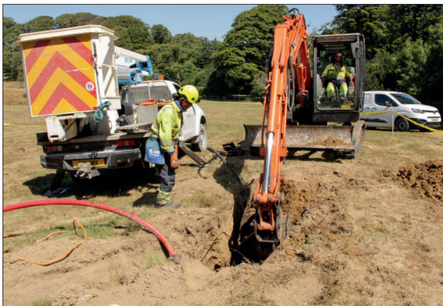
Figure 9: Excavation of Trench 3 at Location 2, view from the north-east
