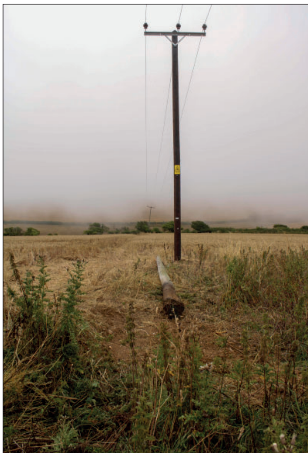
Figure 7: Completed work in Location 1, view from the west
