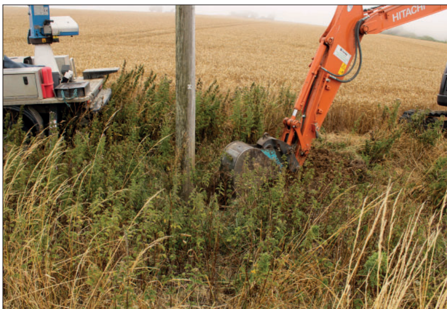
Figure 4: Start of excavation of Trench 1, view from the south-west
