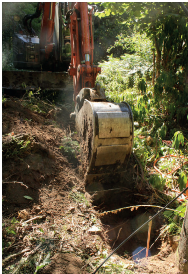
Figure 17: Working shot of Trench 4, view from the north-west
