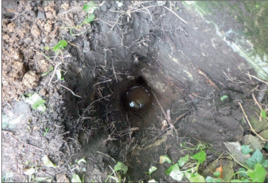
Figure 2: TP1 showing depth of bridge foundations
