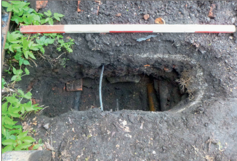
Figure 7: TP9, modern services, view from north, 1 x 1 m scale
