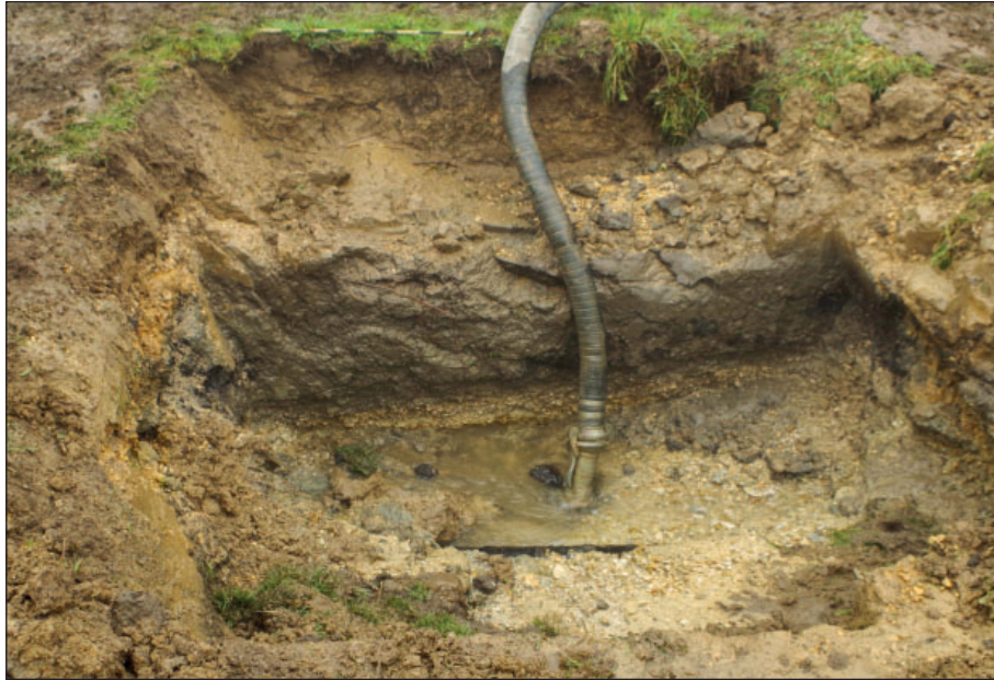
Figure 4: Trial pit 1 from the north, scale: 1 x 1 m
