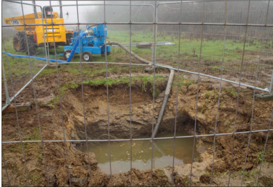
Figure 2: Trial pit 1 from the north
