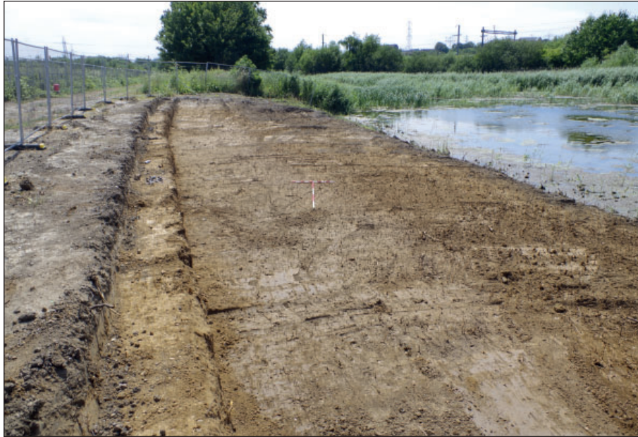
Figure 3: Initial strip for southern cofferdam, viewed from the north, 1 m and 2 m scales. (Photograph taken by Lisa McCaig)
