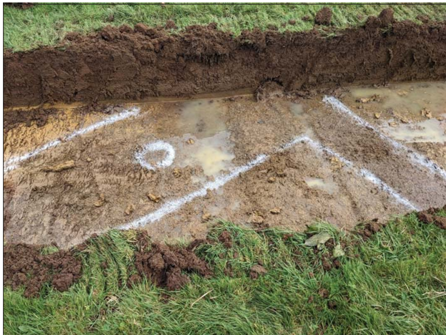
Figure 12: Ditches 2204 and 2206 prior to water ingress. View looking east
