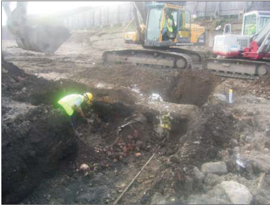
Plate 1: Excavation of Building N area, east facing
