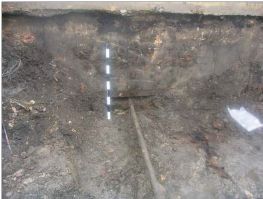
Plate 4: Exposed river wall with tie-rod, from east, 1m scale
