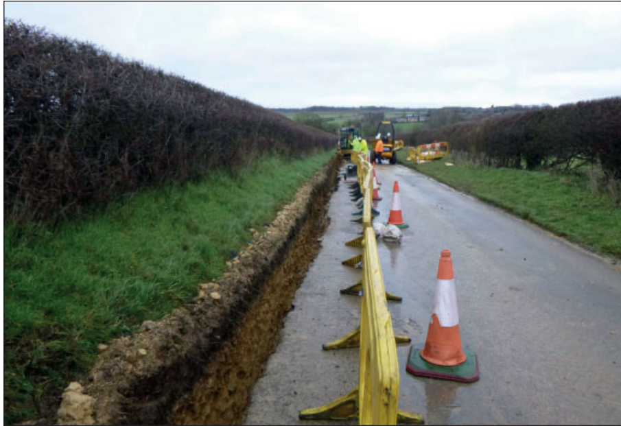
Figure 5: Trench 303 from the south
