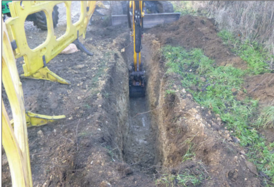
Figure 6: Excavation of trench 306 from the north-east
