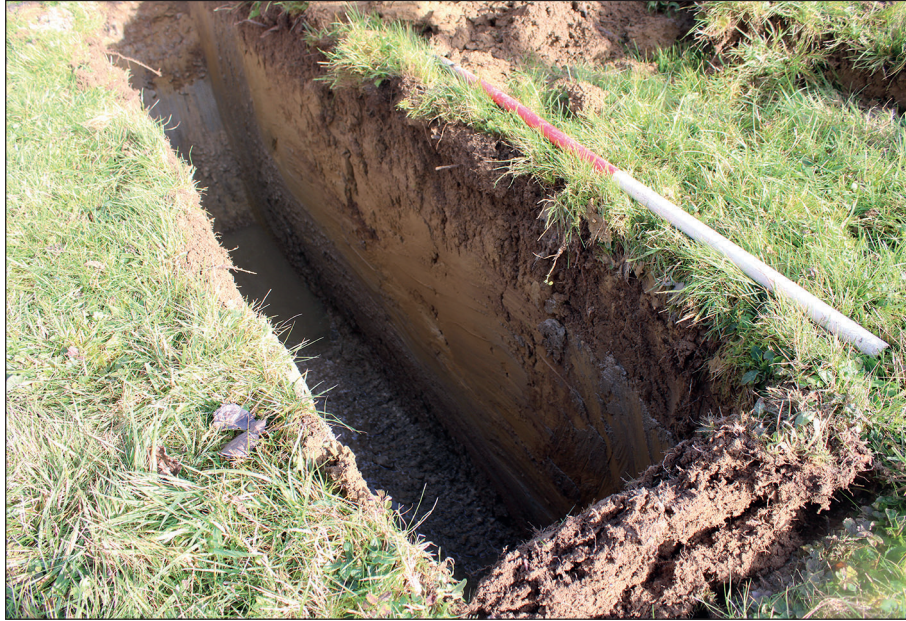
Figure 5: Trial Pit 7, looking northeast, 1 m scale
