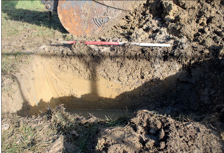
Figure 4: Trial Pit 6, looking northwest, 1 m scale
