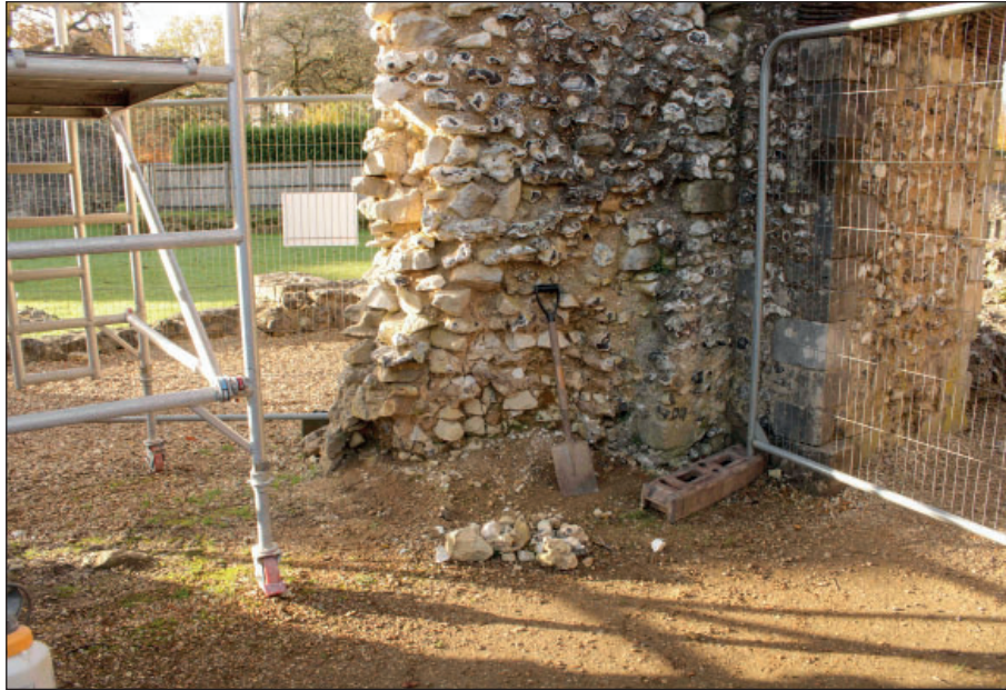
Figure 2: Pre-excitation shot of Trench 1 location, view from NE
