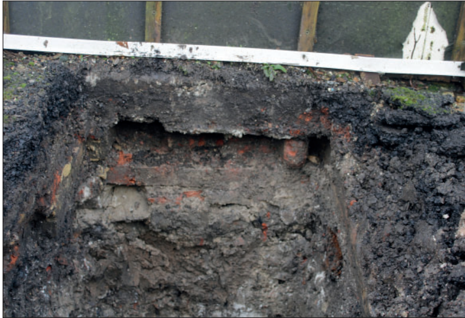
Figure 8: North facing section of Test Pit 3 showing modern foundations
