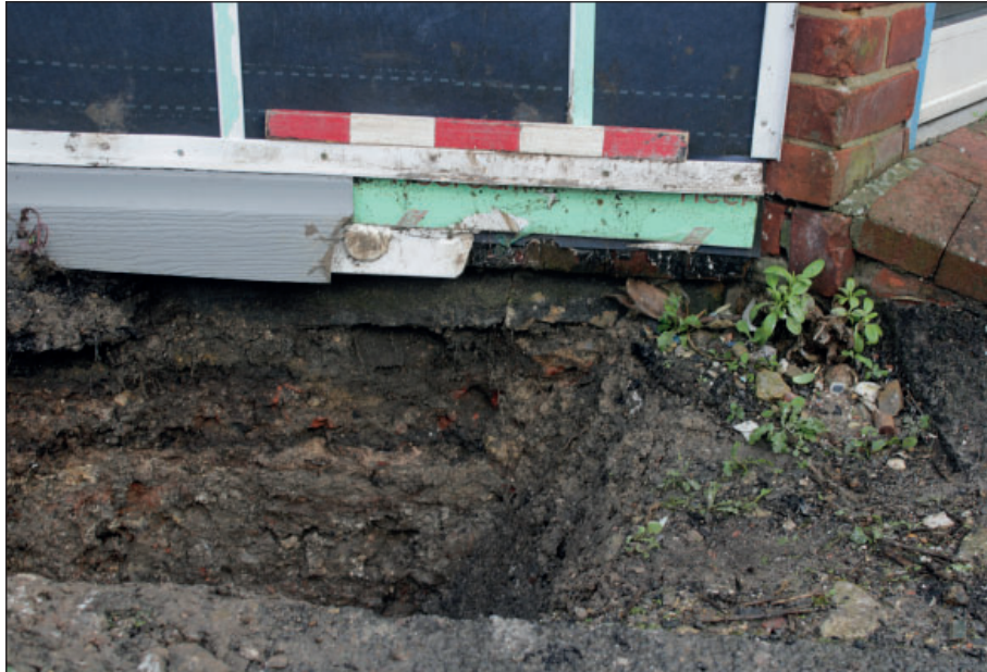
Figure 5: South facing section of Test Pit 2 showing modern foundations (1 x 0.50 m)
