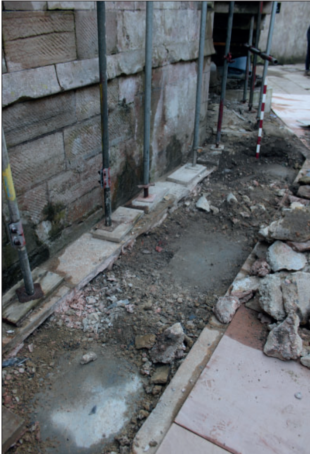
Figure 3. Trench 1 looking west, 1m scale
