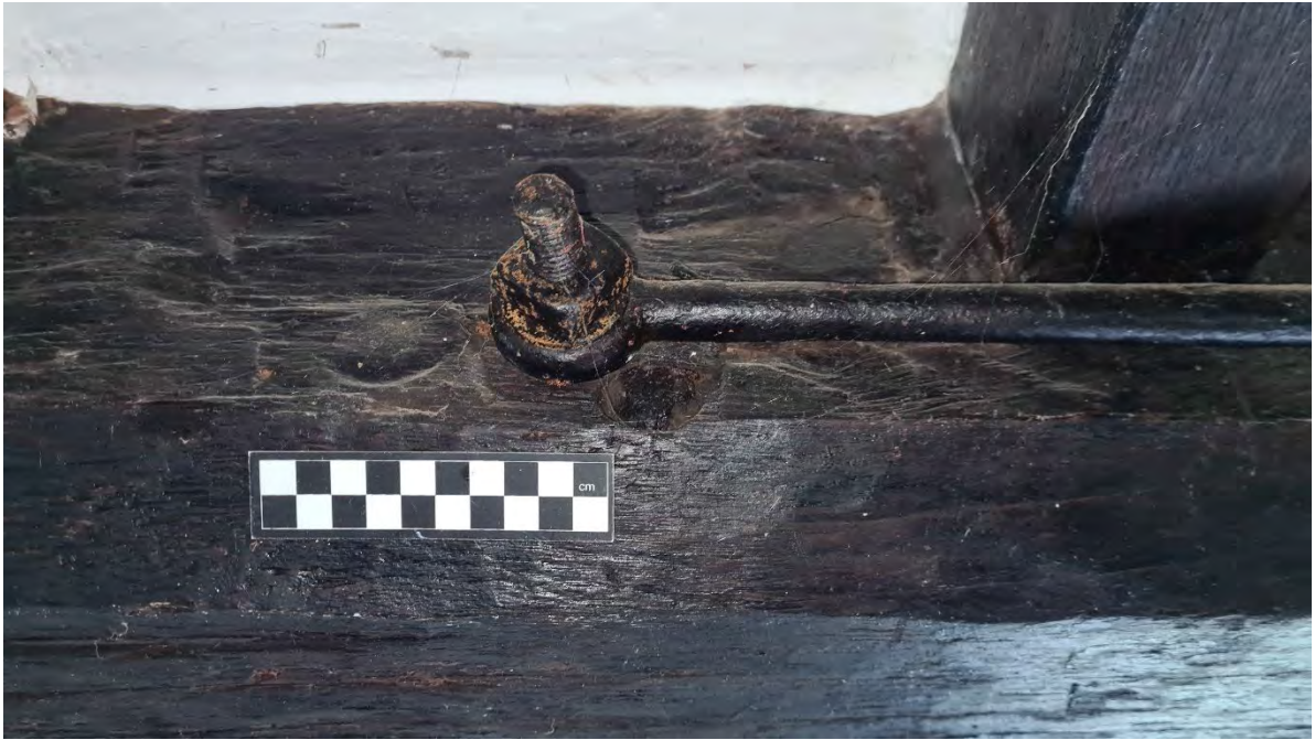
Plate 79 - Steel brace on timber beam in Room G7
