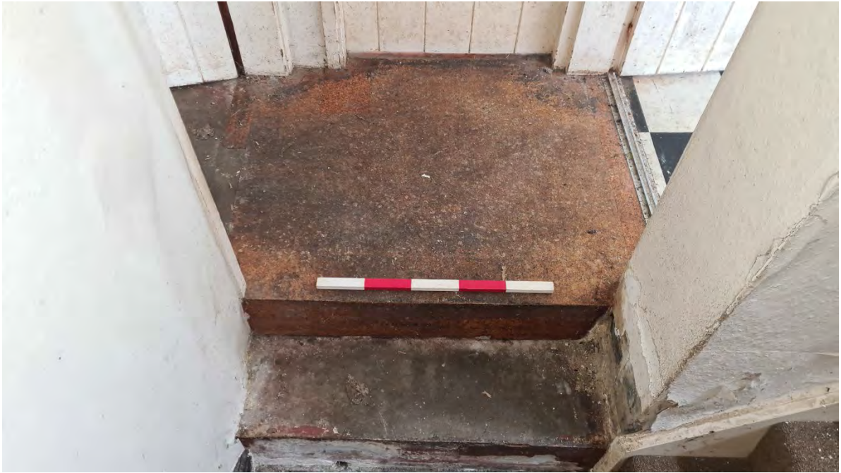
Plate 47 - Detail shot of foot of staircase
