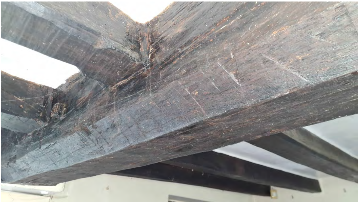
Plate 76 - East facing shot of timber beams in Room G7
