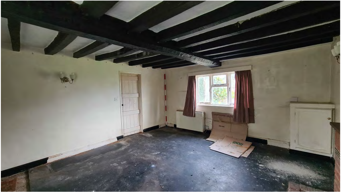
Plate 67 - Southwest facing shot of Room G7
