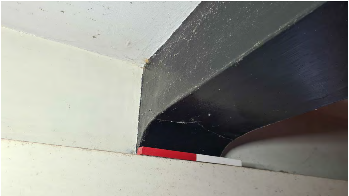
Plate 61 - East facing shot of timber beam in Room G6
