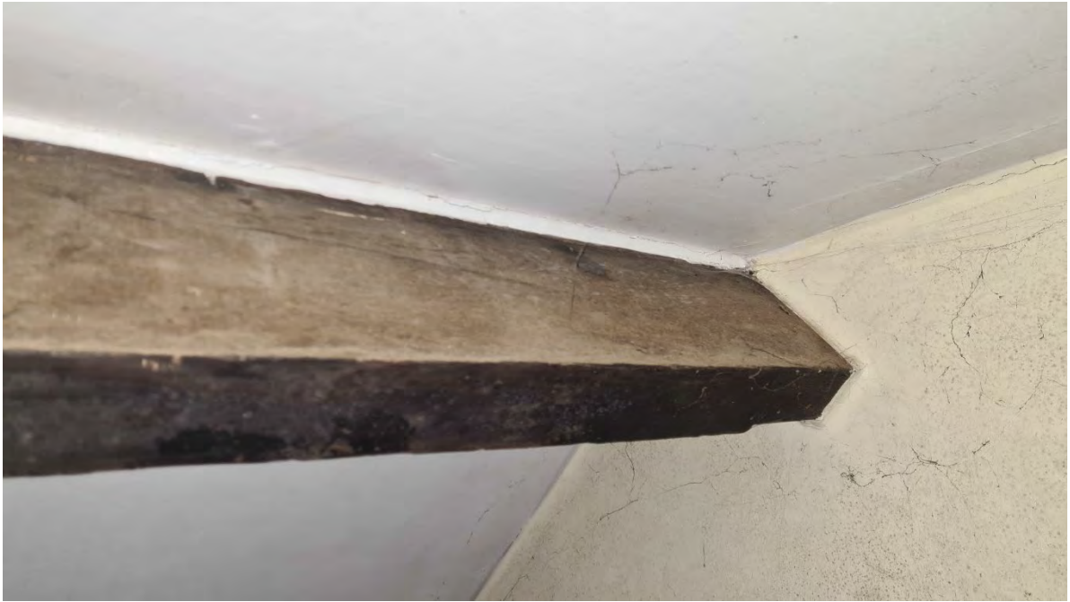
Plate 89 - Northeast facing photo of timber beam in Room G9
