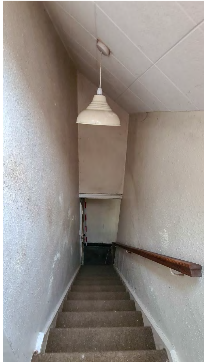
Plate 48 - South facing shot of staircase
