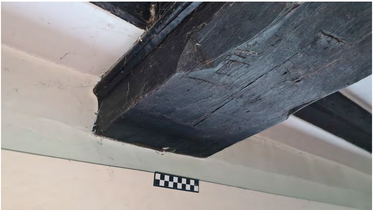
Plate 78 - West facing photo of restoration of timber beam in Room G7
