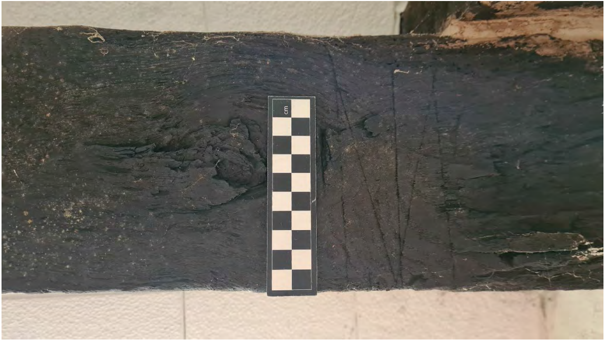
Plate 51 - Detail shot of timber beam on landing area
