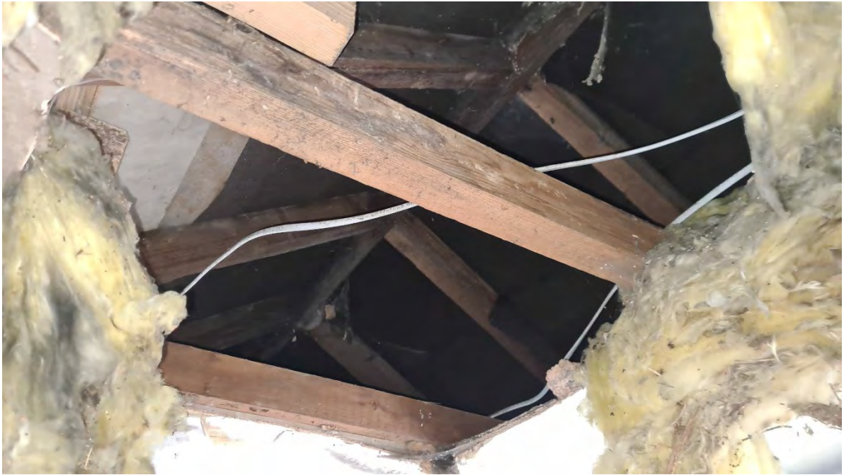
Plate 87 - Exposed timber framed roof in Room G9
