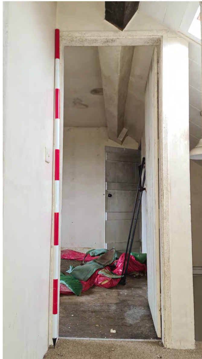
Plate 80 - South facing shot of G8 threshold
