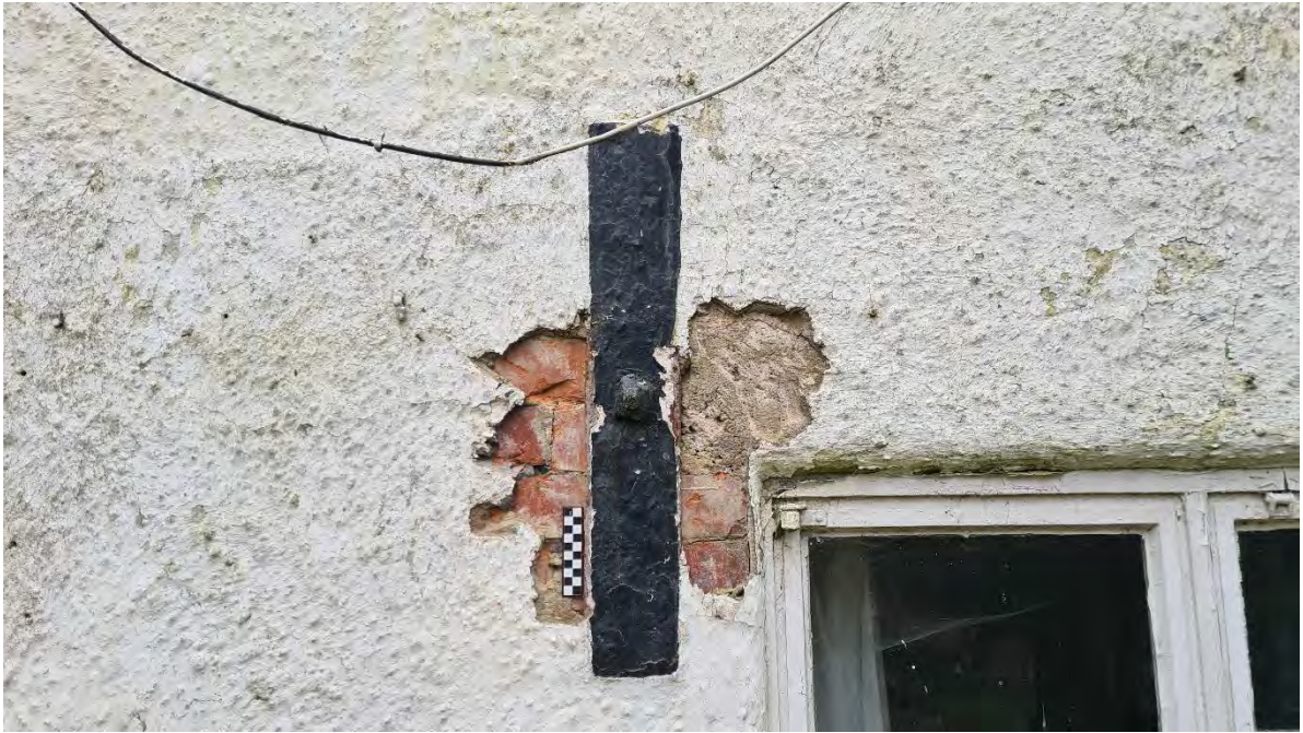
Plate 15 - Anchor plate south of north most ground floor window east elevation
