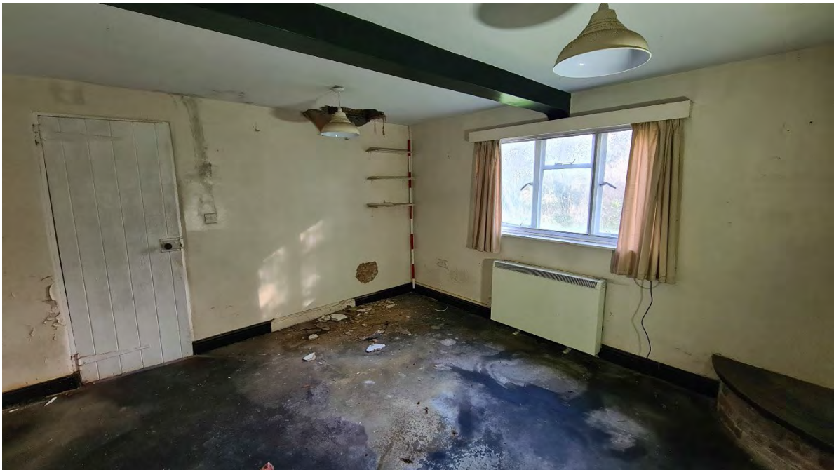
Plate 59 - Northeast facing shot of Room G6
