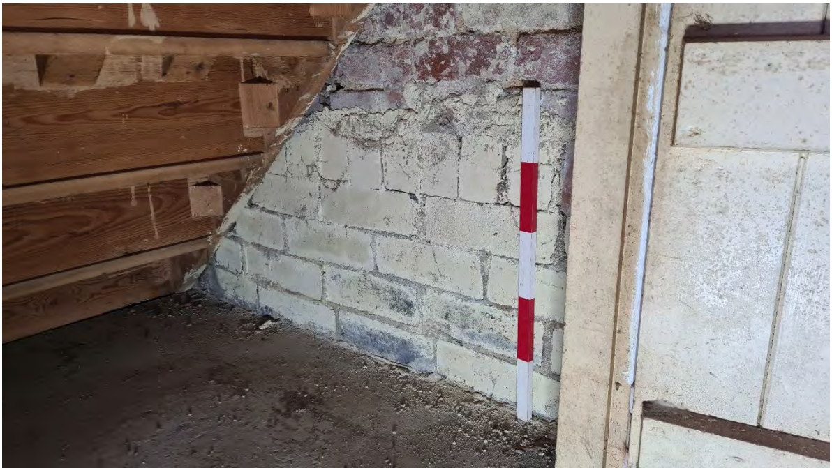
Plate 66 - Cupboard below staircase in Room G6
