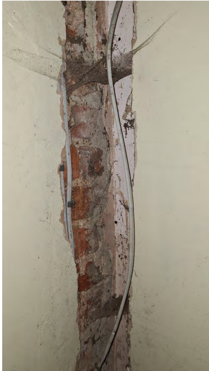
Plate 90 - Southwest shot of exposed plaster in Room G9
