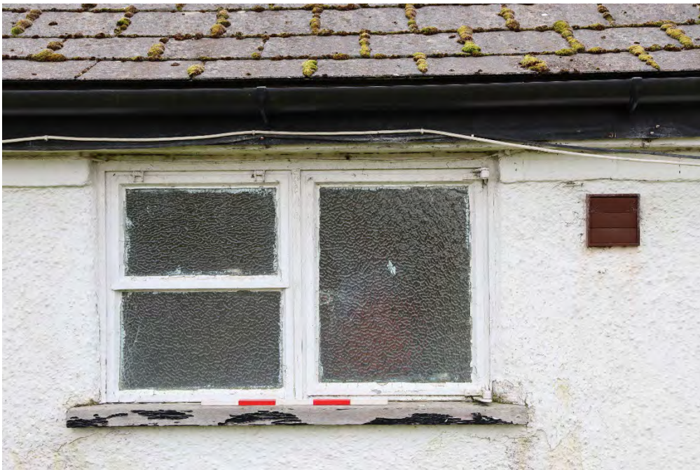
Plate 24 - South most ground floor window west elevation
