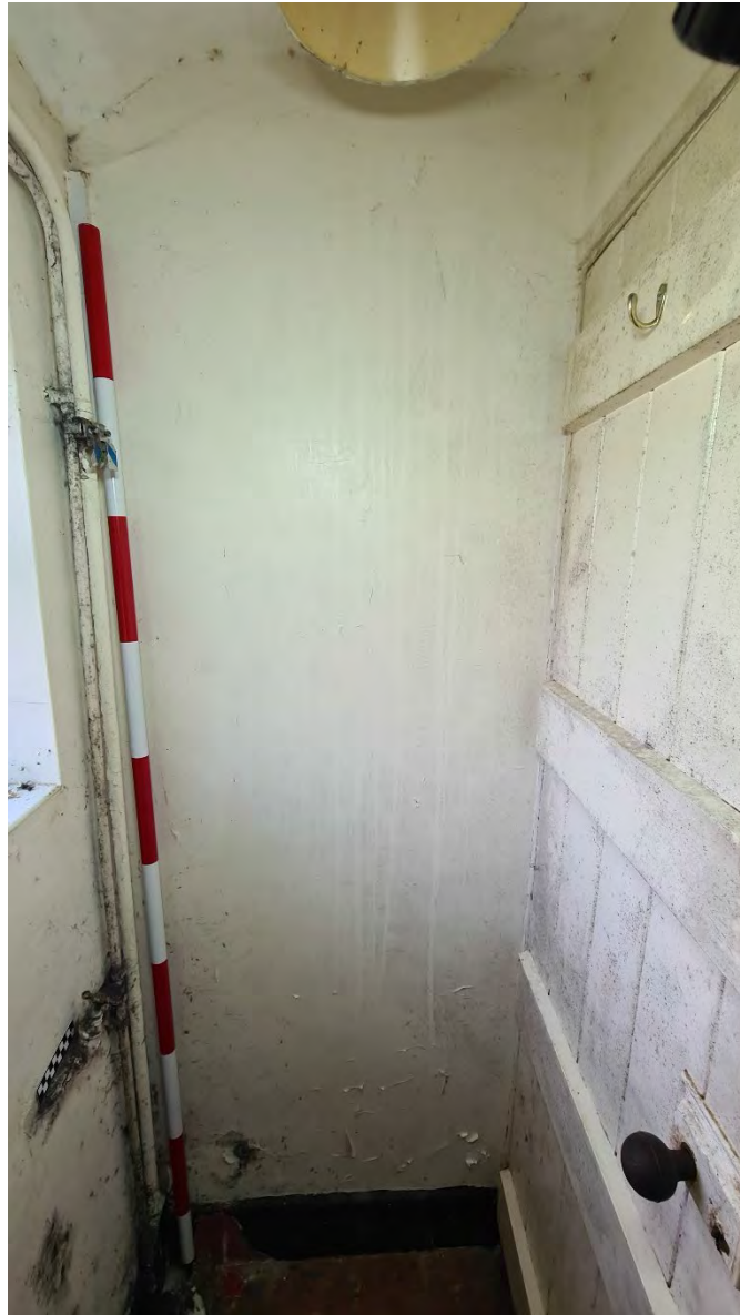
Plate 37 - North facing shot of Room G3
