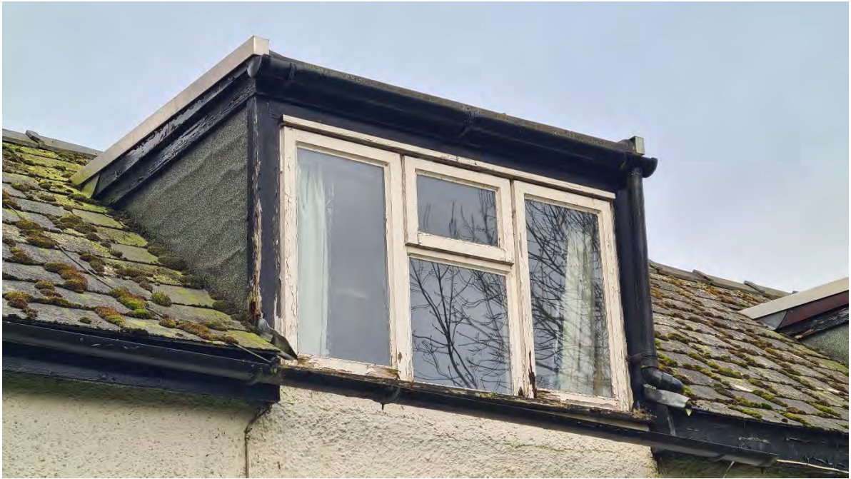
Plate 11 - East elevation first floor dormer window
