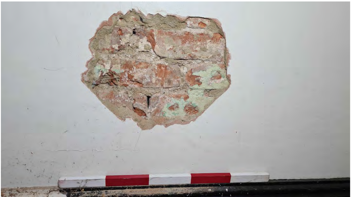
Plate 58 - Exposed brick fabric in Room G6
