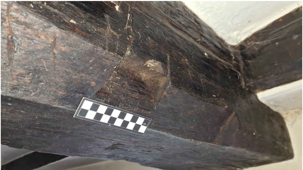
Plate 73 - Southwest facing photo of timber and timber peg fitting beam in Room G7
