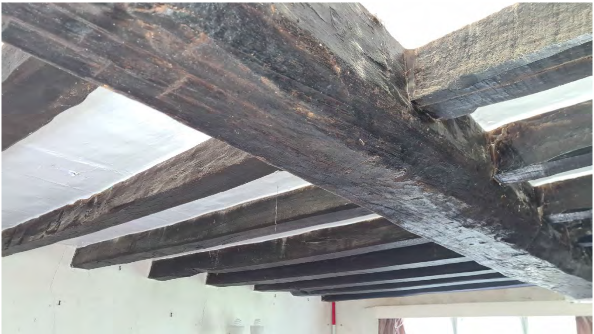
Plate 70 - Northeast facing photo of timber beams in Room G7
