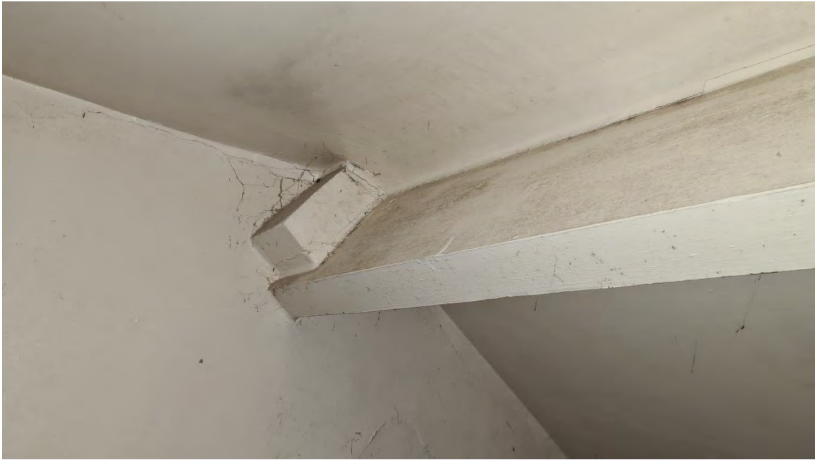
Plate 83 - Northwest facing photo of timber beam in Room G8
