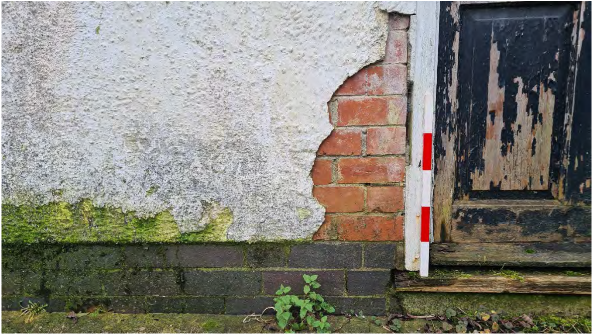
Plate 14 - East elevation central threshold into G7 exposed fabric
