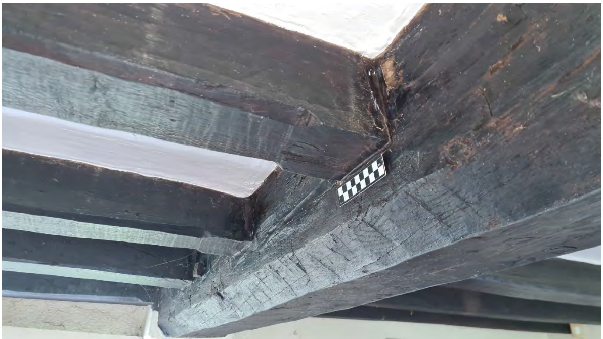
Plate 74 - East facing photo of timber beams in Room G7
