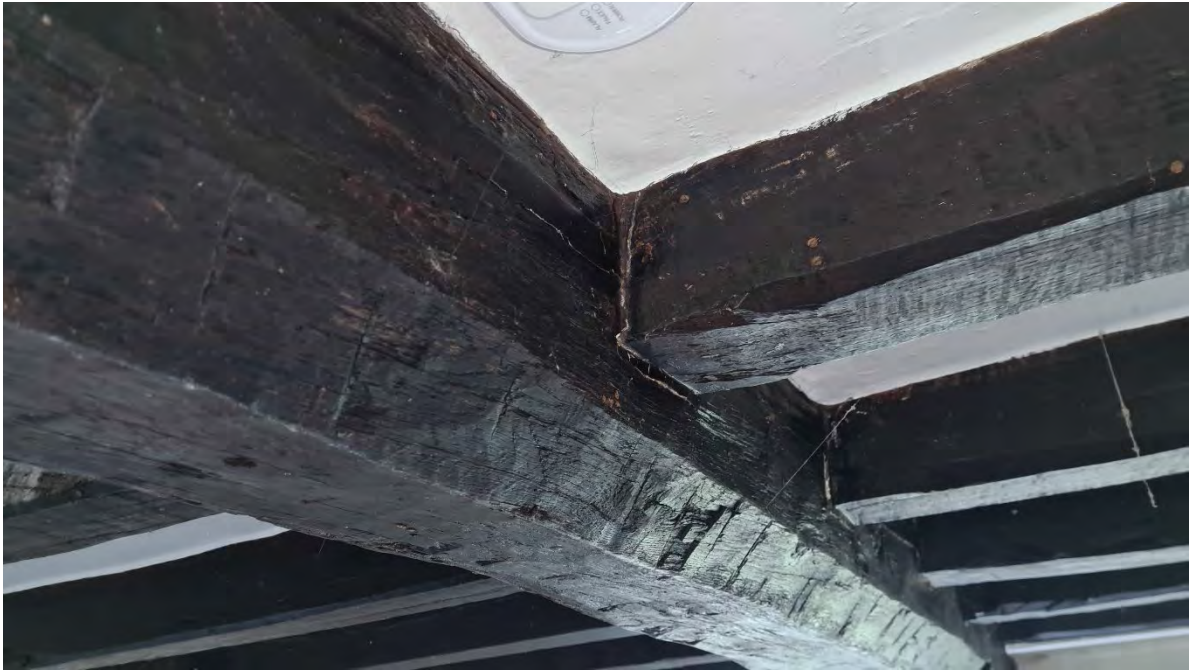
Plate 75 - Southwest facing shot of timber beams in Room G7
