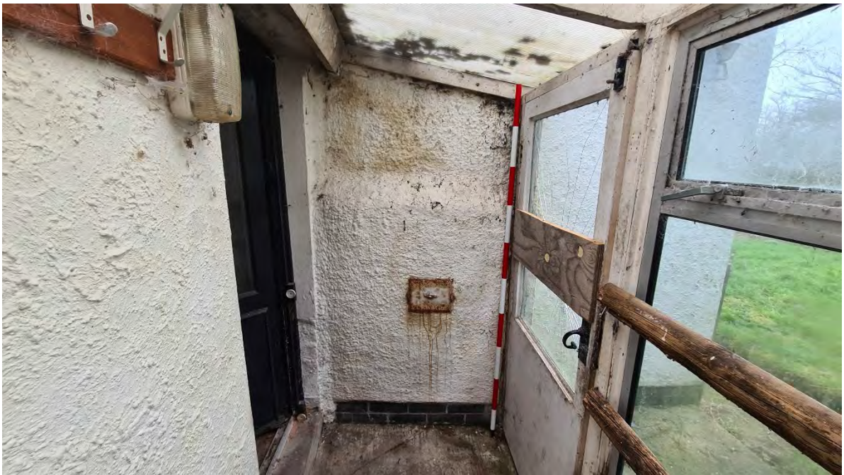
Plate 30 - Porch area Room G1 north facing
