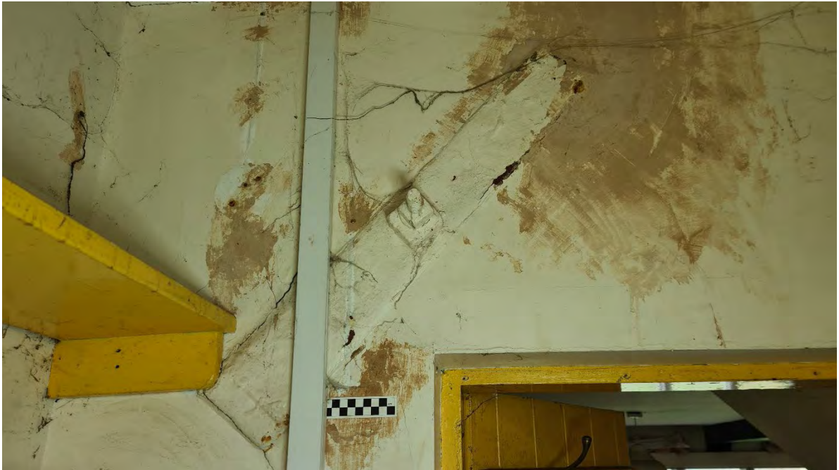
Plate 55 - Anchor plate fixed to east elevation wall in Room G5
