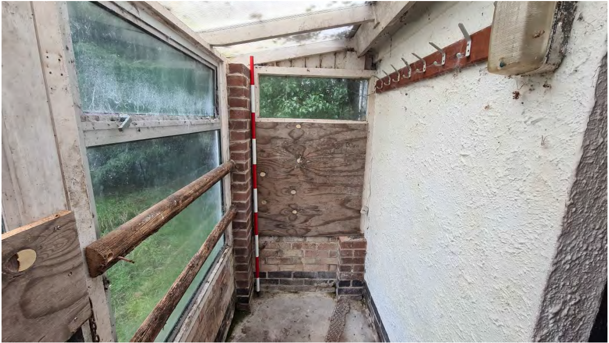
Plate 29 - Porch area Room G1 south facing
