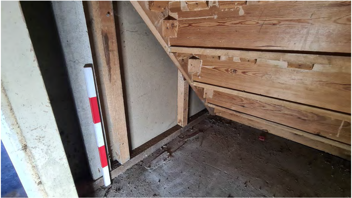
Plate 65 - Cupboard below staircase in Room G6
