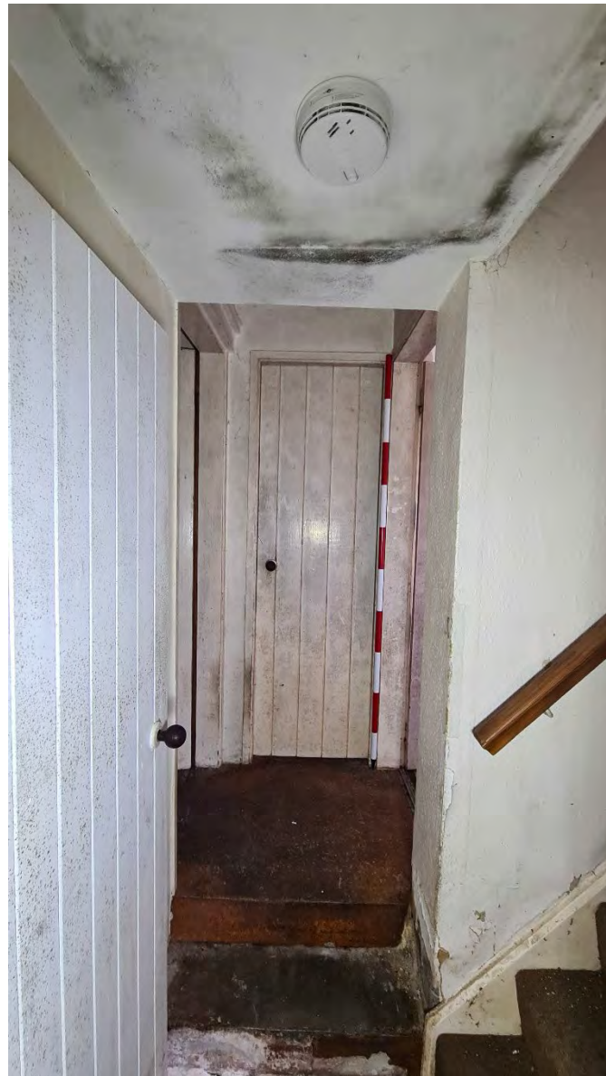
Plate 46 - West facing shot of foot of staircase
