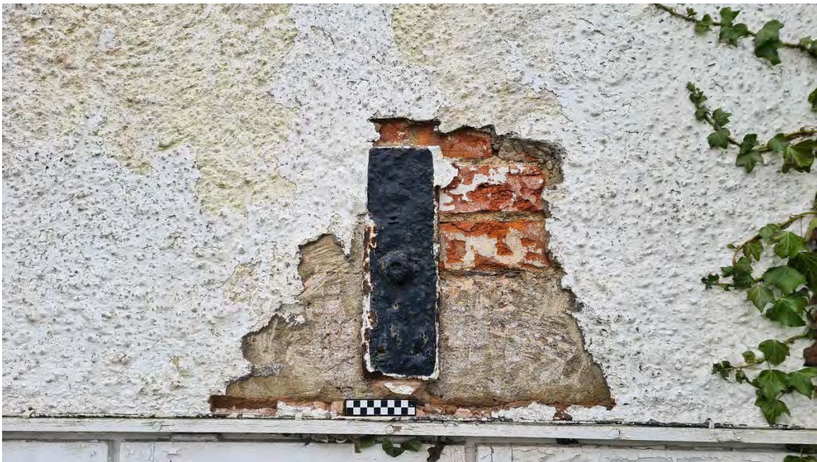
Plate 26 - Anchor plate above north most ground floor window west elevation
