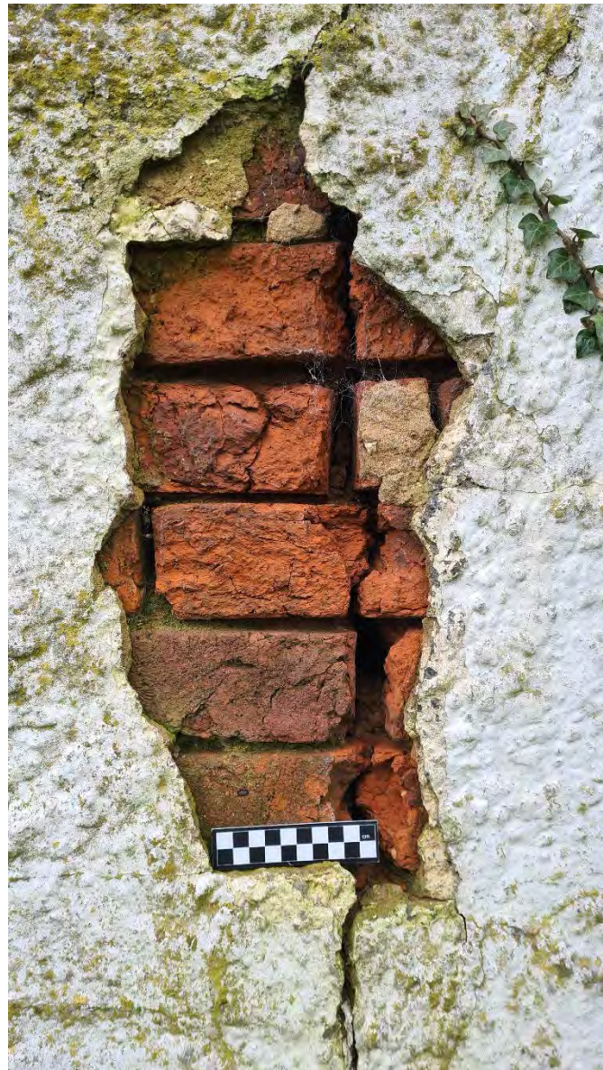
Plate 8 - Exposed brick fabric north chimney
