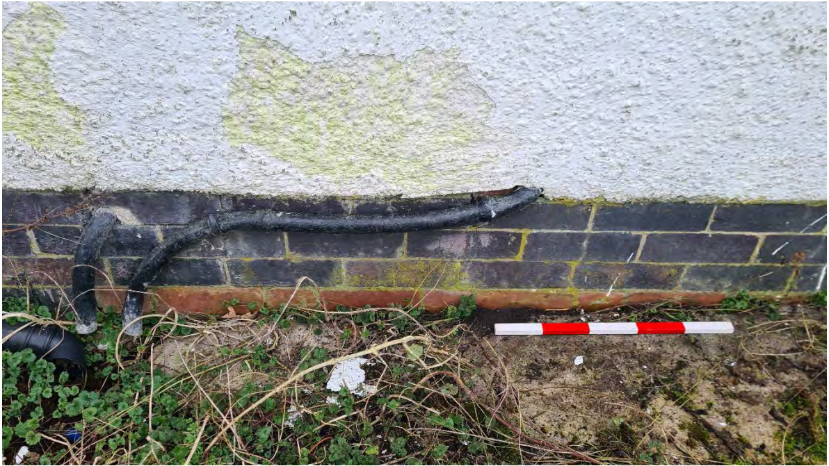
Plate 27 - Staffordshire blue brick footing west elevation
