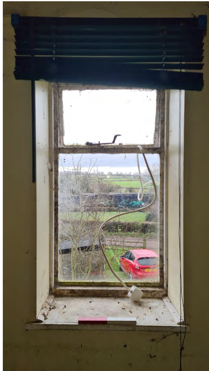
Plate 91 - South facing shot of casement window in Room G9
