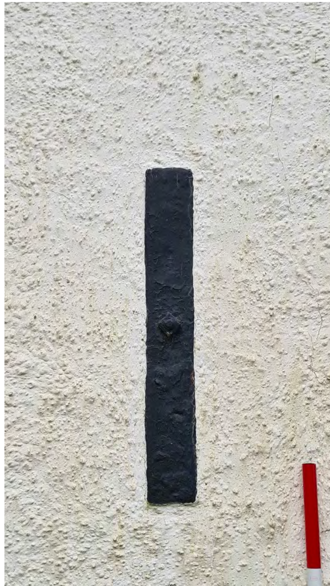
Plate 16 - Anchor plate south of threshold east elevation
