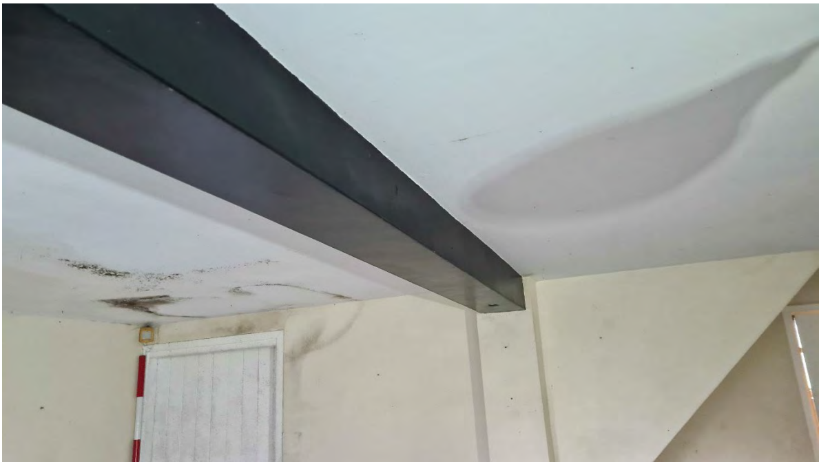
Plate 60 - West facing shot of timber beam in Room G6
