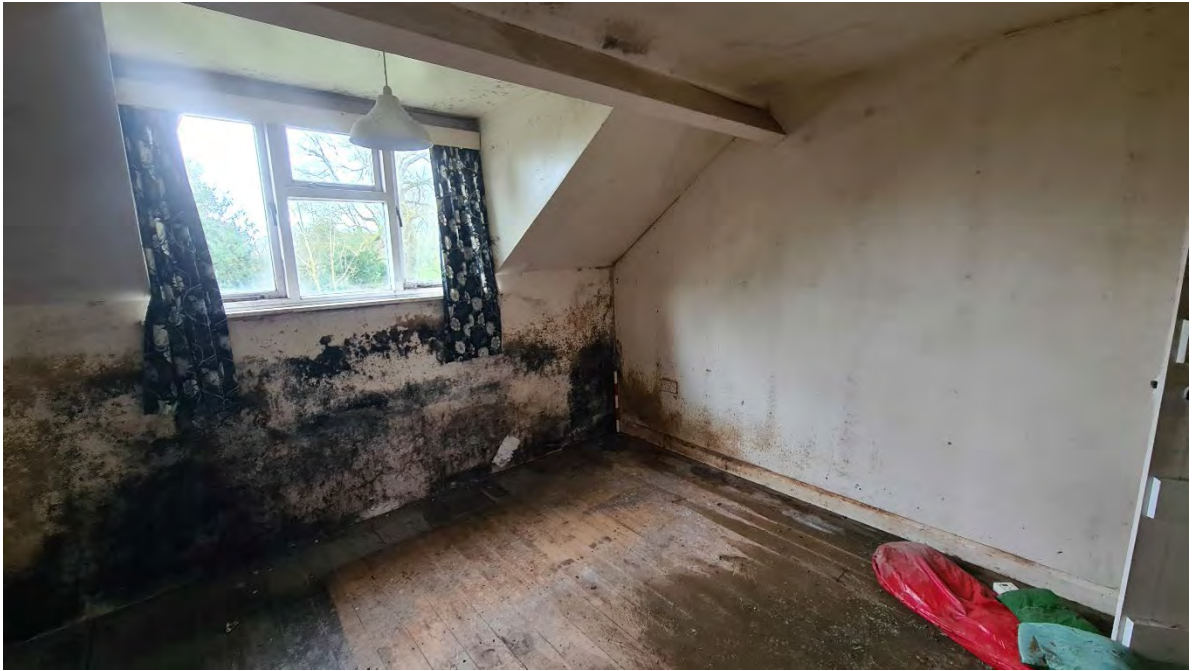
Plate 81 - Southeast facing photo of Room G8
