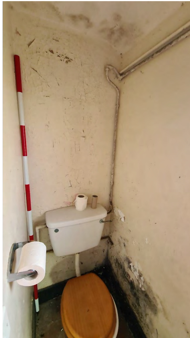
Plate 36 - Southwest shot of Room G3
