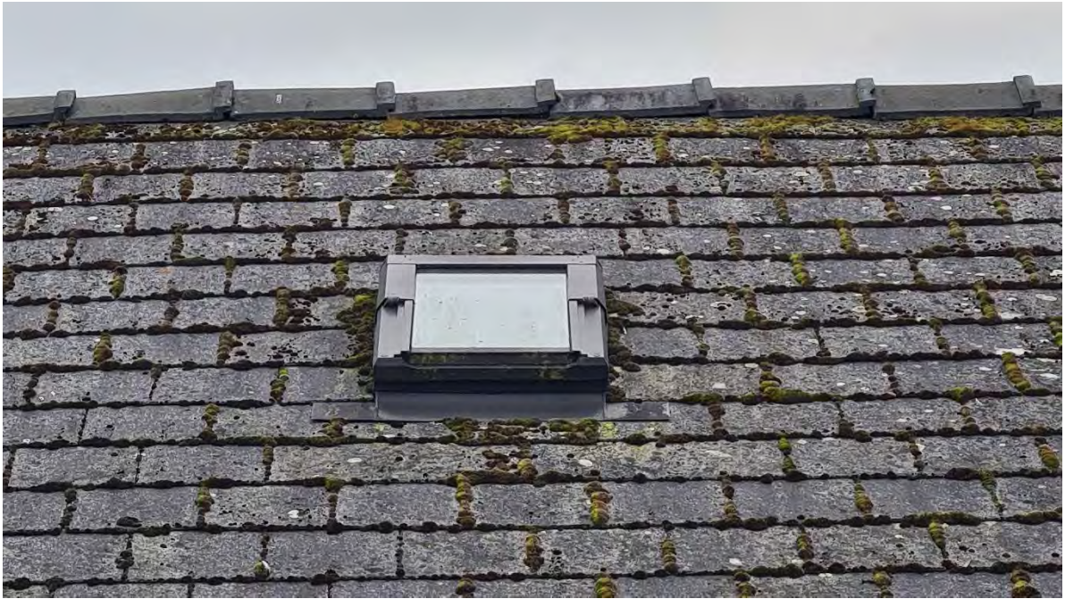
Plate 23 - West elevation skylight
