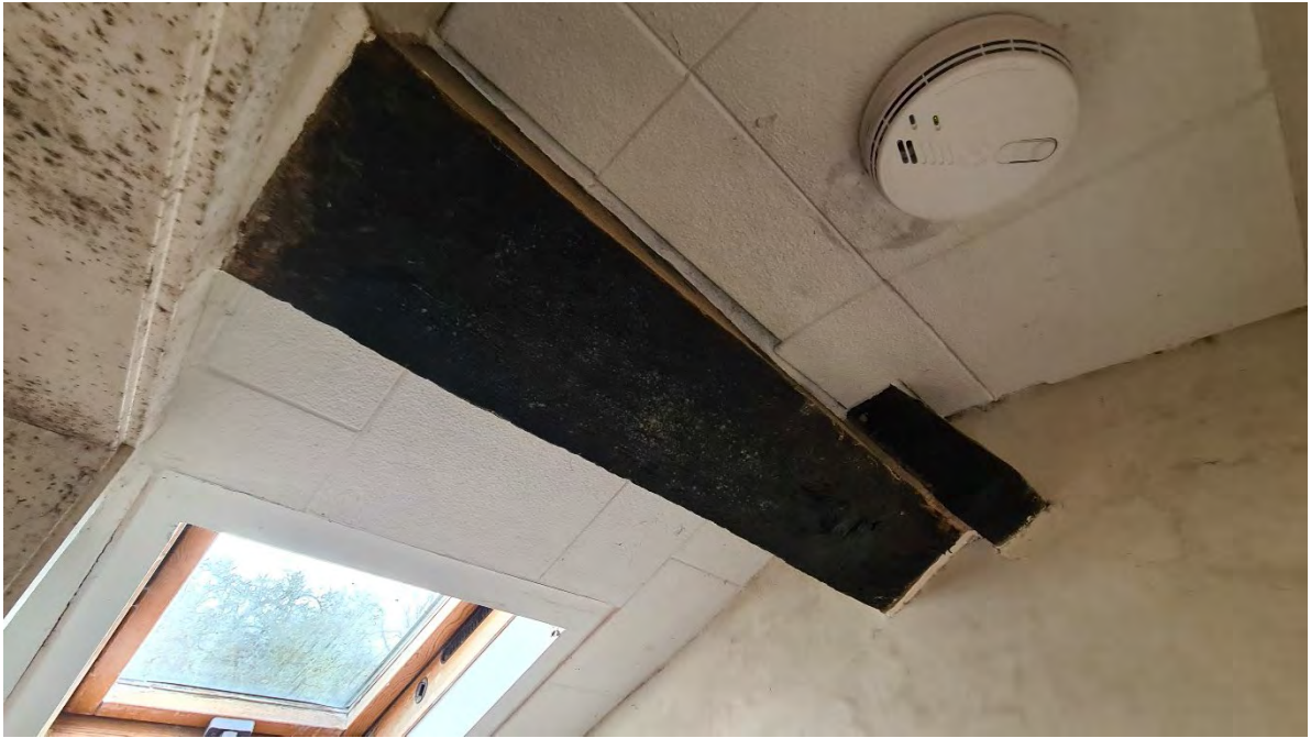
Plate 50 - Timber beam on landing area
