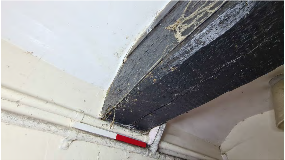
Plate 39 - Detail of timber beam in Room G3
