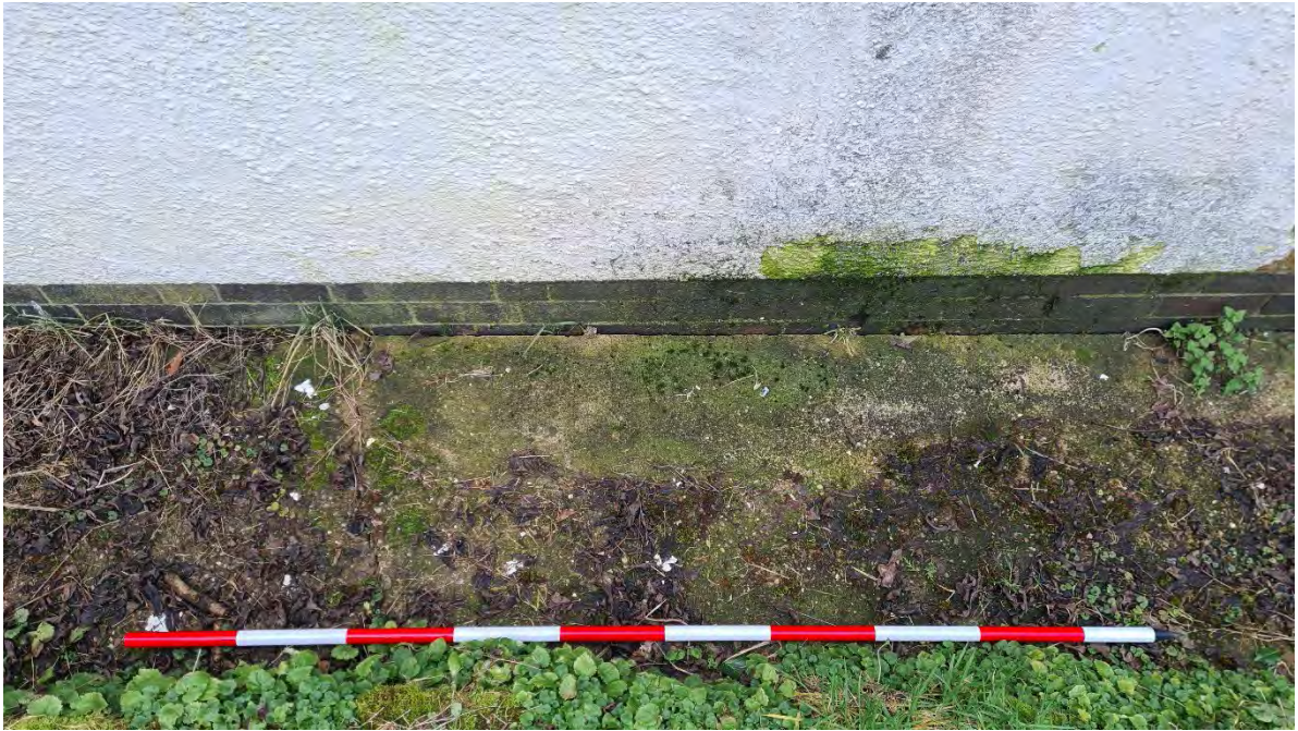
Plate 17 - Concrete footpath east elevation
