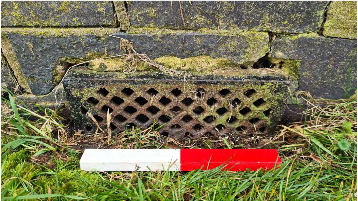
Plate 9 - Cast iron air vent at foot of north chimney
