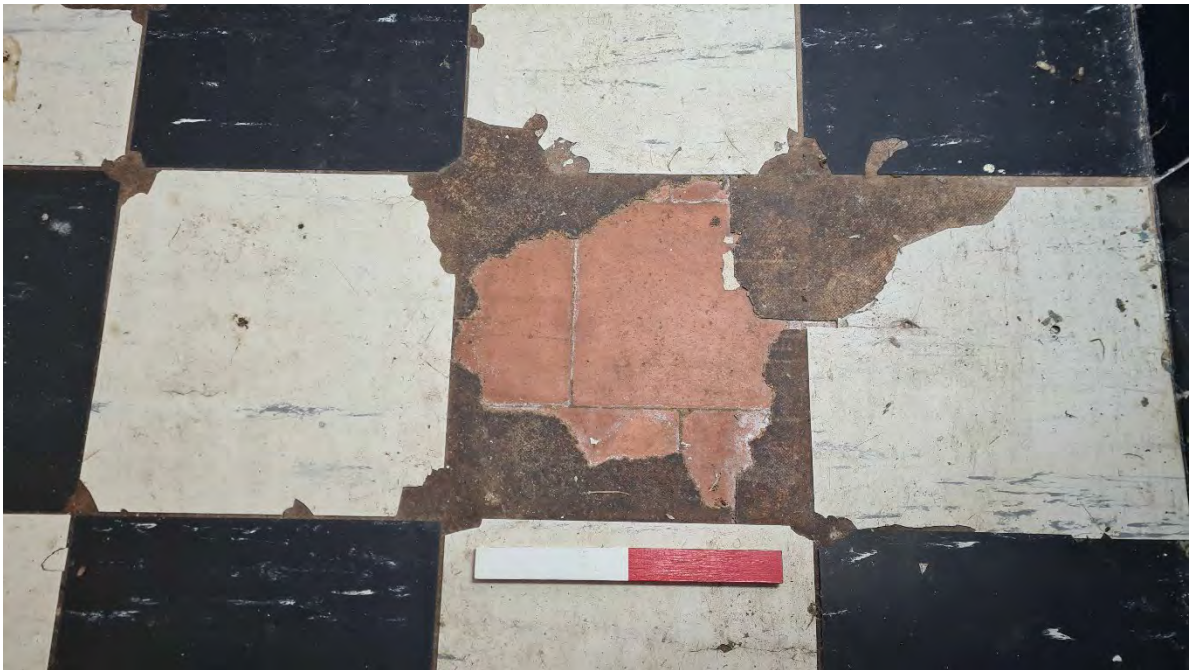
Plate 45 - Tile and Linoleum floor in Room G4
