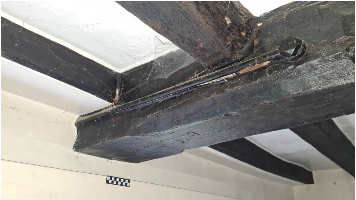
Plate 71 - Northwest facing photo of timber beams in Room G7
