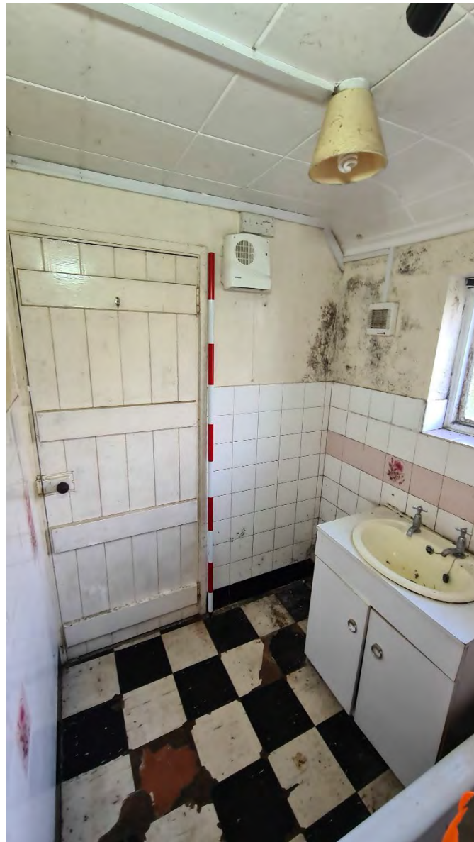
Plate 43 - Southwest facing shot of Room G4
