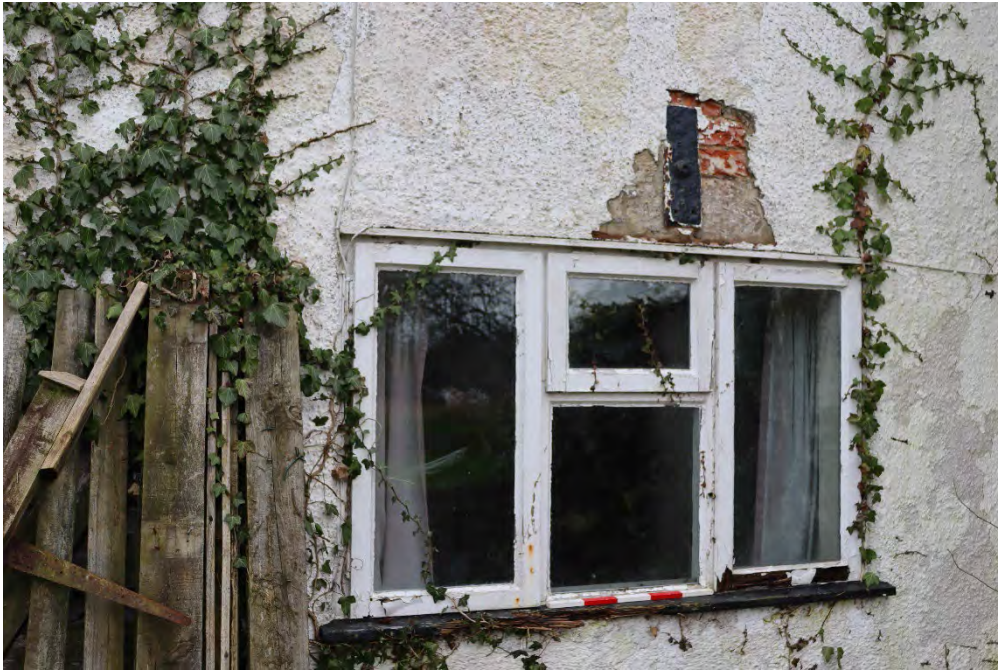
Plate 25 - North most ground floor window west elevation
