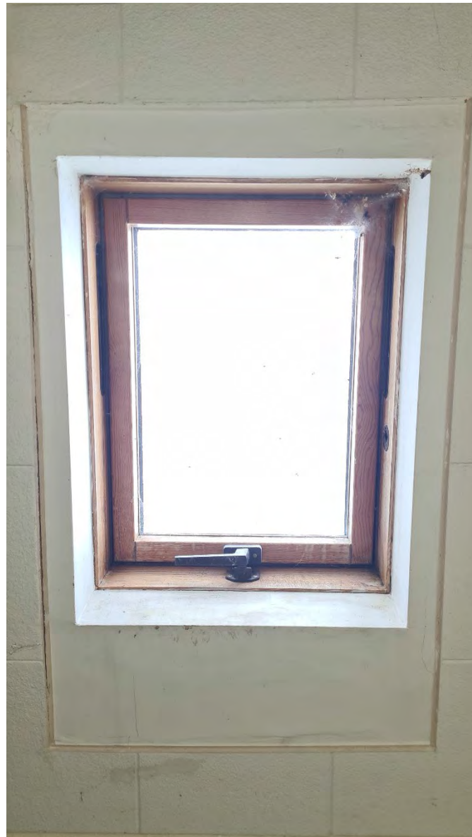
Plate 49 - West facing shot of skylight on landing
