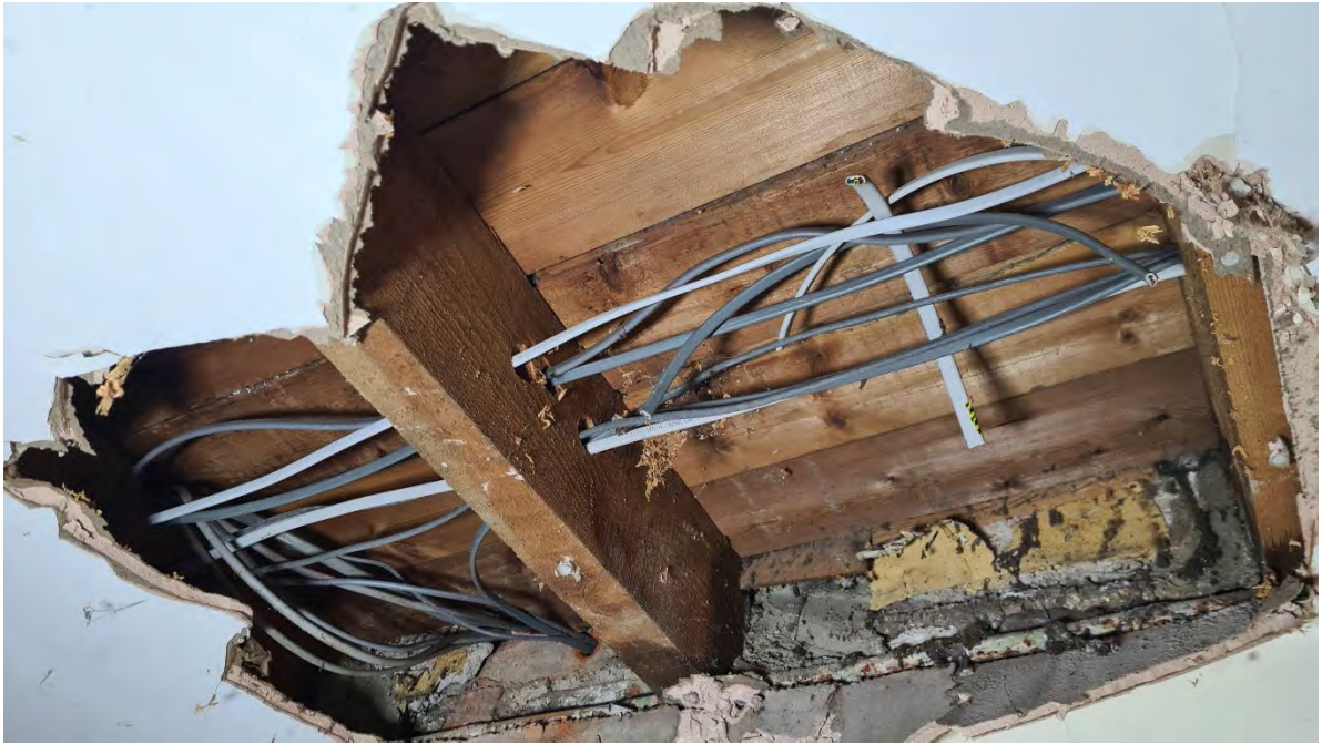
Plate 57 - Exposed ceiling and structural timber beams in Room G6
