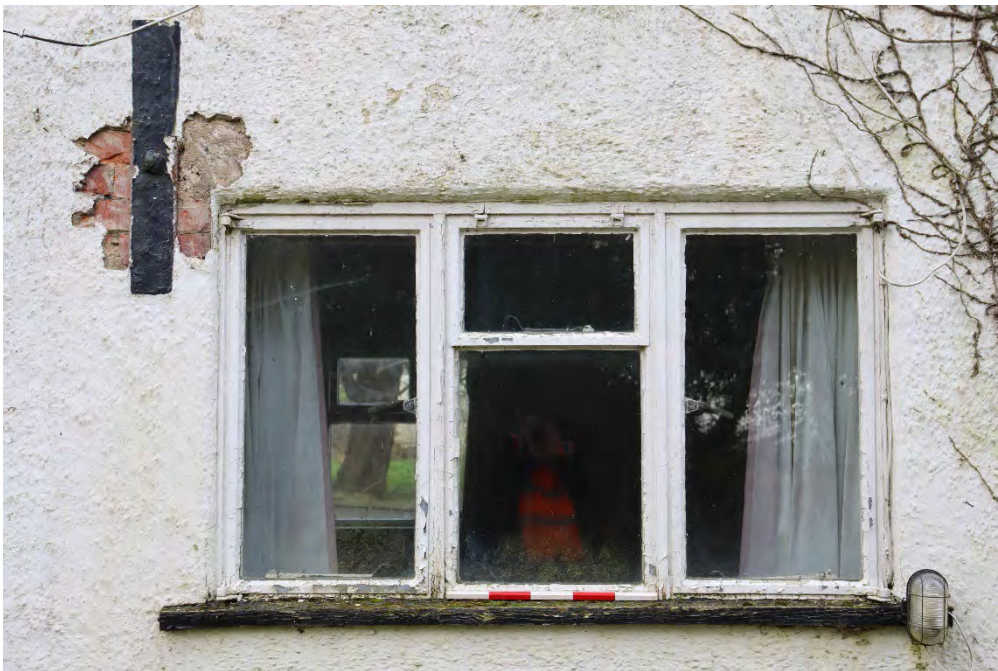
Plate 12 - Ground floor east elevation, north most window Room G7
