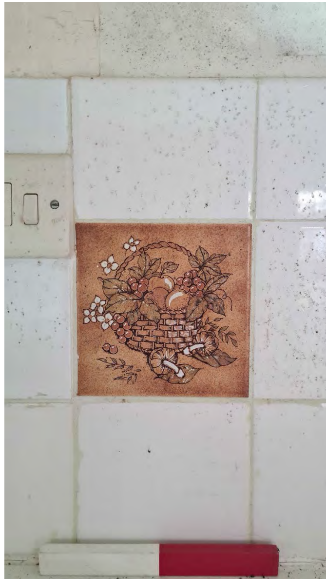
Plate 34 - Detail shot of kitchen tile Room G2
