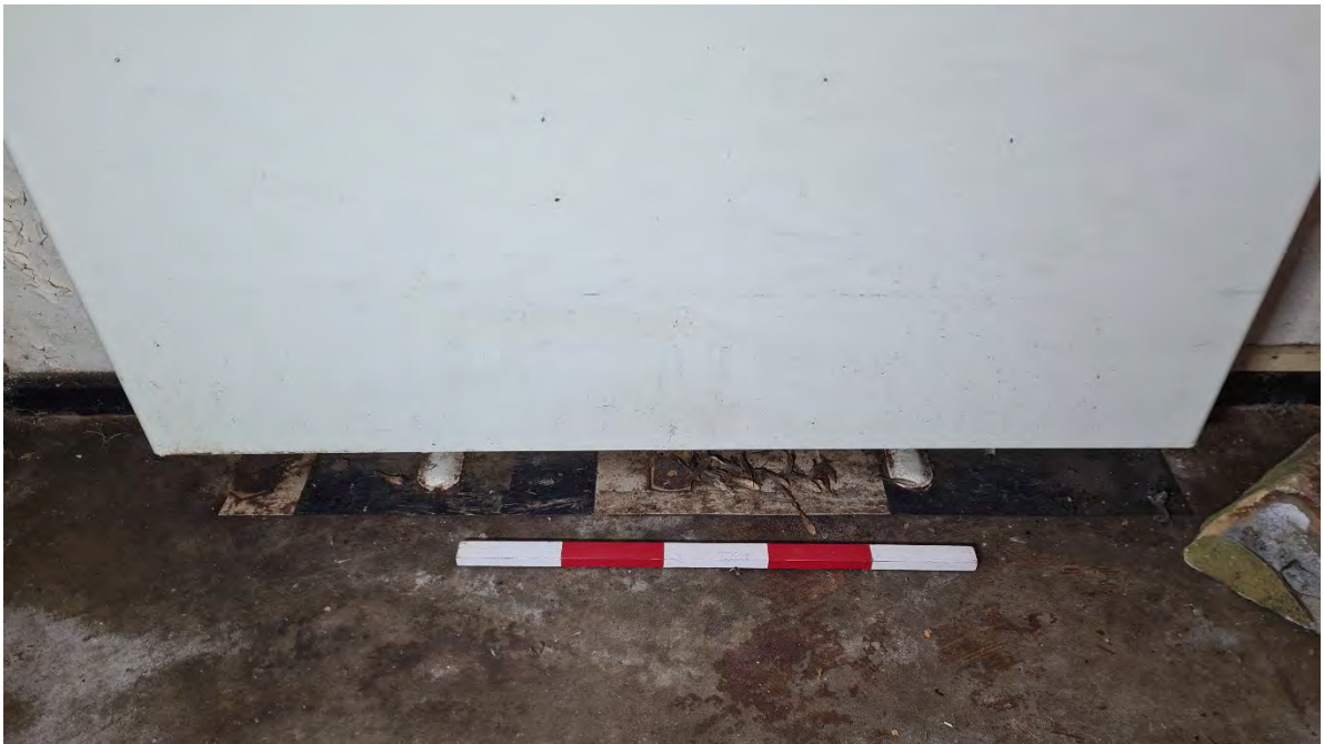
Plate 35 - North facing shot of floor Linoleum in Room G2
