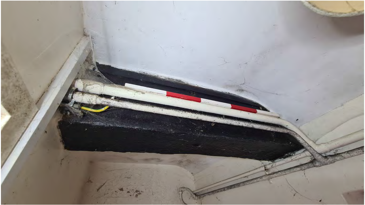
Plate 38 - Timber beam in Room G3
