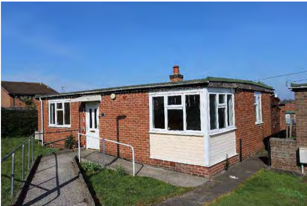
Plate 10 - North-east facing photo of bungalow 42, west elevation (front façade)
