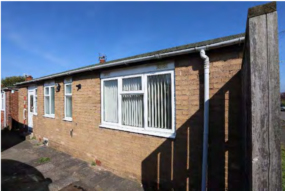
Plate 7 - North-east facing photo of bungalow 43, west elevation (rear façade)
