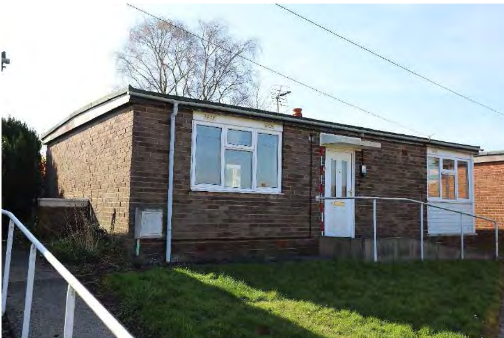
Plate 12 - North-west facing photo of bungalow 37, east elevation (front façade)
