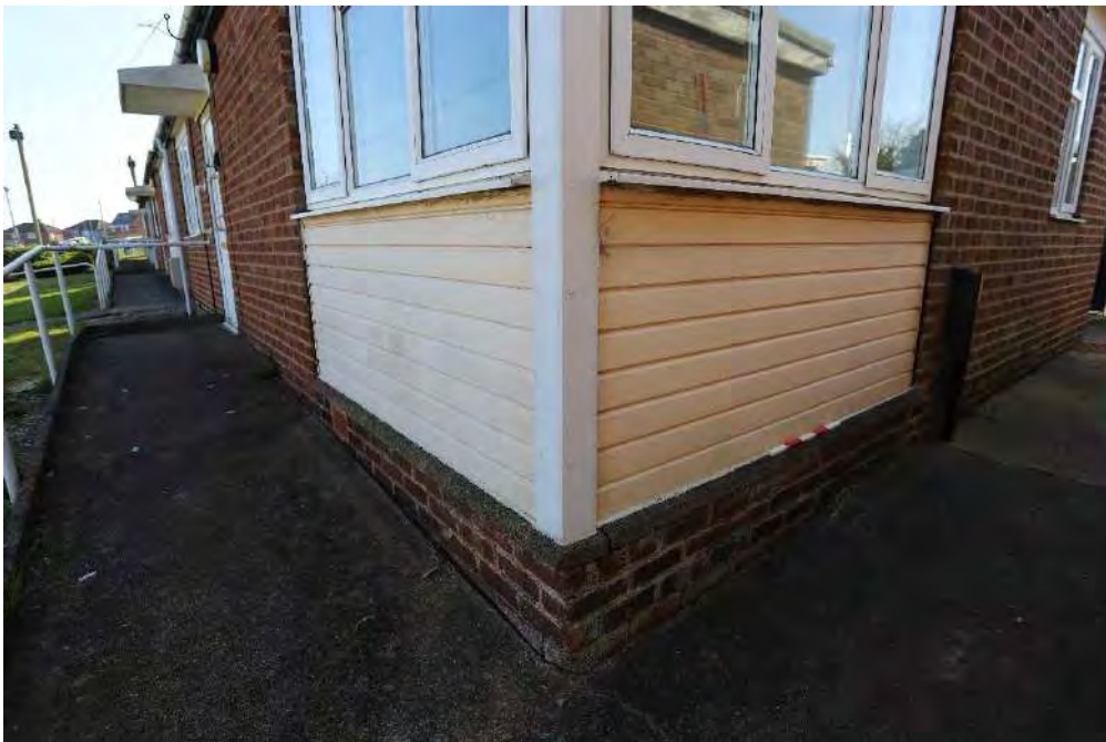
Plate 44 - South-west facing concrete sill below modern uPVC window of bungalow 45
