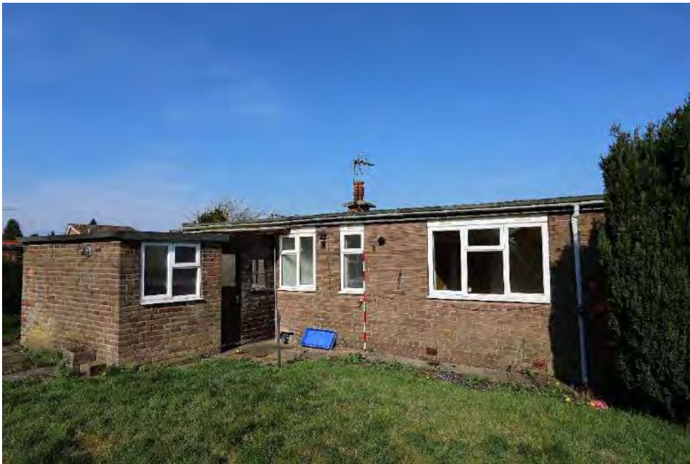
Plate 13 - North-east facing photo of bungalow 37, west elevation (rear façade)
