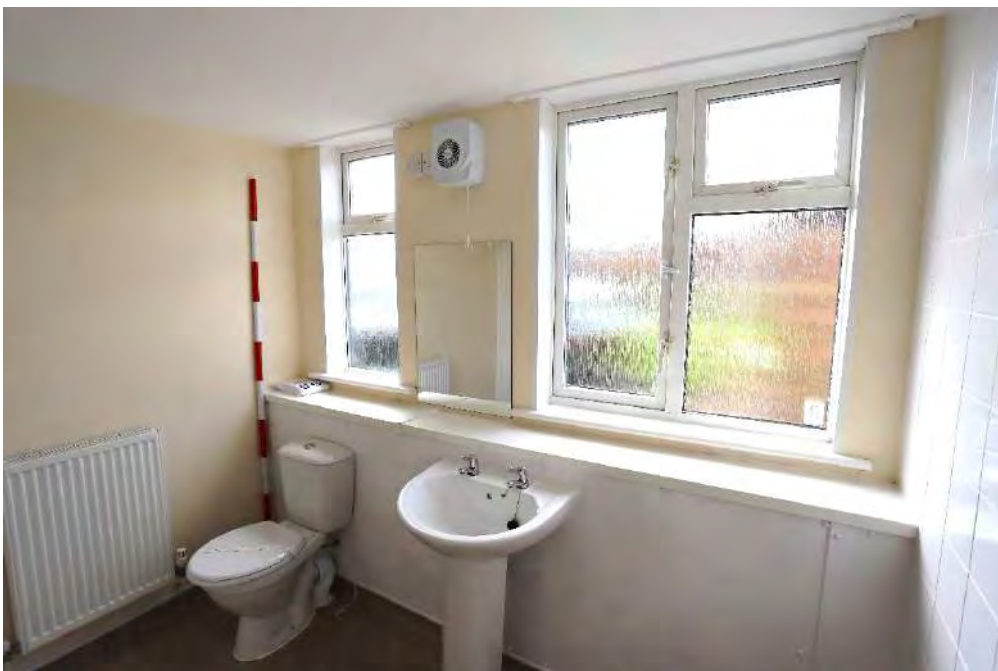
Plate 26 - West facing photo of WC room in bungalow 43
