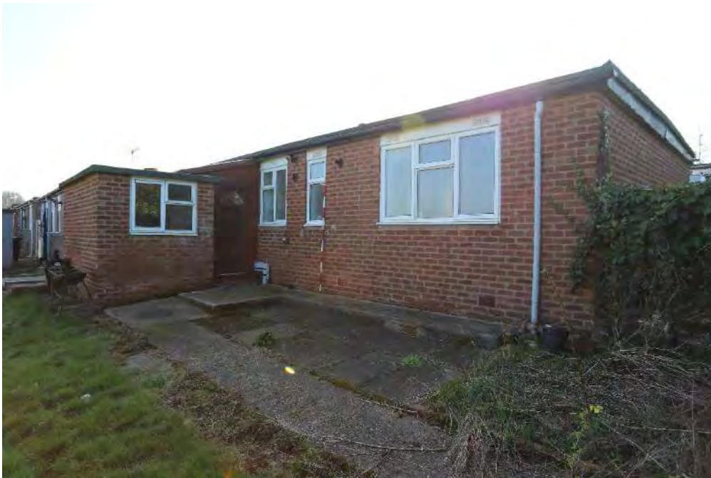
Plate 11 - South-west facing photo of bungalow 42, east elevation (rear façade)
