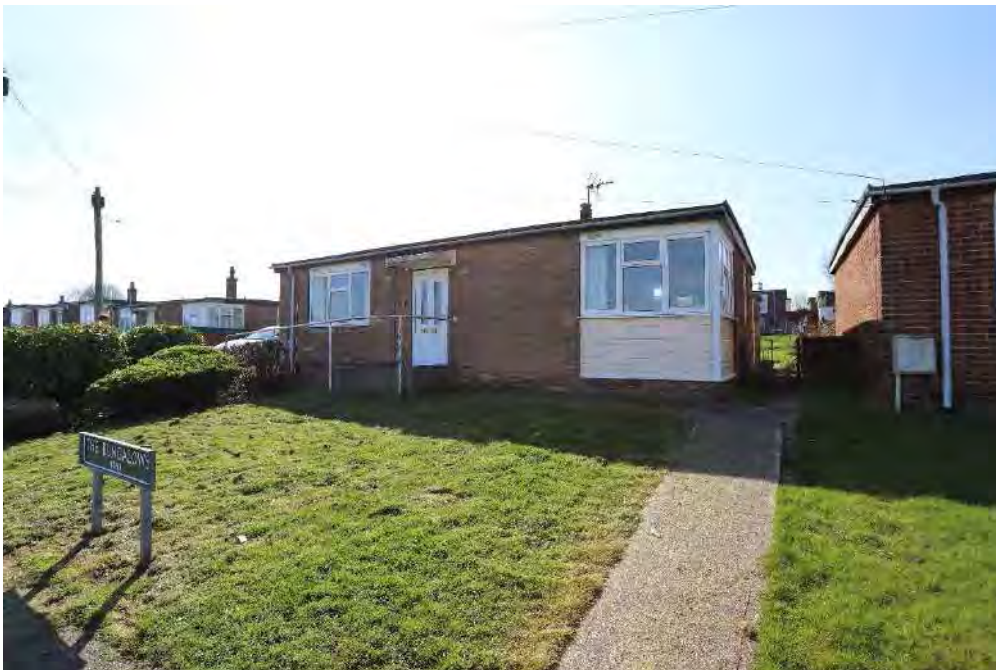
Plate 6 - South-west facing photo of bungalow 43 east elevation (front façade)
