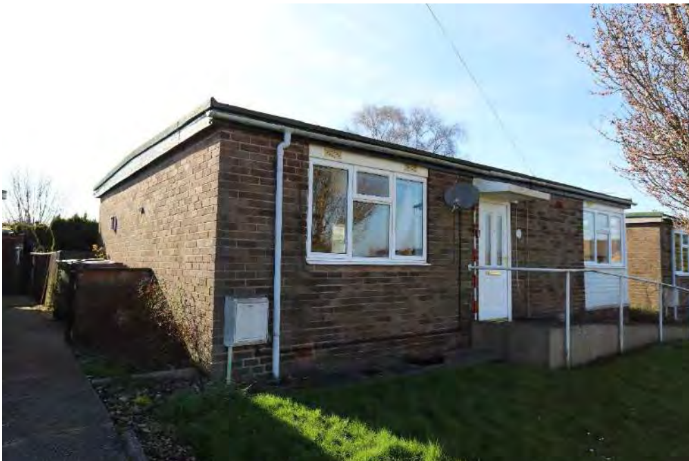
Plate 14 - North-west facing photo of bungalow 36, east elevation (front façade)
