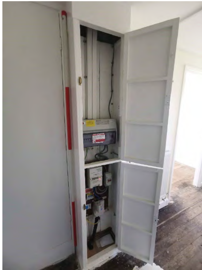
Plate 33 - North-east facing photo of utility cupboard in hallway of bungalow 45
