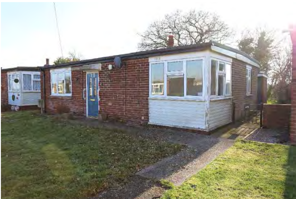
Plate 18 - South-west facing photo of bungalow 28, east elevation (front façade)
