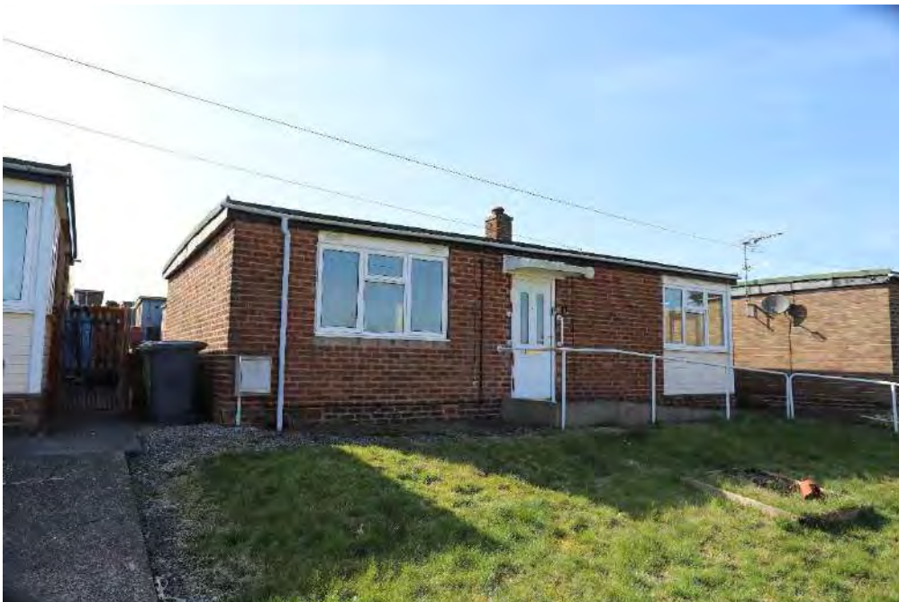
Plate 8 - South-west facing photo of bungalow 45 east elevation (front façade)
