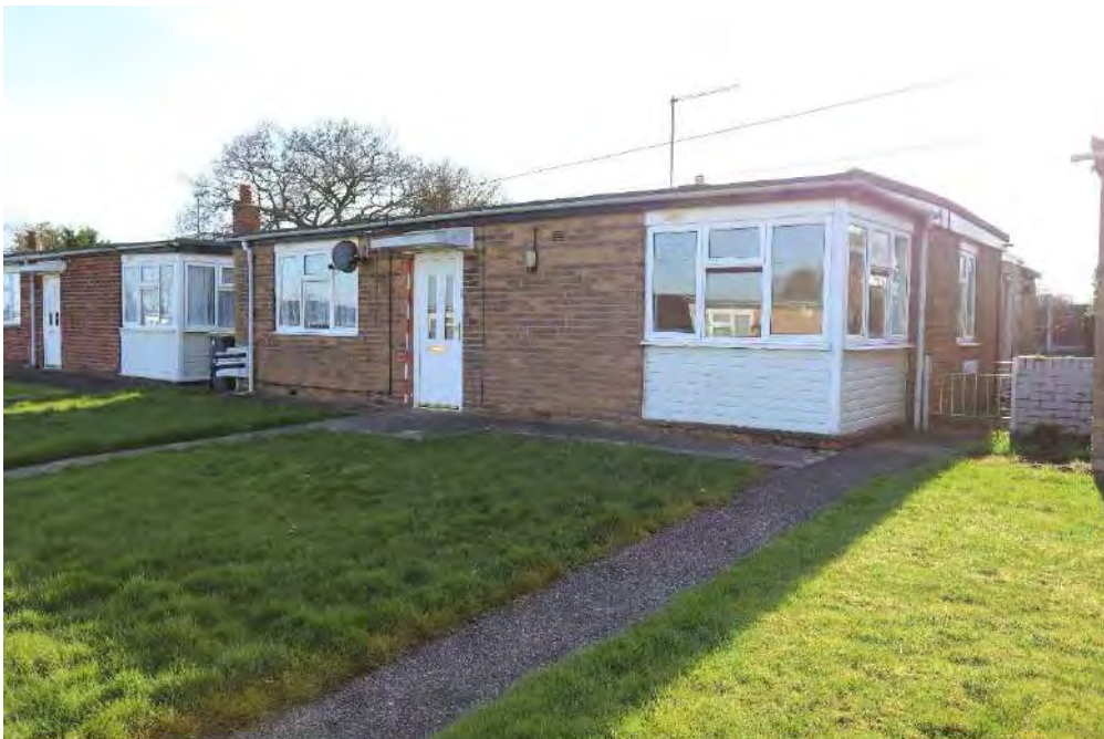
Plate 16 - South-west facing photo of bungalow 30, east elevation (front façade)
