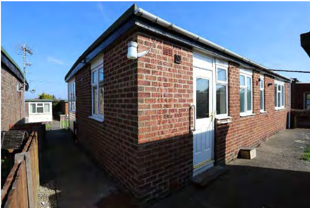
Plate 9 - North-east facing photo of bungalow 45, west elevation (rear façade)
