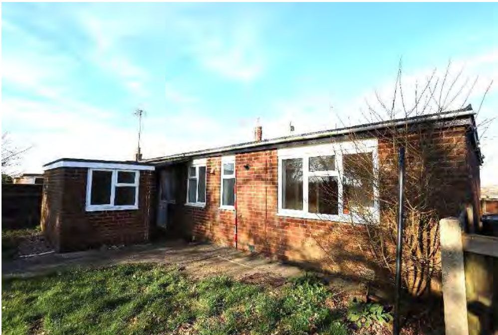
Plate 19 - North-east facing photo of bungalow 28, west elevation (rear façade)
