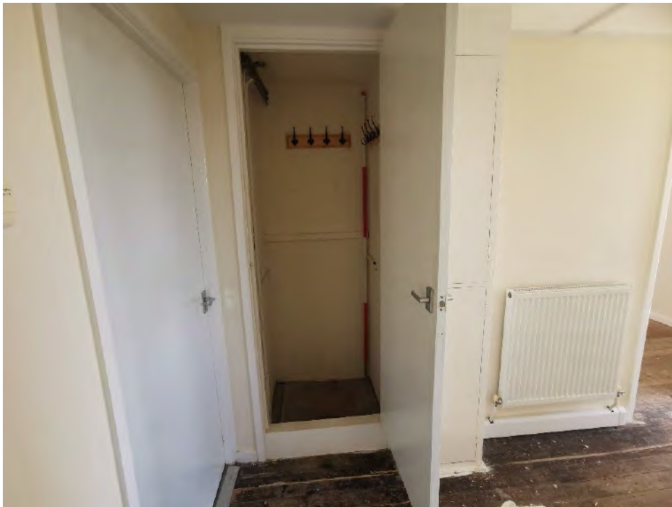
Plate 35 - North facing photo of airing cupboard/storage space in hallway of bungalow 45
