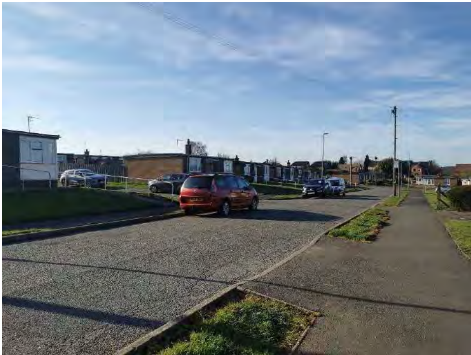
Plate 3 - North facing photo of The Bungalows
