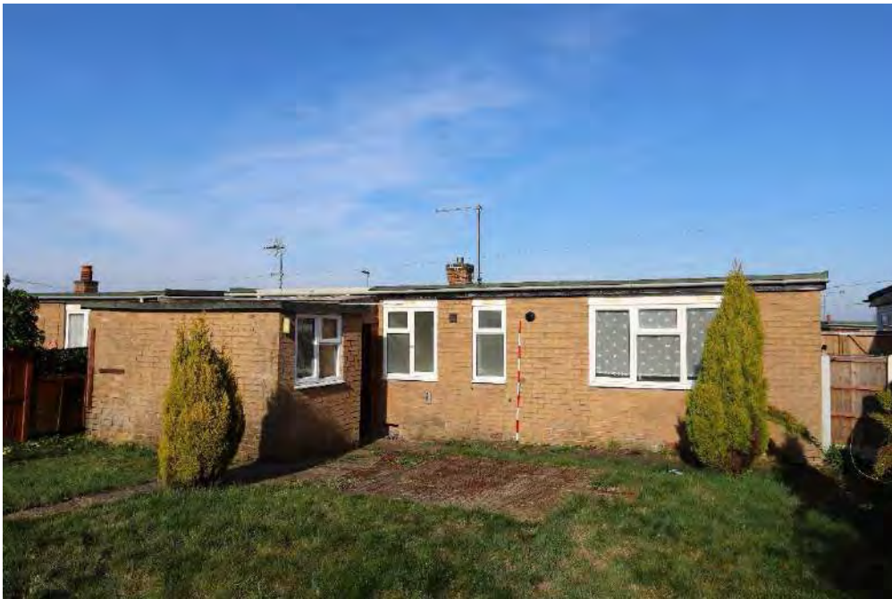
Plate 17 - East facing photo of bungalow 30, west elevation (rear façade)
