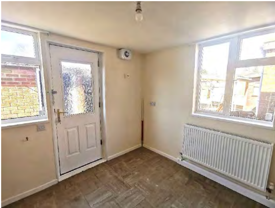
Plate 25 - North-west facing photo of north-west kitchen room in bungalow 45
