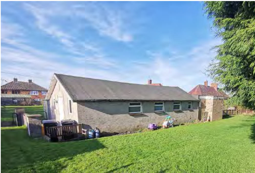
Plate 47 – South facing photo of Village Hall/Pre-school
