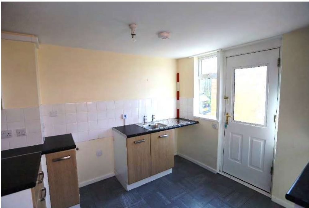
Plate 24 - South-west facing photo of north-west kitchen room in bungalow 43
