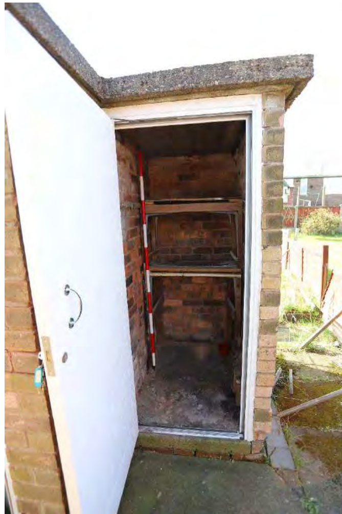
Plate 40 - West facing photo of coal shed of bungalow 43
