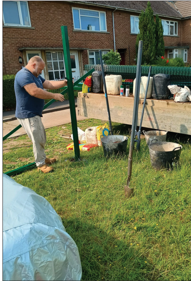
Figure 32. Fencing works in progress, looking southwest
