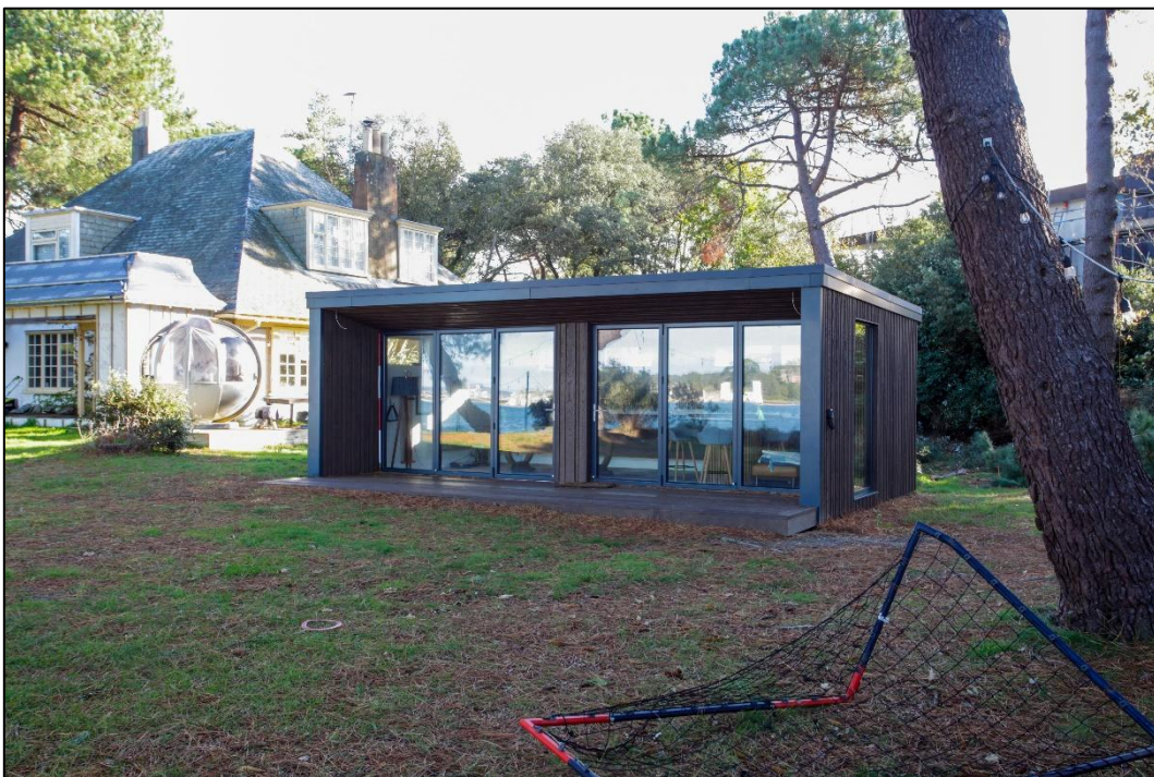
Plate 16. Modern outbuilding southwest of site
