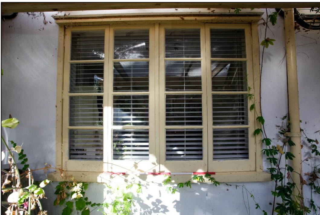
Plate 4. East elevation ground-floor window detail
