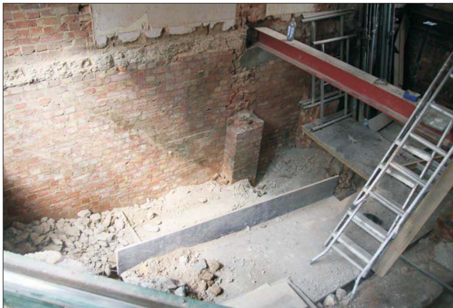
Plate 2: Internal basement wall with buttress
