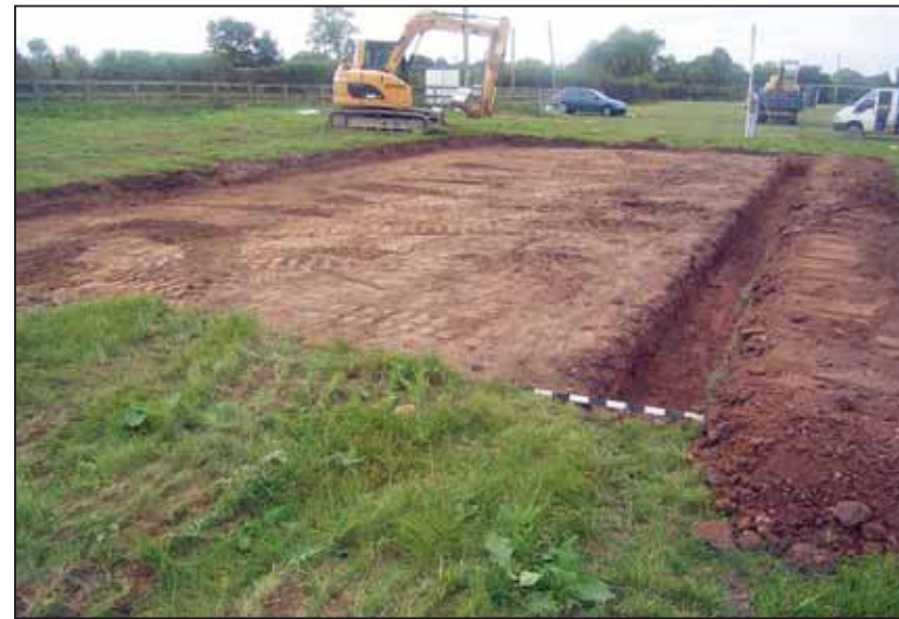
Plate 4: Stripped barn footprint and northern foundation trench viewed from the east
