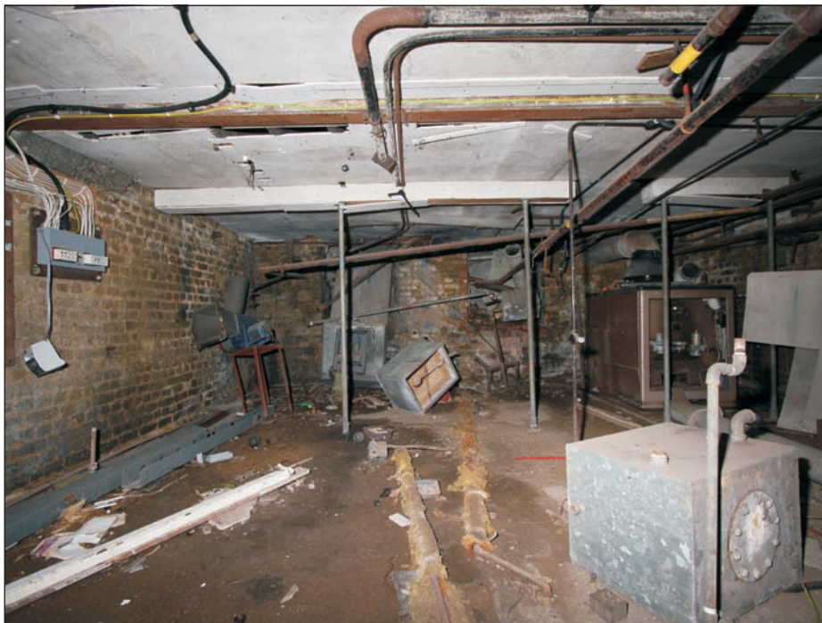
Plate 20: View of basement below link building. Looking south
