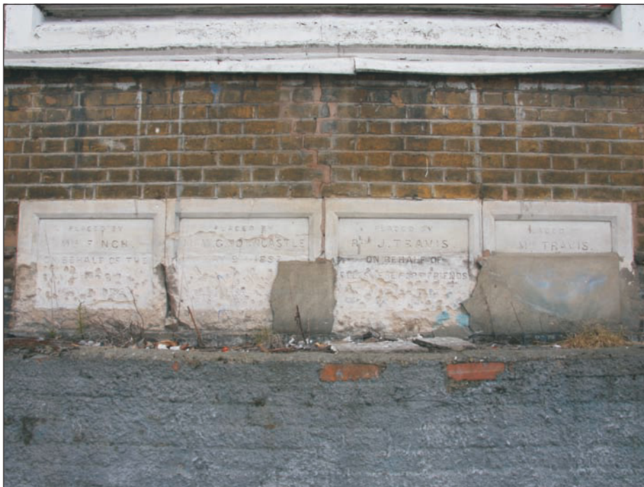
Plate 6: Foundation stones, main elevation of chapel. Looking east
