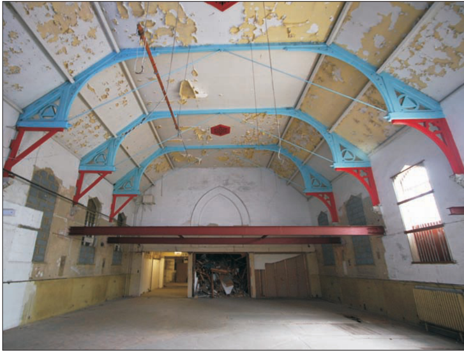
Plate 7: Interior of Main Worship Space. Looking east
