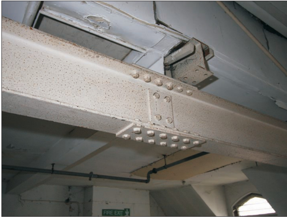
Plate 19: Detail of rolled steel joist, first floor, Hall. Looking north-east
