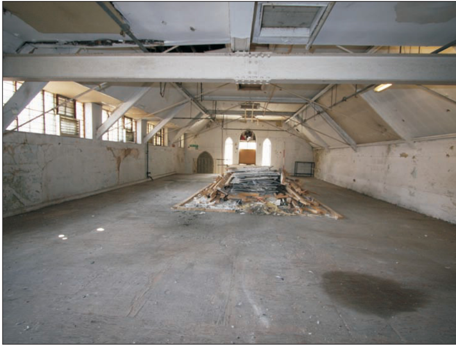
Plate 17: First floor interior, Hall. Looking south
