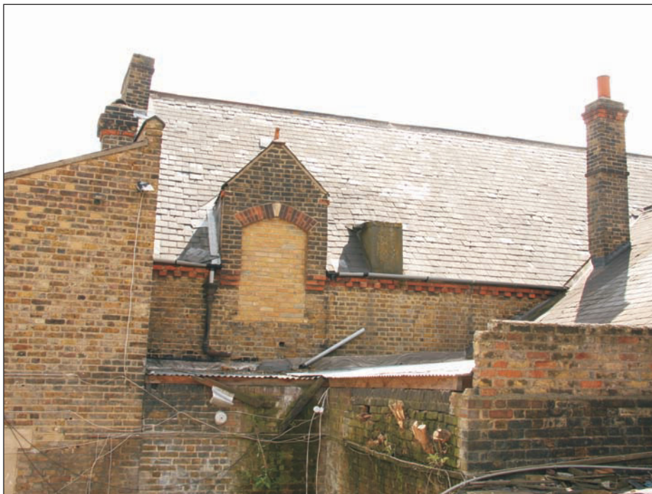
Plate 14: Western elevation of Hall showing dormer window. Looking south-east
