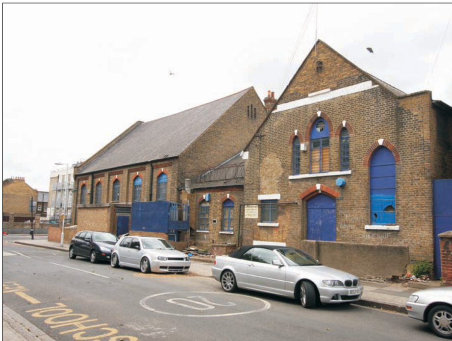
Plate 2: View along Doris Road showing southern elevation of chapel buildings. Looking north-west
