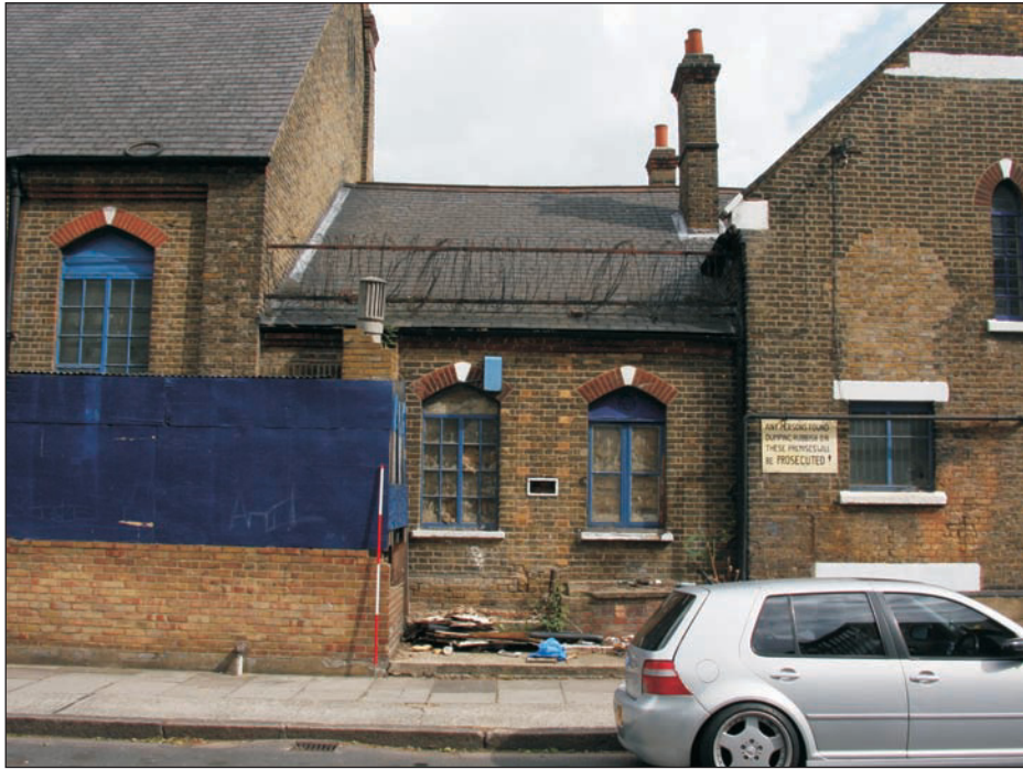
Plate 11: Southern elevation of Link Building. Looking north
