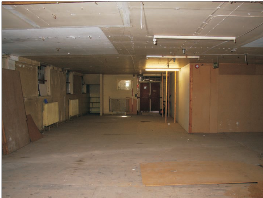
Plate 16: Ground floor interior, Hall. Looking south
