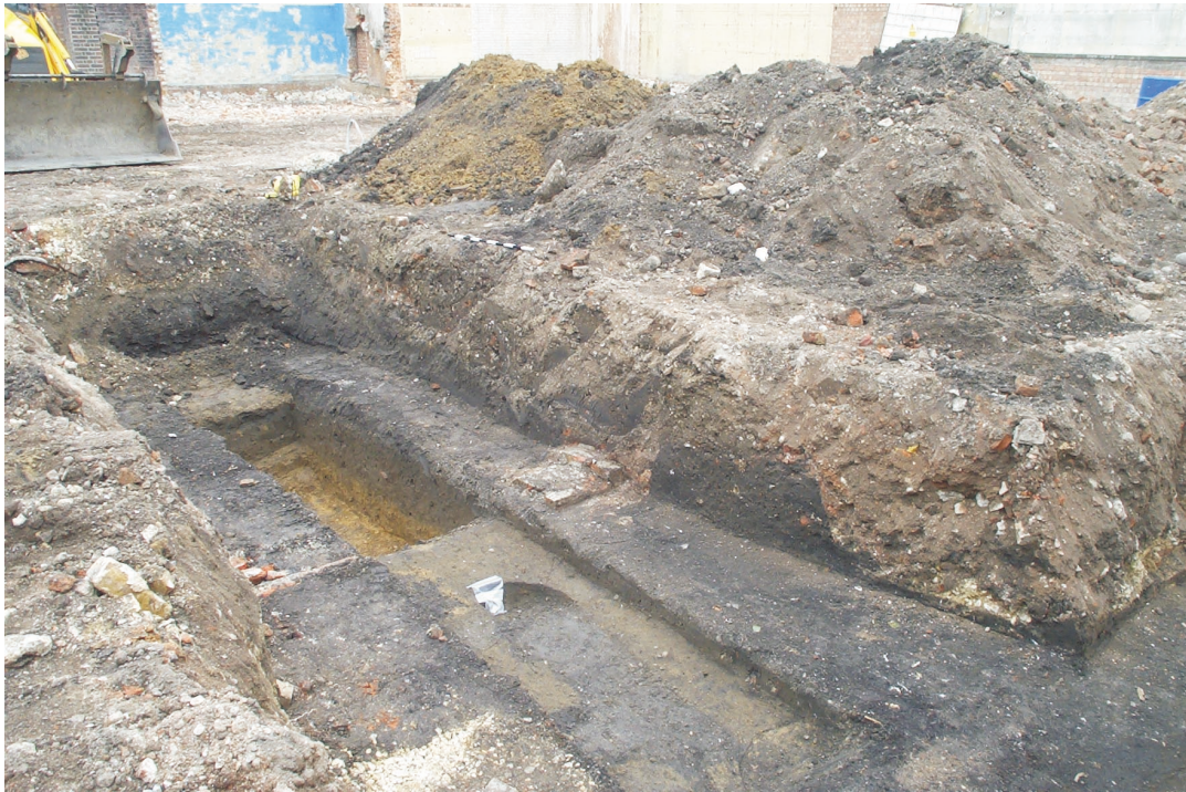
Figure 8: Trench 2 showing sondage, from the northeast (Scale 1m)
