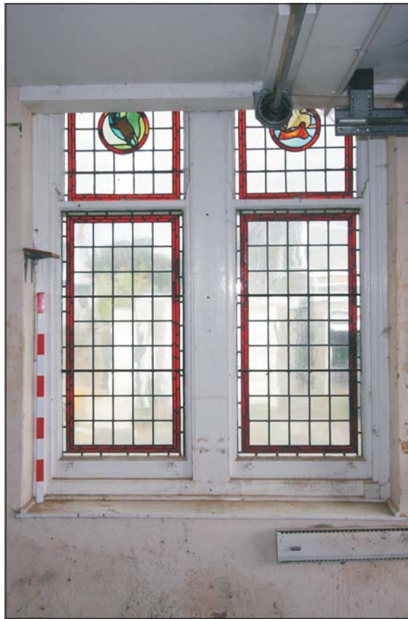
Plate 7: Window situated in the north-west wall of the Lifeboat Station
