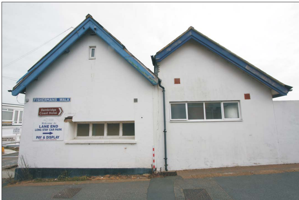
Plate 8: South-west gable ends of the Lifeboat Station and adjoining Extension
