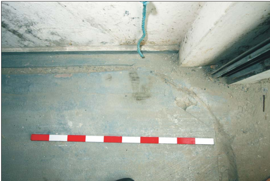
Plate 4: Curved track for former door set within the floor of the Boathouse
