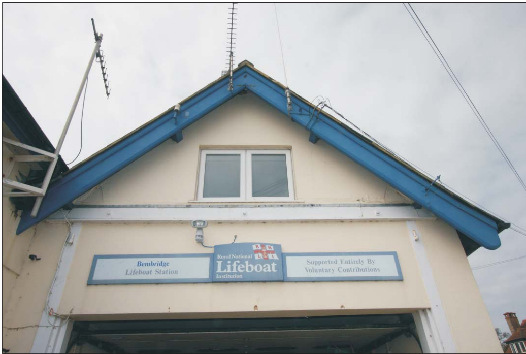
Plate 5: Top half of the north-east gable end featuring remnant iron hinges
