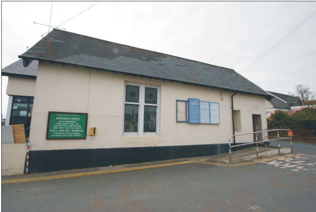
Plate 6: North-west elevation of the Lifeboat Station
