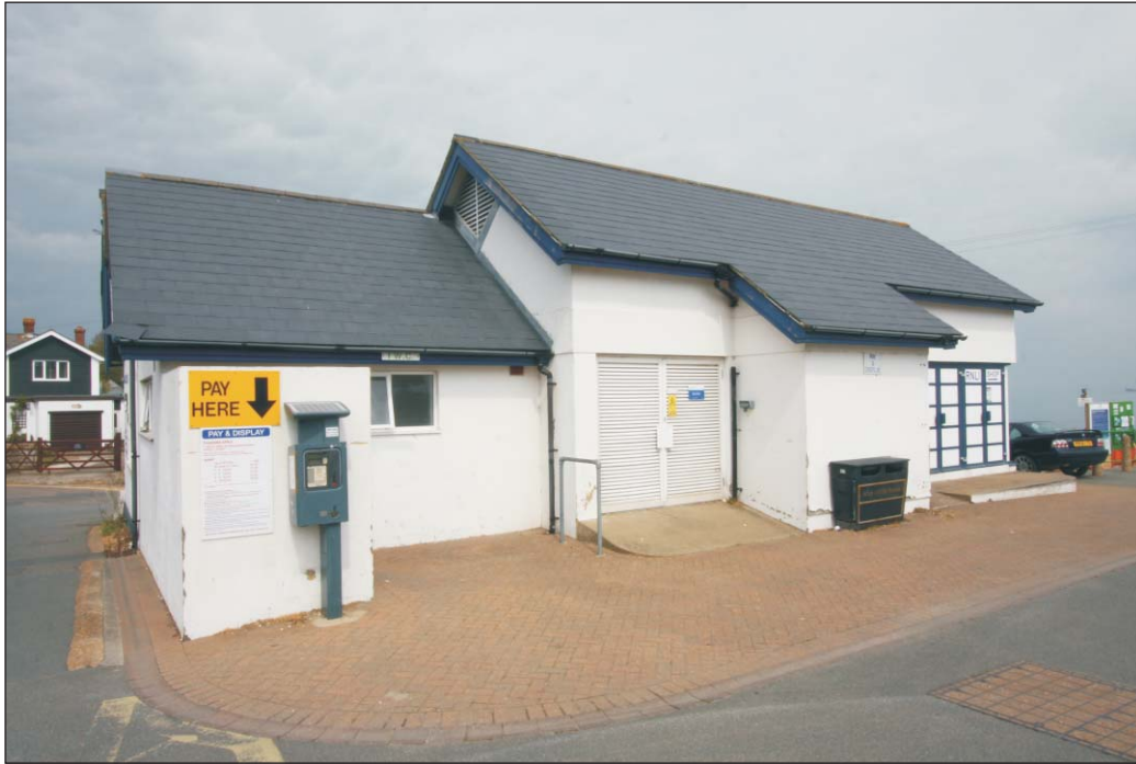
Plate 17: Extension viewed from the south
