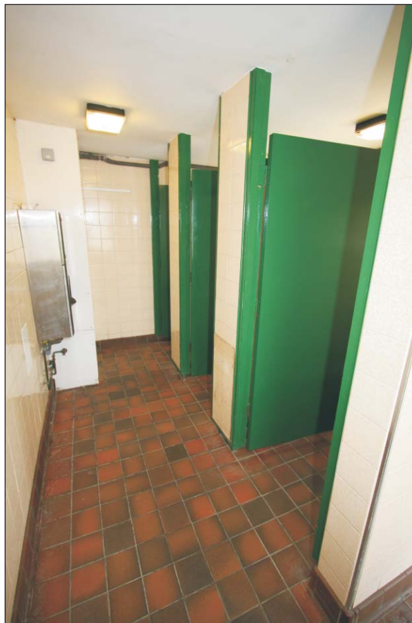
Plate 12: Ladies public toilets viewed from the north-west
