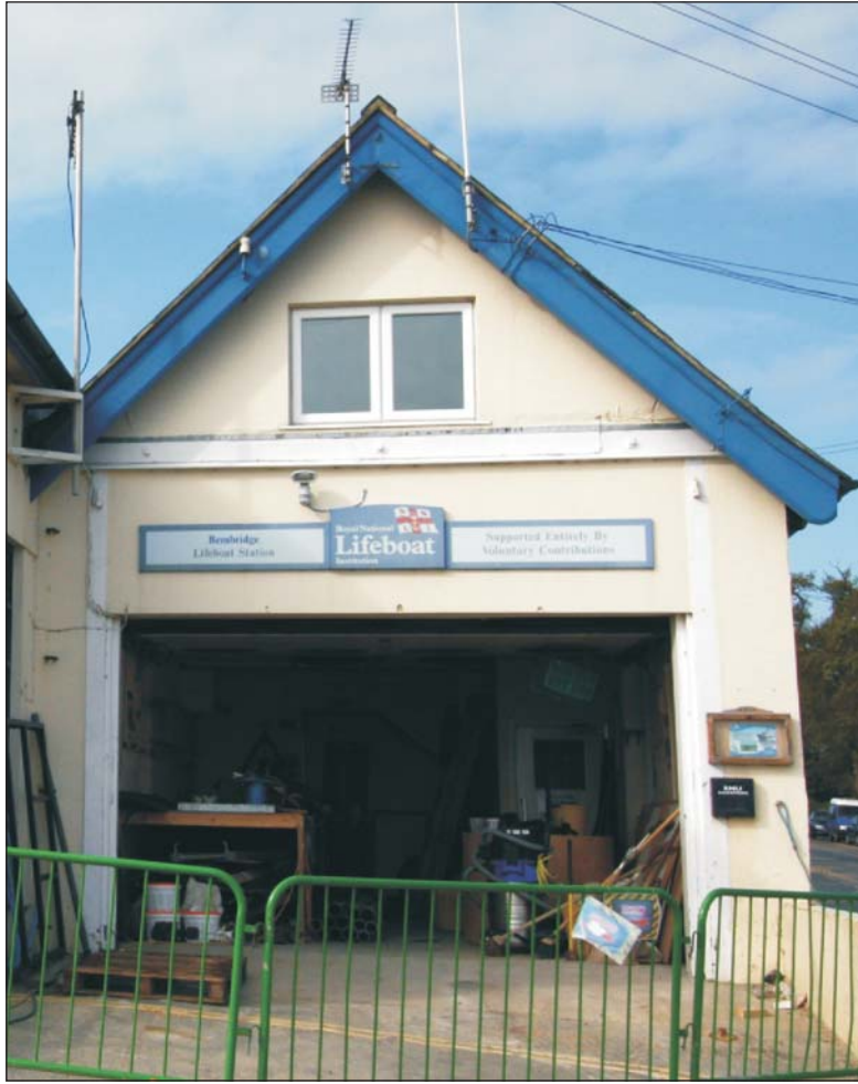
Plate 3: North-east elevation of the Lifeboat Station
