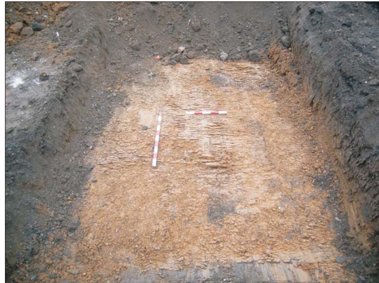
Plate 1: Area stripped for services, viewed from the south
