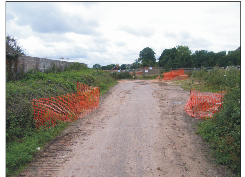
Plate 8: Location of service investigation pit
