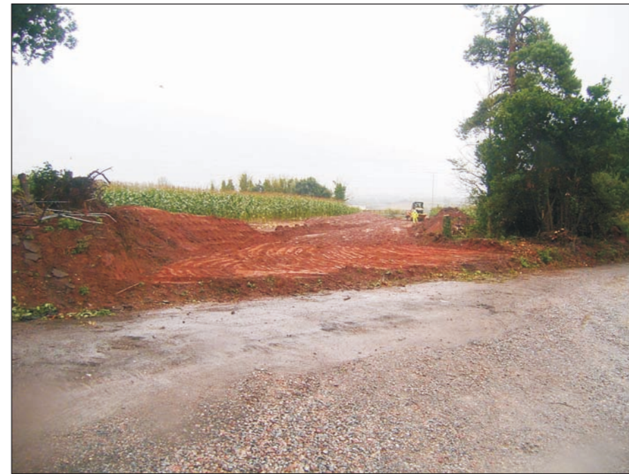
Plate 15: Redhayes Lodge Haul Road extension
