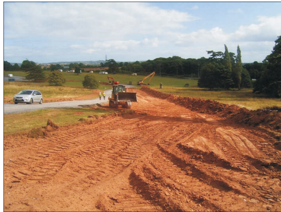
Plate 14: Haul Road widening
