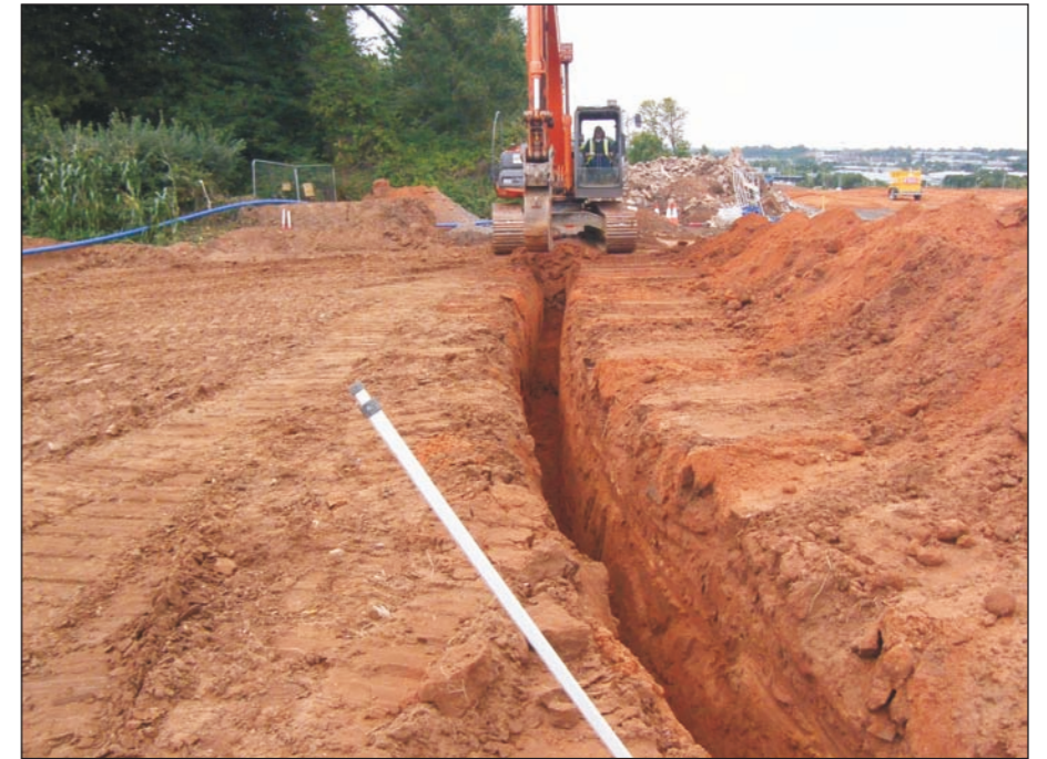
Plate 13: Water main diversion, north of Blackhorse Lane
