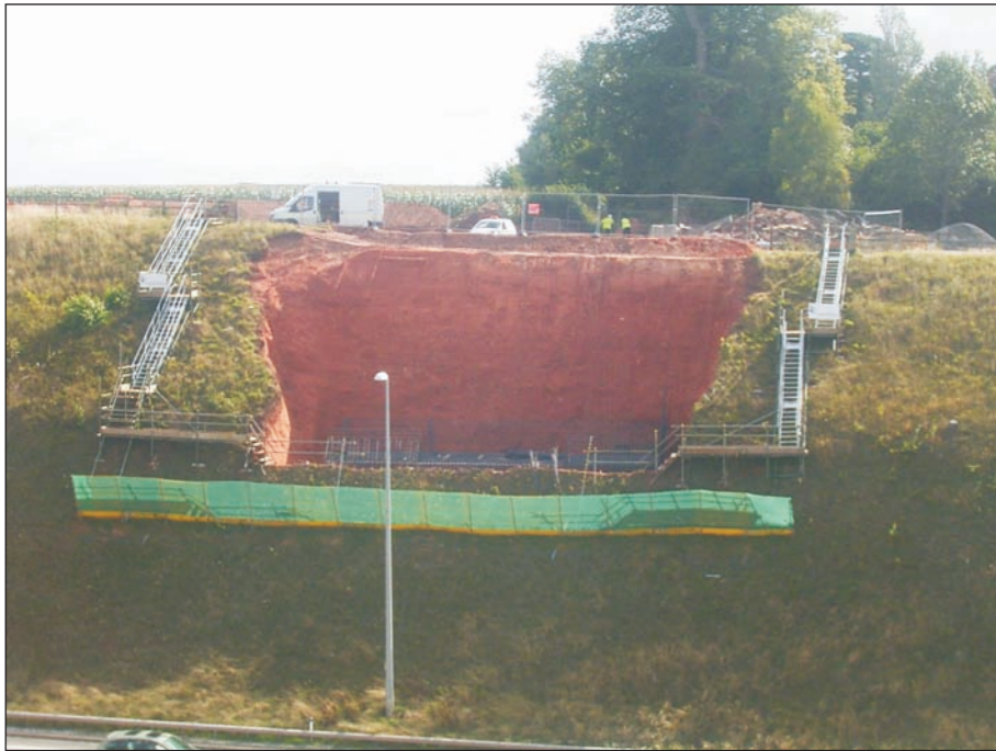
Plate 11: Reduction of embankment on eastern side
