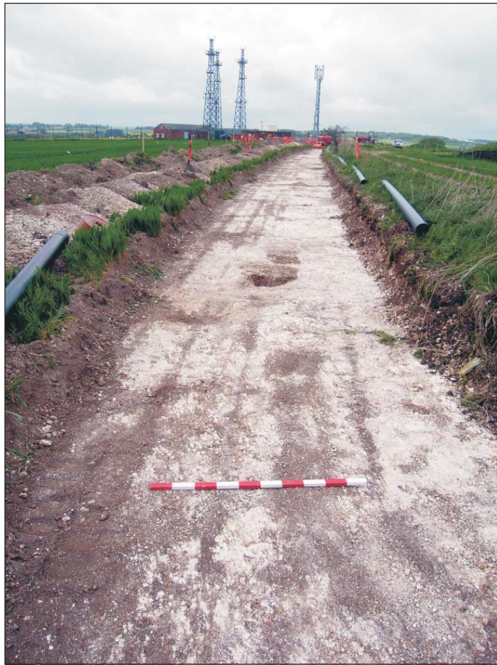
Plate 5: General view towards Area F from the west
