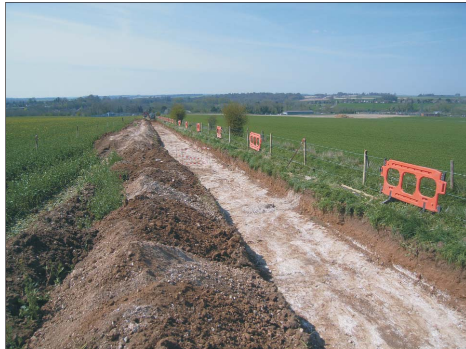
Plate 1: General view of Area C to D from the north east
