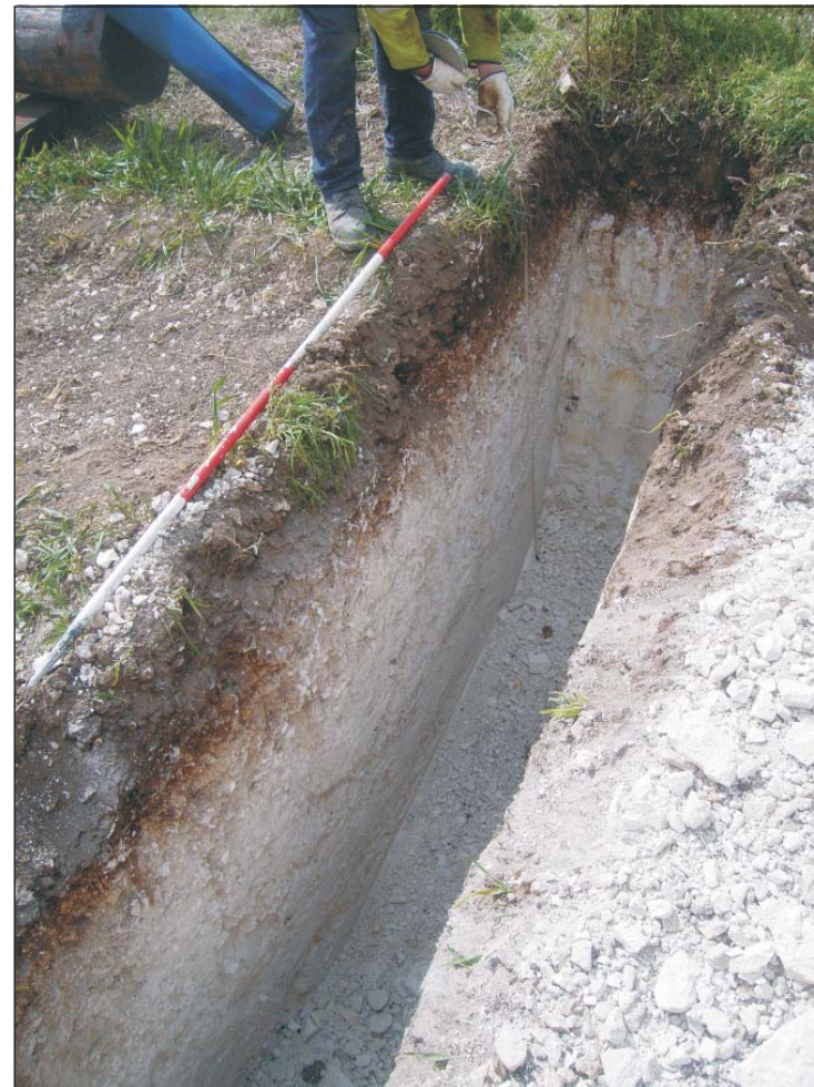
Plate 7: Trench for double electricity poles
