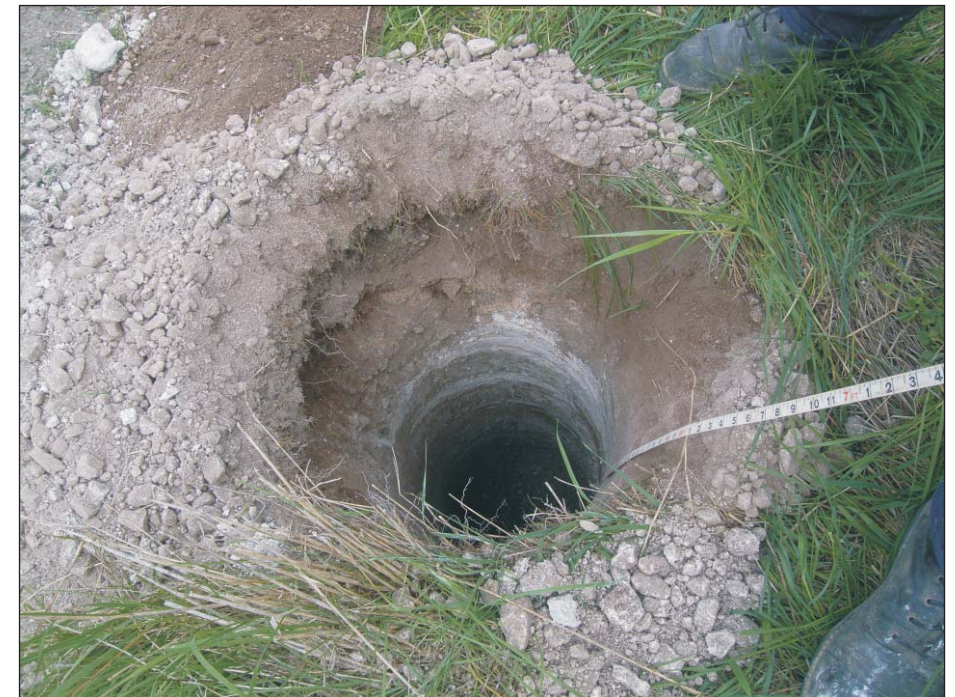
Plate 8: Screw-bored pole hole 106
