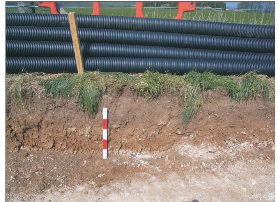
Plate 4: South facing section of Area D to F
