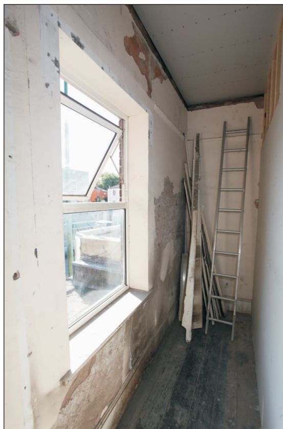
Plate 12: Storeroom showing residual decorative elements on the south and east walls
