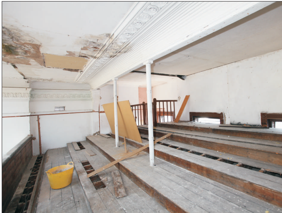
Plate 15: Second floor Gallery viewed from the south-west
