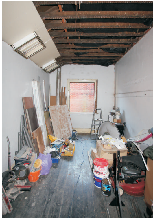
Plate 14: Storeroom to the north of St Mary's Hall
