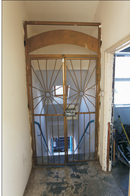
Plate 13: Access to back staircase to the north of St Mary's Hall
