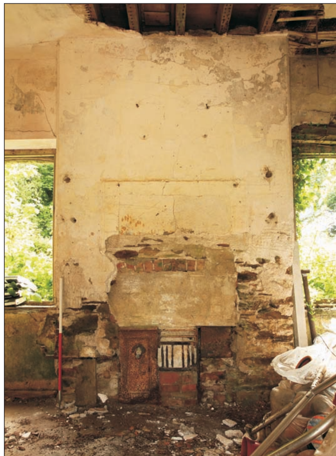
Plate 8: Detail of original Victorian fire grate, water tank and evidence of fire surround east room ground floor A
