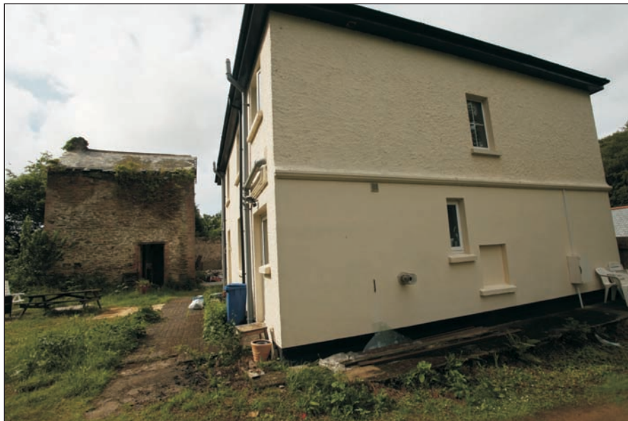
Plate 14: 1930's houses built on the site of the original coach house north wing
