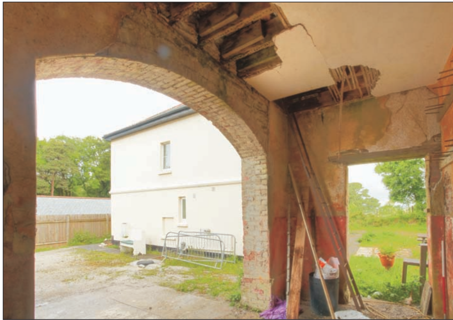
Plate 9: Covered porch area showing iron pole ladder access to first floor
