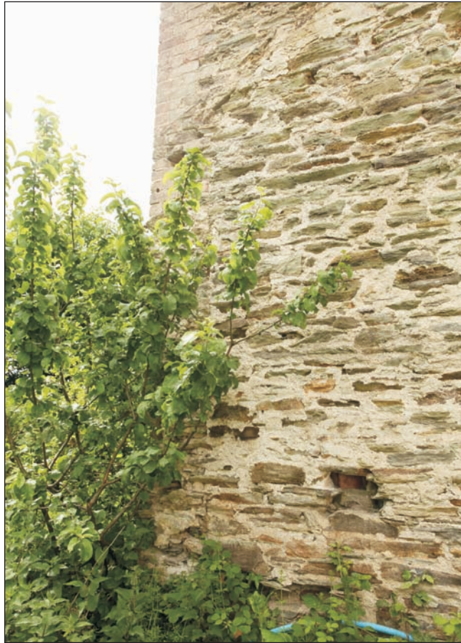
Plate 3: Evidence of original stone wall and brick quoins at north-east corner of central element A
