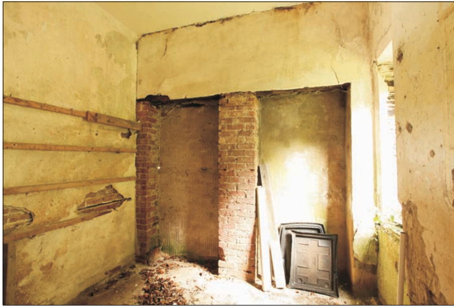
Plate 7: Cupboard recesses in north wall of east ground floor room
