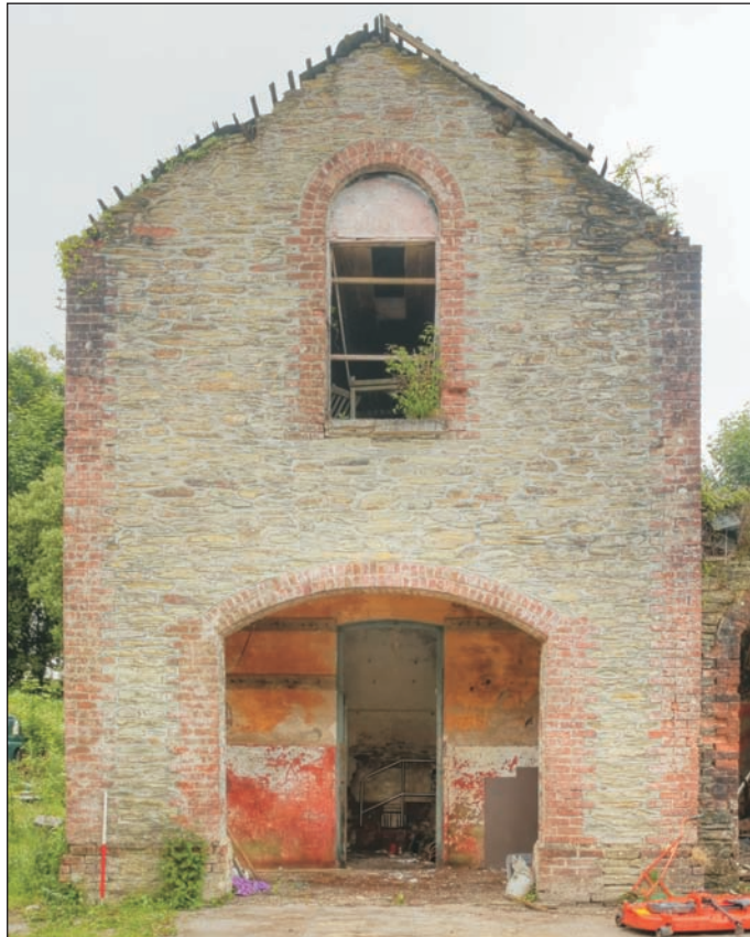
Plate 1: Two storey element A west facing elevation
