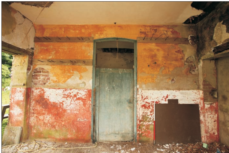
Plate 5: Central porch area showing door access into east room office/bothy
