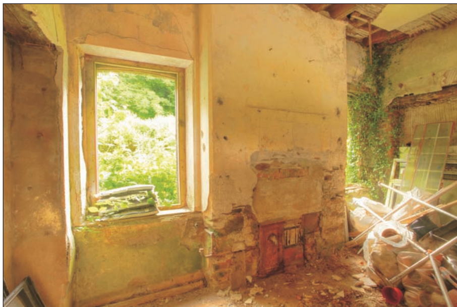
Plate 6: Ground floor east room showing original window openings either side of chimney
