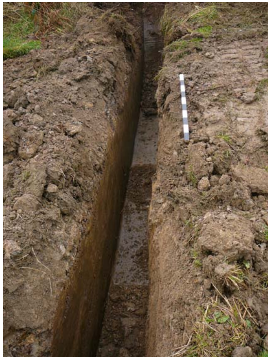
Plate 2: View from the northeast showing pipe trench into natural clays.
