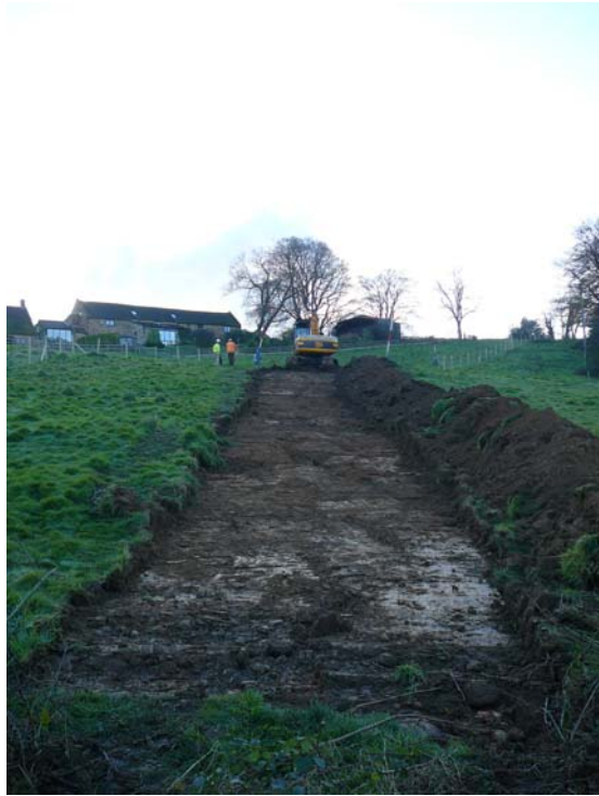
Plate 1: View from the northeast looking southwesterly along the top and subsoil strip.
