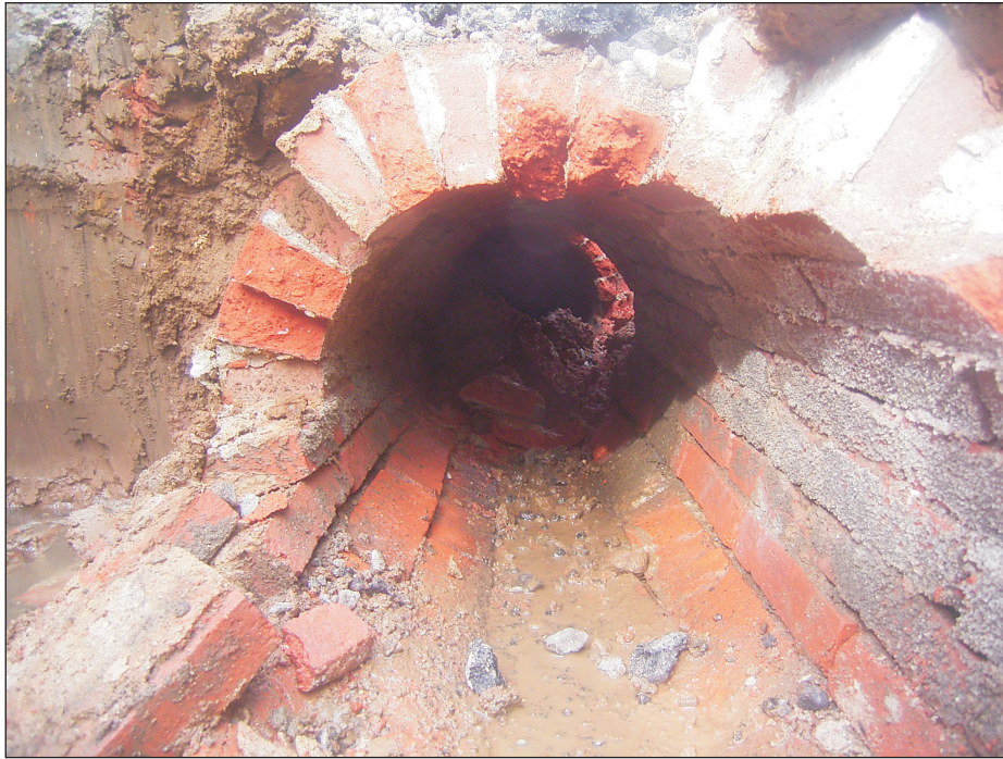
Plate 1: Culvert in Trench 12
