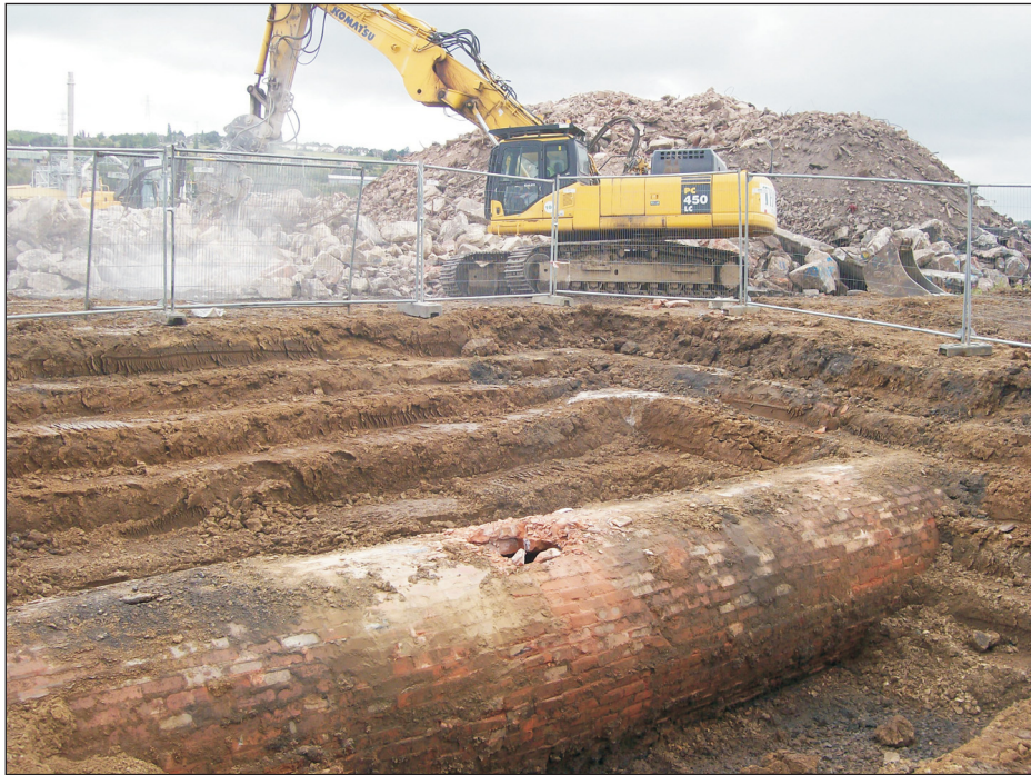
Plate 2: Culvert 2, looking north east.
