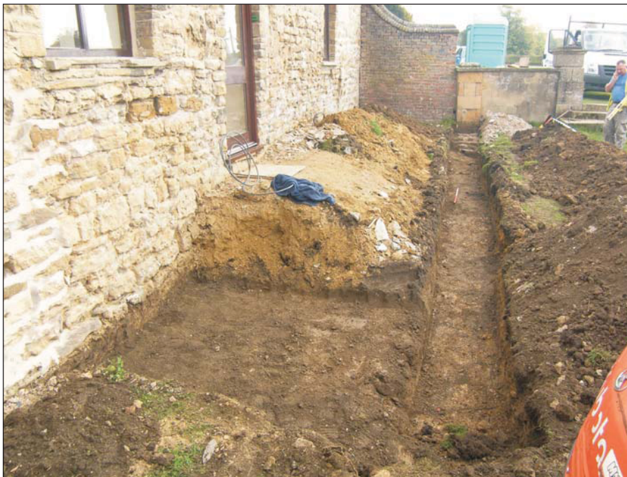
Plate 6: General view of Trench 2, looking east
