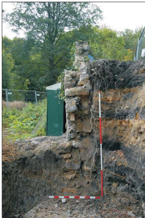
Plate 4: Detail of north facing section of the Western Retaining Wall
