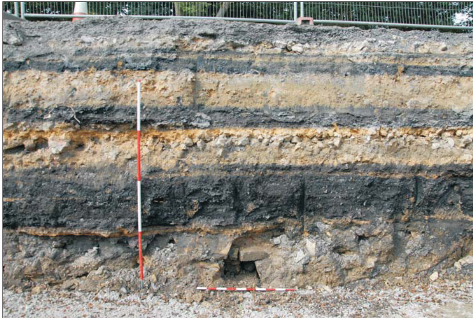
Plate 5: Detail of east facing section of Trench 1 showing sequence of road surfaces and culvert at the base
