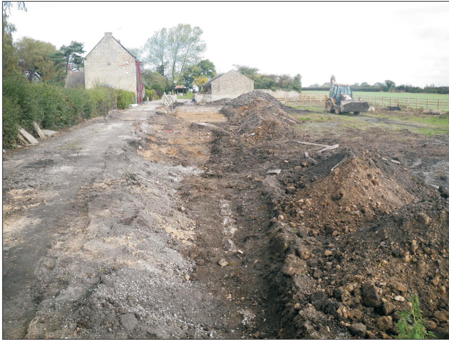
Plate 1: Site fully excavated, looking north.
