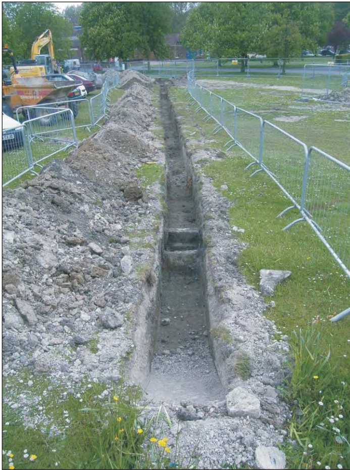
Plate 1: Pipe trench in WXC605, looking south
