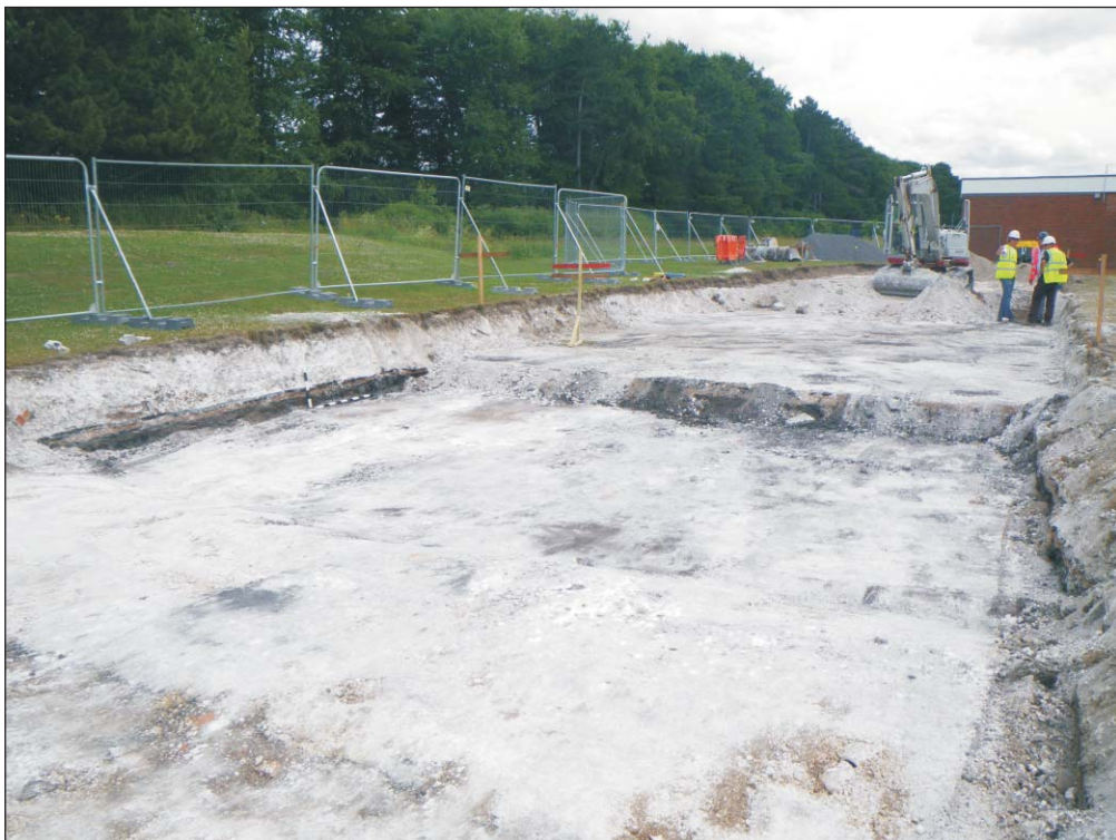
Plate 2: View of access road showing made ground layers
