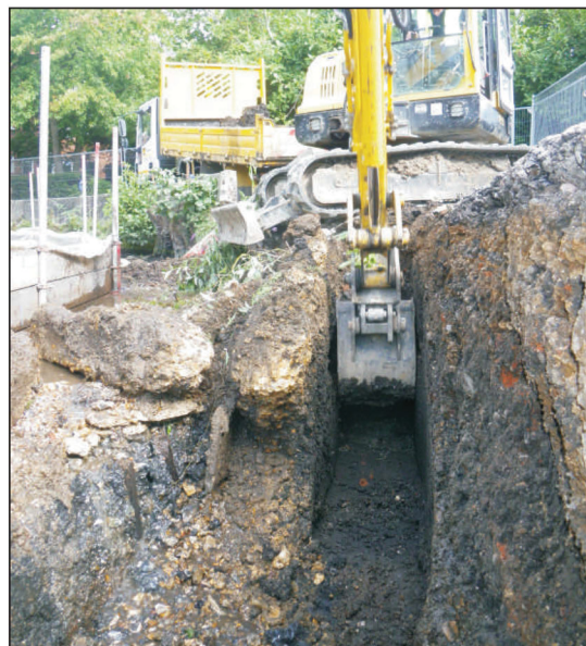
Plate 5: Removal of existing retaining wall
