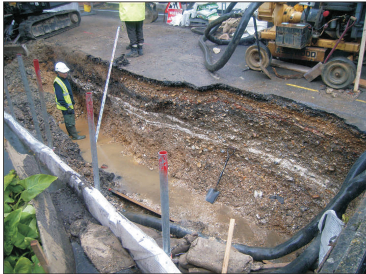
Plate 4: Exposed section after removal of existing retaining wall
