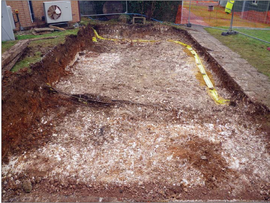
Plate 5: Overview of Area 3 from the south
