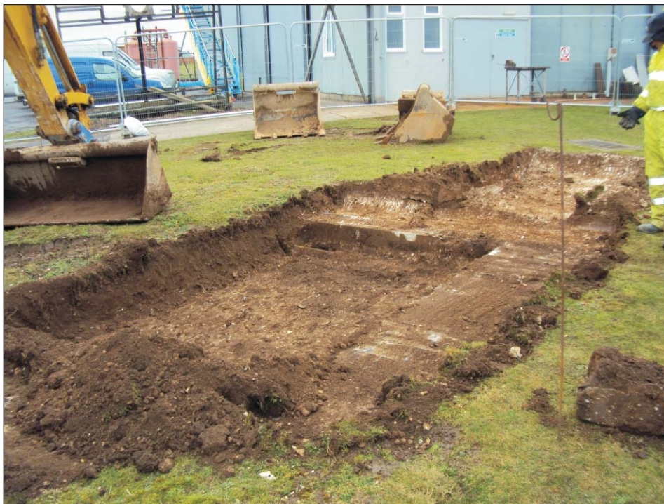
Plate 2: Fuel tank location: During excavation, looking northwest
