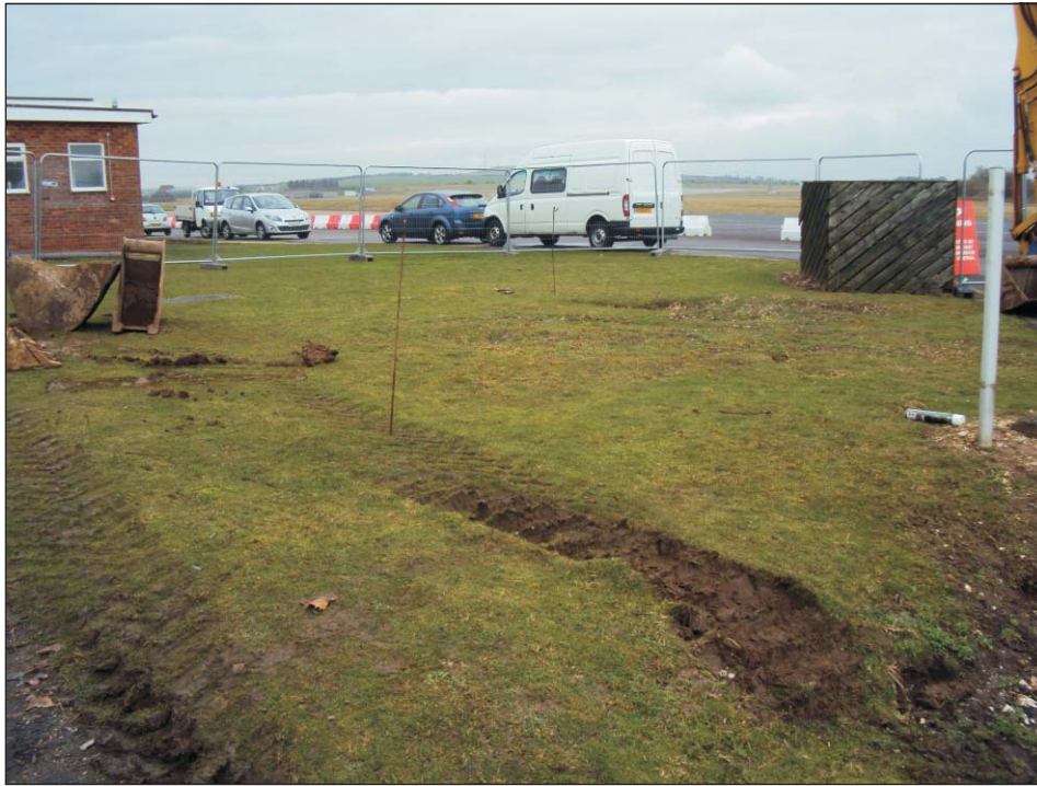
Plate 1: Proposed fuel tank location: Pre-excavation, looking northeast
