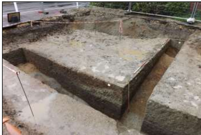
AREA 1 LOOKING NORTHWEST; SHOWING TERMINUS OF DITCH 1, AS WELL AS PART OF BANK 1
