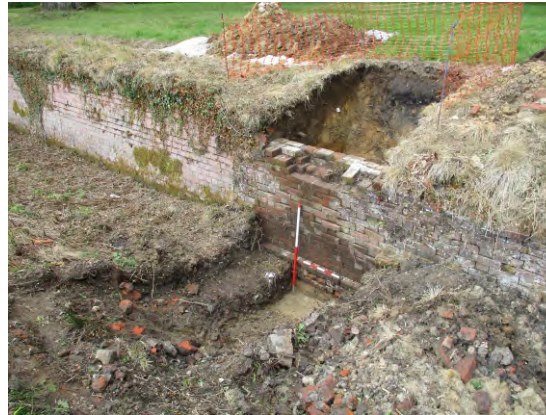
PHOTOGRAPH 40: TEST PITS 2 AND 3, LOOKING WEST
