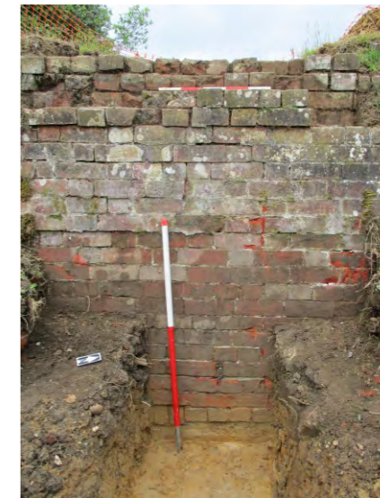
PHOTOGRAPH 35: TRENCH 9 LOWER, HA HA WALL (9002) LOOKING WEST
