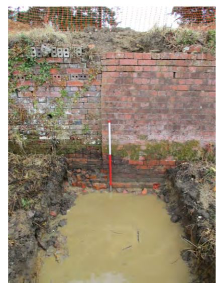
PHOTOGRAPH 31: TRENCH 8 LOWER, HA HA WALL (8001/2) LOOKING WEST
