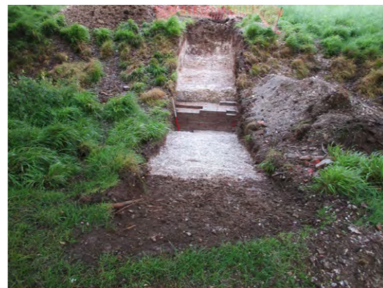
PHOTOGRAPH 24: TRENCH 6, LOOKING NORTHWEST
