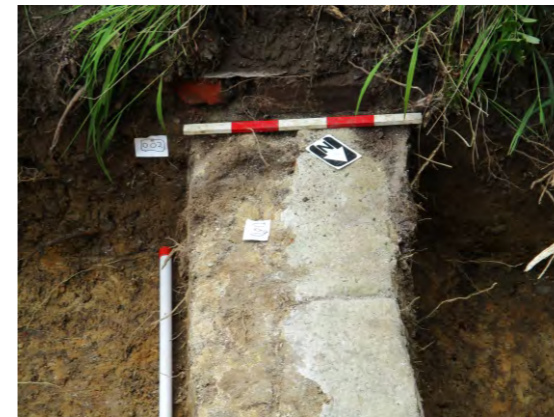
PHOTOGRAPH 39: TEST PIT 1, KERB / EDGING (101)/(123) DETAIL
