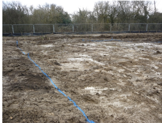
PHOTOGRAPH 2: COMMENCEMENT OF SUBSOIL STRIP
