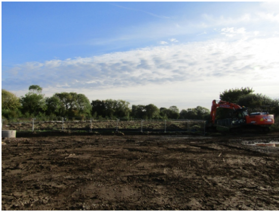
PHOTOGRAPH 1: TOPSOIL STRIP IN PROGRESS
