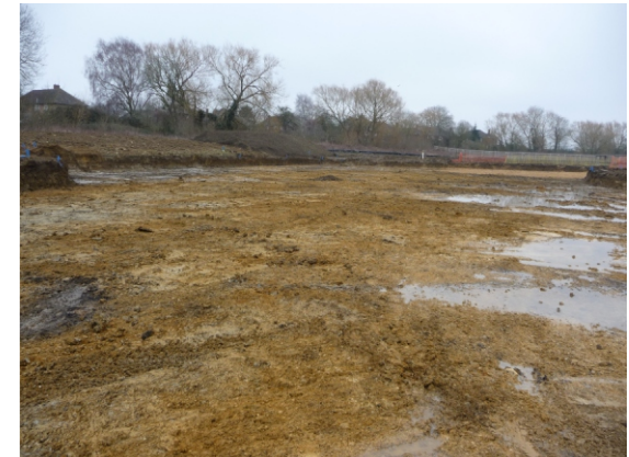
PHOTOGRAPH 3: COMPLETION OF MECHANICAL STRIP
