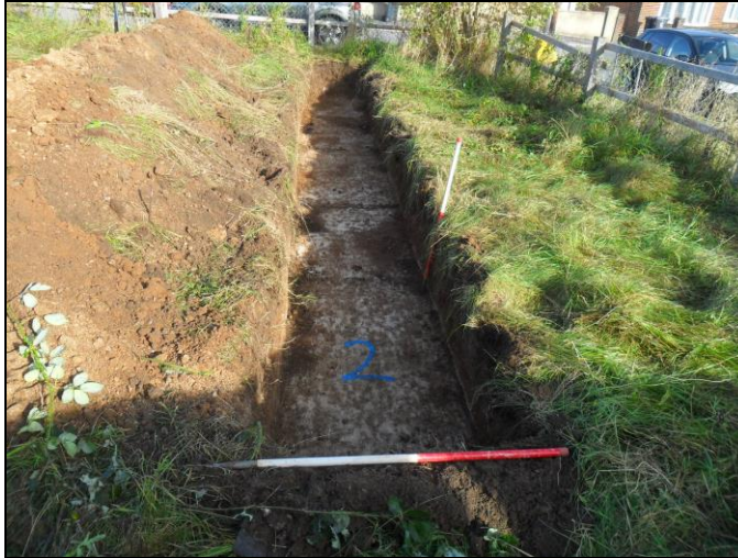
Photograph 2: Trench 2 looking north
