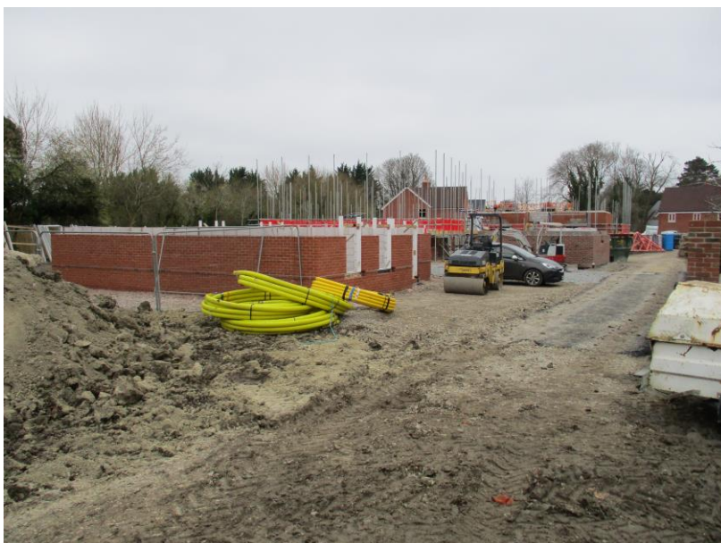
Photograph Taken During Site Visit 19 th March 2019
