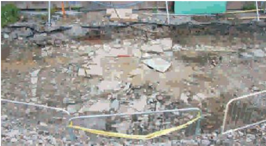
WEST FACING SHOT OF AREA 2
