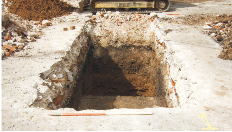
NORTHWEST FACING SHOT TRENCH 1
