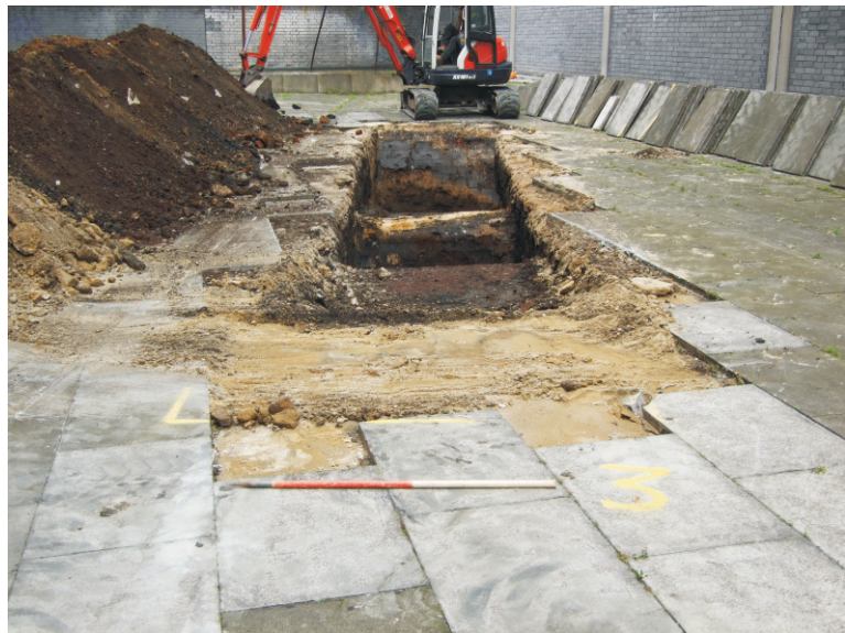
WEST FACING SHOT TRENCH 3
