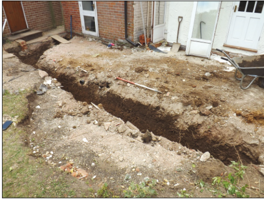
PHOTOGRAPH 1: NORTH FACING REPRESENTATIVE SECTION 001
