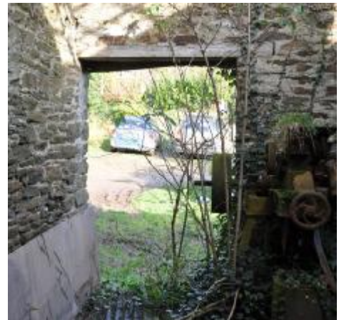
077: BUILDING 2, INTERNAL: NE WALL, DOOR 5, NE FACING.
