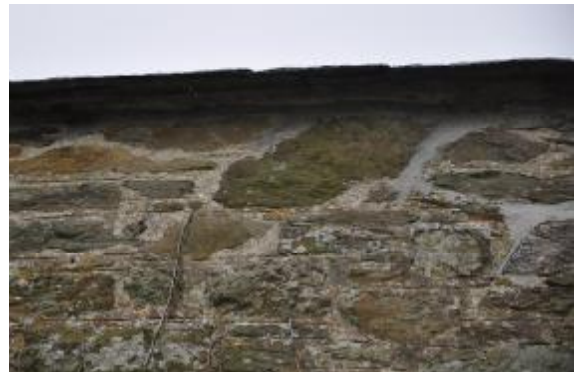
015: NORTHEAST ELEVATION, BUILDING 1: DETAIL OF UNDER EAVE. SW FACING.
