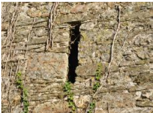
043: SOUTHWEST ELEVATION: BUILDING 1, WINDOW 10 DETAIL.
