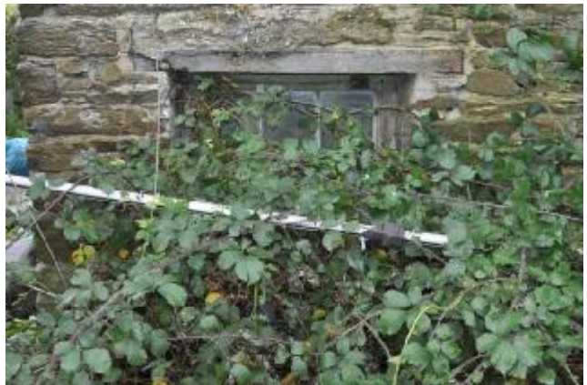
025: NW ELEVATION, BUILDING 1: WINDOW 6 DETAIL, SE FACING.
