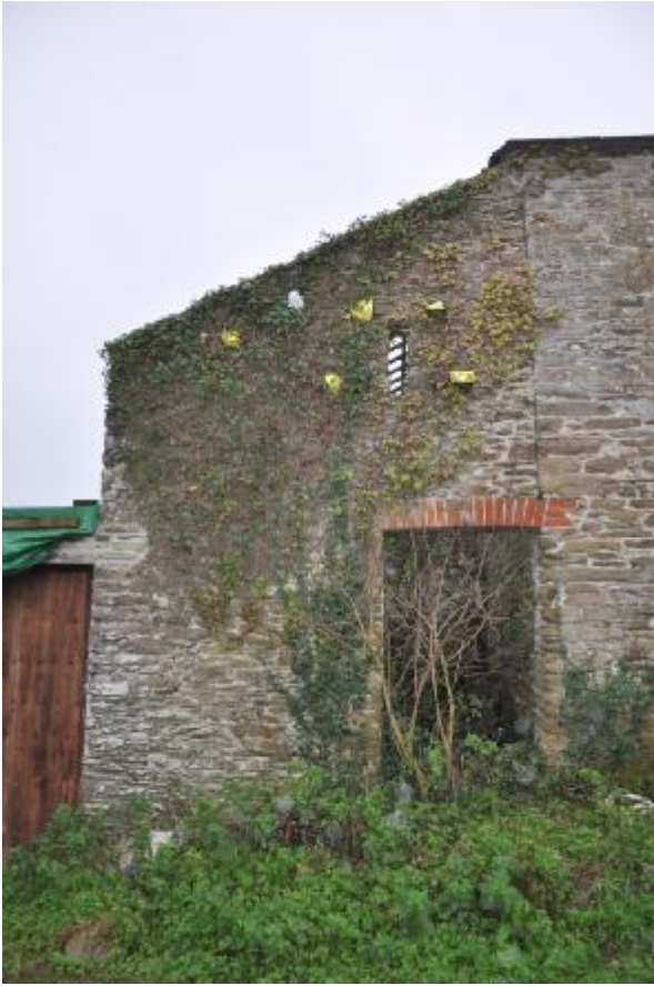
016: NORTHEAST ELEVATION OF BUILDING 2, SW FACING.
