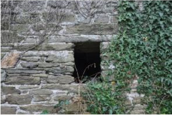
008: NORTHEAST ELEVATION: WINDOW 3, SW FACING.
