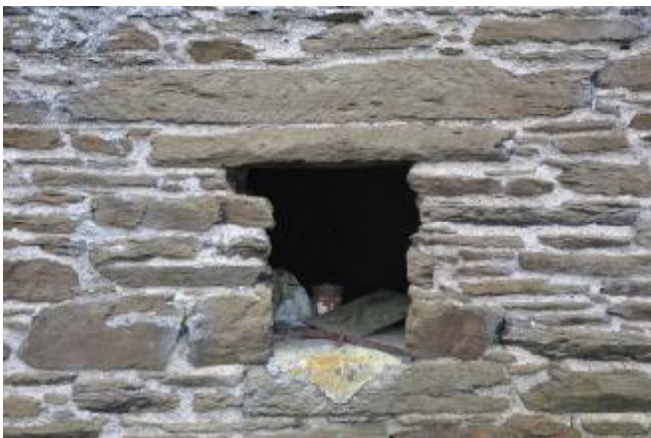
005: NORTHEAST ELEVATION: WINDOW 2. SW FACING.
