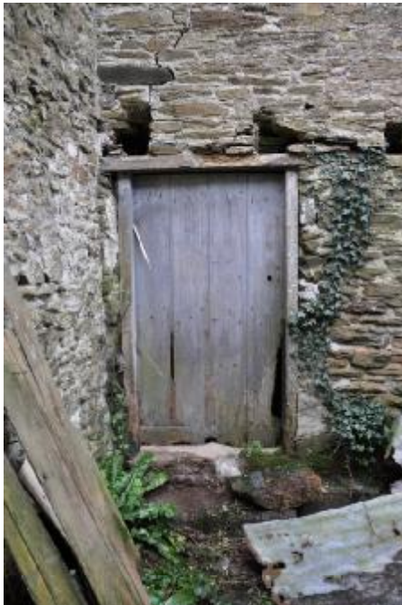
087: BUILDING 2, INTERNAL/BUILDING 1 SE ELEVATION: DOOR 3. NW FACING.
