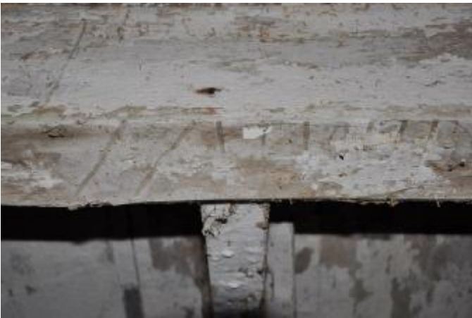
069: BUILDING 1, INTERNAL: CARPENTER MARK ON JOIST. SE FACING.
