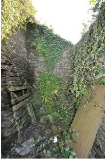
099: EXTENSION 1, INTERNAL: NE, SE AND SW WALLS. SE FACING.
