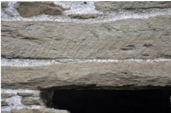
006: NORTHEAST ELEVATION: WINDOW 2, LINTEL DETAIL. SW FACING.
