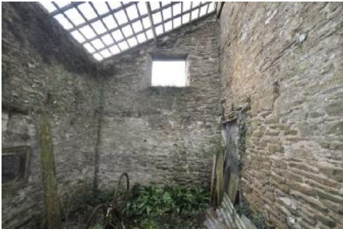
075: BUILDING 2, INTERNAL: SW WALL, SW FACING.
