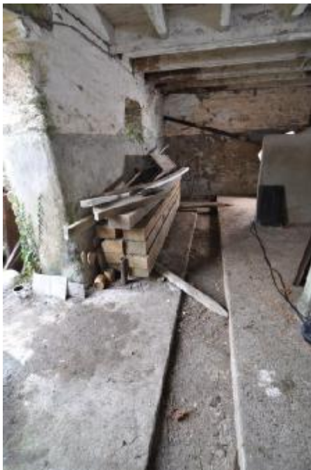
065: BUILDING 1, INTERNAL: DAIRY DRAINAGE GULLY. SE FACING.
