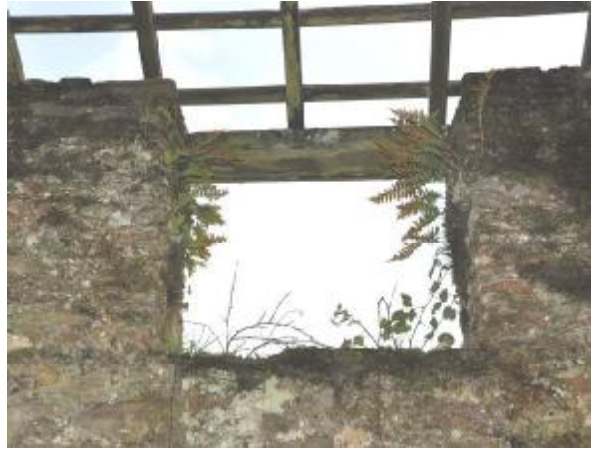
080: BUILDING 2, INTERNAL: SE WALL, WINDOW 14. SE FACING.
