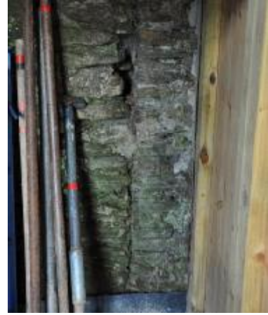
072: BUILDING 2: SE ELEVATION, BUTT JOINT, NW FACING.
