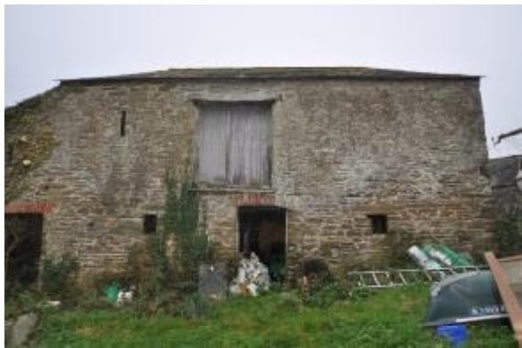
002: NORTHEAST ELEVATION: GENERAL SHOT BUILDING 1. SW FACING.
