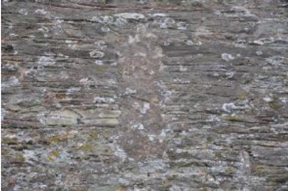
010: NORTHEAST ELEVATION: WINDOW 5, SW FACING.
