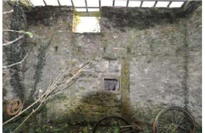
074: BUILDING 2, INTERNAL: SE WALL, SE FACING.
