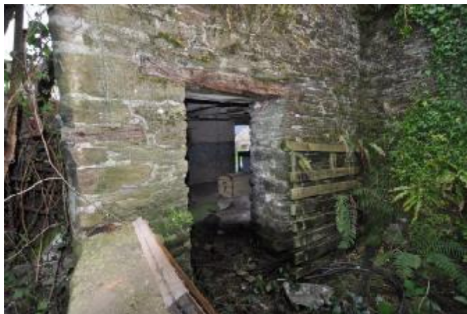
101: EXTENSION 1, INTERNAL/BUILDING 1, SW ELEVATION: DOOR 2. ENE FACING.
