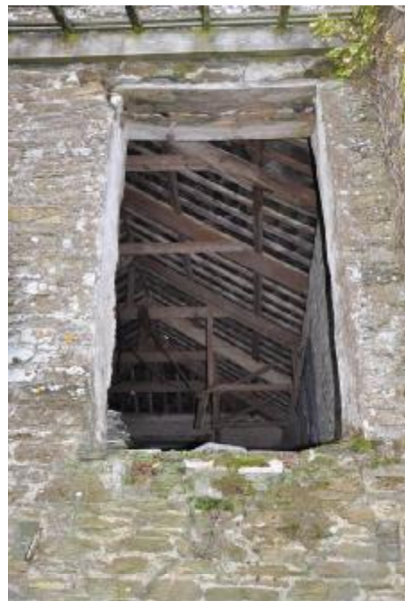
088: BUILDING 2, INTERNAL/BUILDING 1 SE ELEVATION: WINDOW 11. NW FACING.
