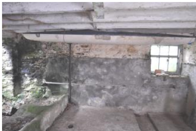
056: BUILDING 1, INTERNAL: NW WALL. NW FACING.
