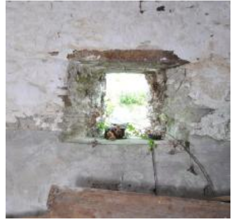
062: BUILDING 1, INTERNAL: NE WALL, WINDOW 2. NE FACING.
