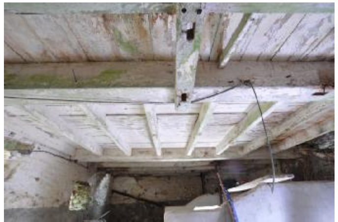
064: BUILDING 1, INTERNAL: CEILING. NW FACING.
