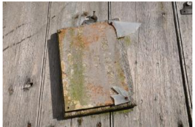
042: SOUTHWEST ELEVATION: BUILDING 1, DETAIL SHOWING PLAQUE ON DOOR 4.
