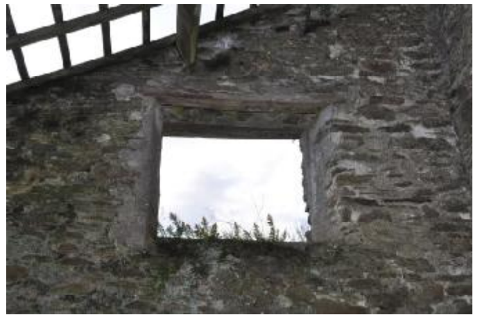
082: BUILDING 2, INTERNAL: SW WALL, WINDOW 15. SW FACING.
