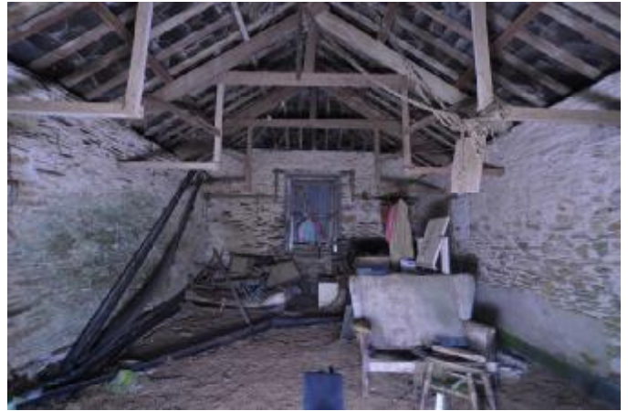
092: BUILDING 1, FIRST FLOOR INTERNAL: NW WALL, NW FACING.
