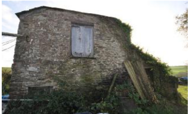
023: NW ELEVATION, BUILDING 1 AND EXTENSION 1, SE FACING.
