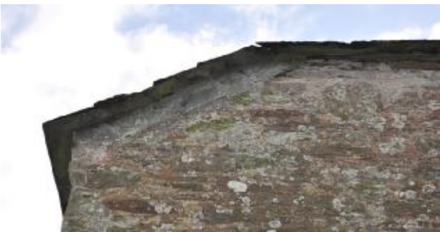
026: NW ELEVATION, BUILDING 1: ROOF DETAIL, SW SIDE.
