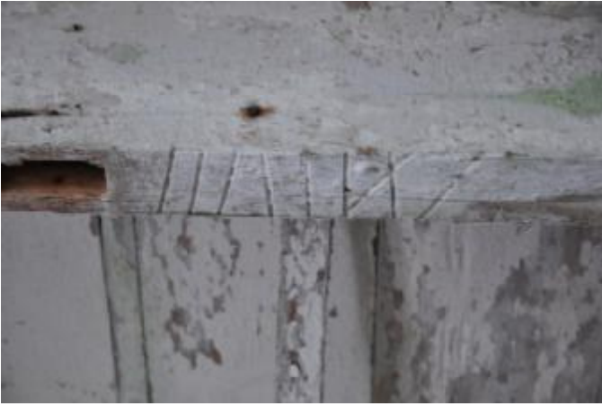
067: BUILDING 1, INTERNAL: CARPENTER MARK ON JOIST. SE FACING.
