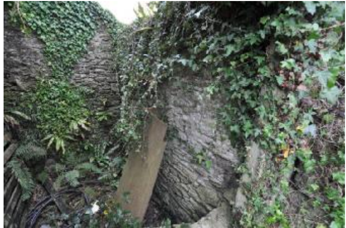
100: EXTENSION 1, INTERNAL: SE AND SW WALLS. SSE FACING.
