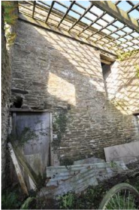
085: BUILDING 2, INTERNAL/BUILDING 1 SE ELEVATION. N FACING.
