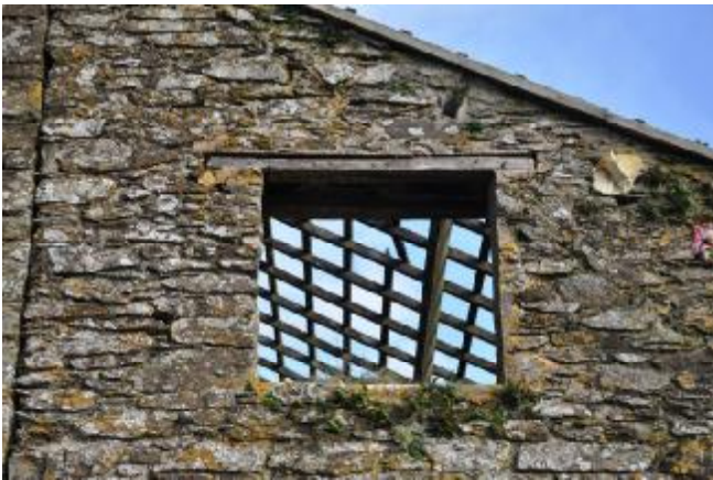
045: SOUTHWEST ELEVATION: BUILDING 2, WINDOW 15, NE FACING.
