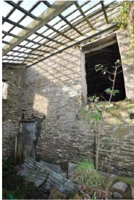
086: BUILDING 2, INTERNAL/BUILDING 1 SE ELEVATION. S FACING.
