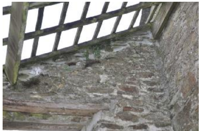
084: BUILDING 2, INTERNAL: SW WALL, ROOF DETAIL. SW FACING.
