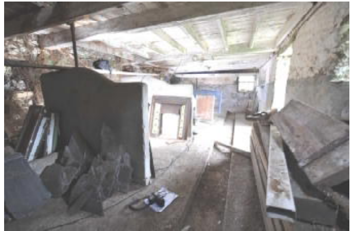
048: BUILDING 1, INTERNAL: GENERAL SHOT. W FACING.
