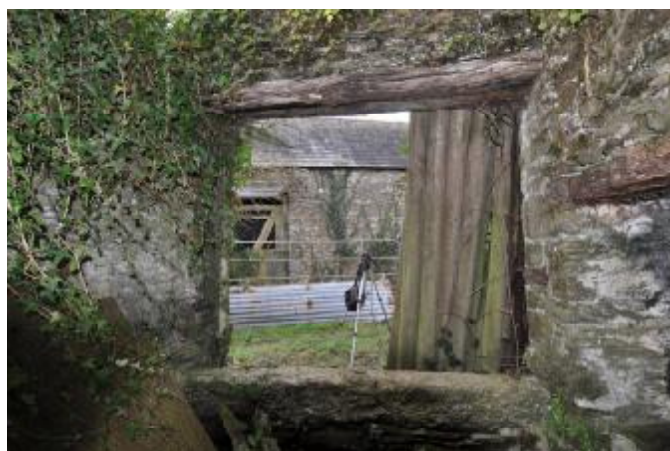
102: EXTENSION 1, INTERNAL: WINDOW 16. NW FACING.
