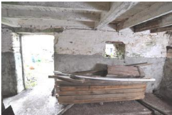
059: BUILDING 1, INTERNAL: NE WALL, SE END. NE FACING.
