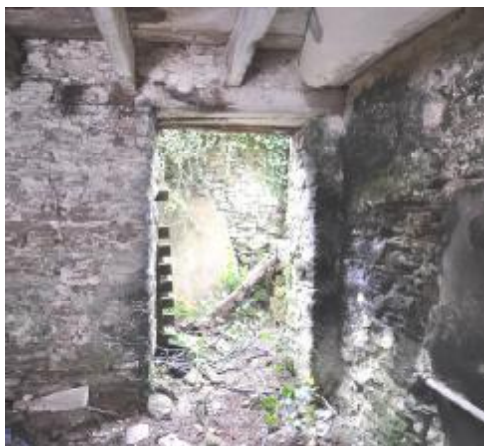
056: BUILDING 1, INTERNAL: SW WALL, DOOR 2 DETAIL. SW FACING.
