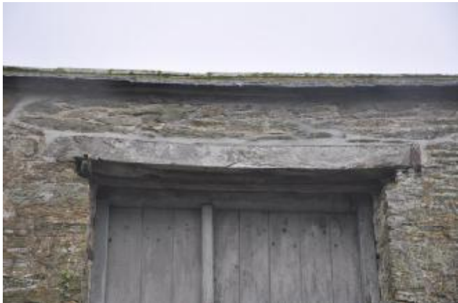
004: NORTHEAST ELEVATION: WINDOW 1 LINTEL DETAIL. SW FACING
