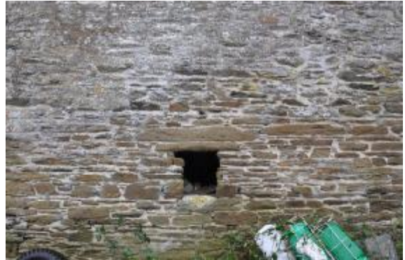
011: NORTHEAST ELEVATION: DETAIL SHOWING CHANGE IN STONEMWORK BETWEEN UPPER AND LOWER FLOOR
