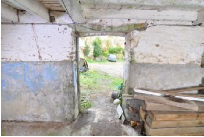
061: BUILDING 1, INTERNAL: NE WALL, DOOR 1. NE FACING.
