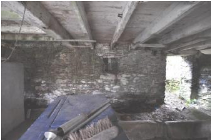
054: BUILDING 1, INTERNAL: SW WALL, SE END. SW FACING.
