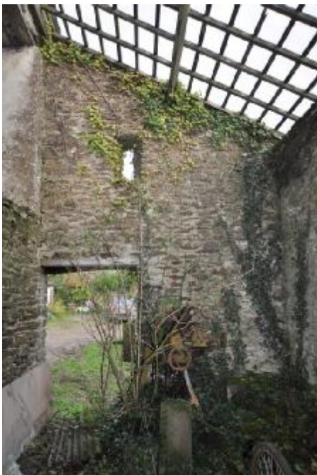
076: BUILDING 2, INTERNAL: NE WALL AND MILL, NE FACING.
