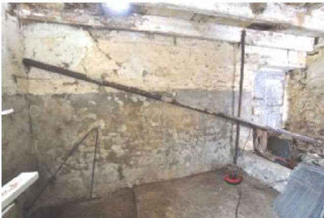
049: BUILDING 1, INTERNAL: SE WALL. S FACING.
