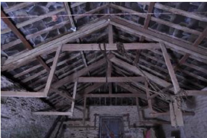
097: BUILDING 1, FIRST FLOOR INTERNAL: ROOF, NW FACING.
