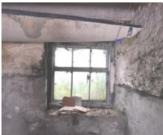
057: BUILDING 1, INTERNAL: NW WALL, WINDOW 6 DETAIL. NW FACING.
