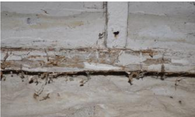
070: BUILDING 1, INTERNAL: CARPENTER MARK ON JOIST. SE FACING.
