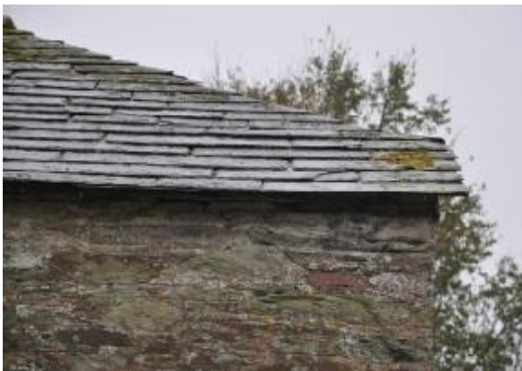
014: NORTHEAST ELEVATION BUILDING 1: UNDER EAVE AND ROOF DETAIL. SW FACING.
