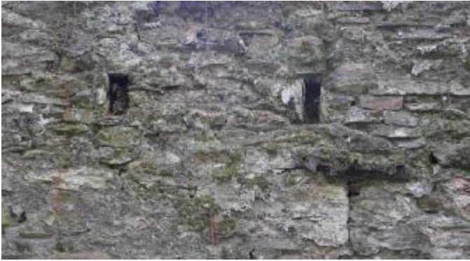
081: BUILDING 2, INTERNAL: SE WALL, WINDOW 14. SE FACING.
