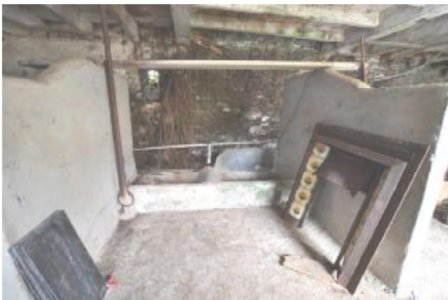
053: BUILDING 1, INTERNAL: DAIRY STALL, SE END. SW FACING.
