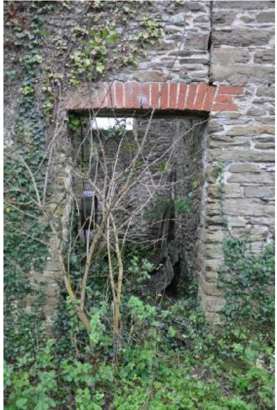
017: NORTHEAST ELEVATION: BUILDING 2, DOOR 5, SW FACING.
