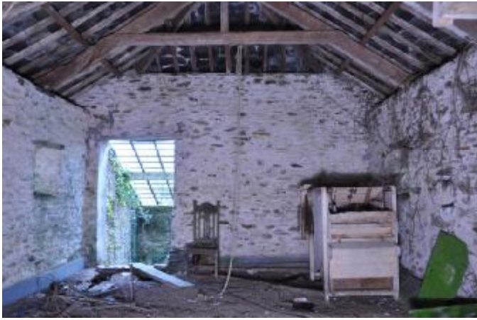
091: BUILDING 1, FIRST FLOOR INTERNAL: SE WALL, SE FACING.
