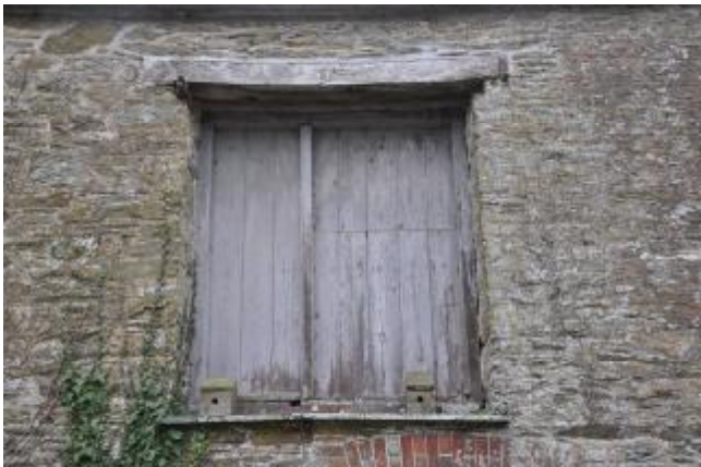
003: NORTHEAST ELEVATION: WINDOW 1 DETAIL. SW FACING.
