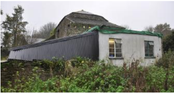
022: SE ELEVATION: N FACING SHOT.
