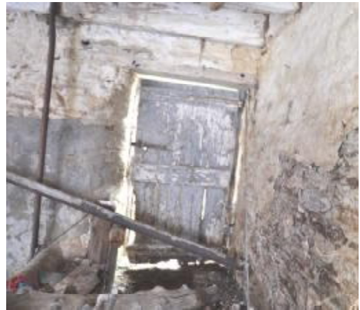
050: BUILDING 1, INTERNAL: SE WALL, DOOR 3. SE FACING.
