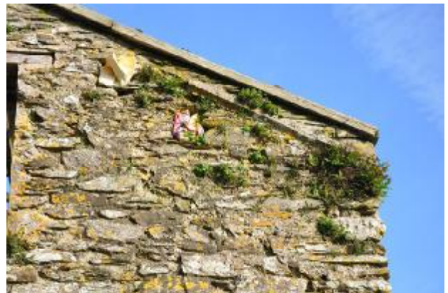
046: SOUTHWEST ELEVATION: BUILDING 2, ROOF LINE DETAIL, NE FACING.
