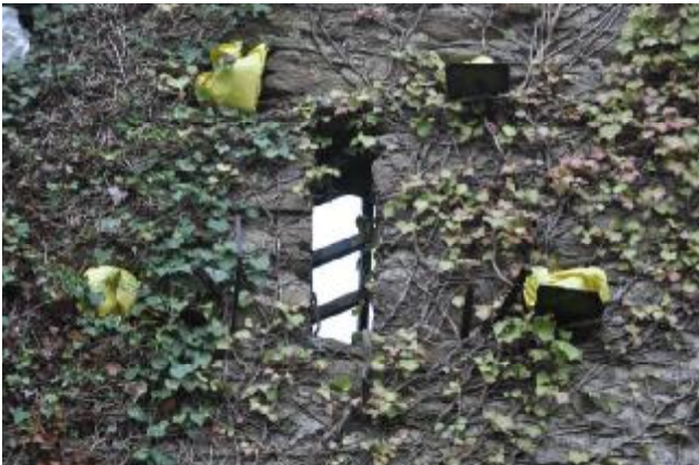
019: NORTHEAST ELEVATION: BUILDING 2, WINDOW 12, SW FACING.
