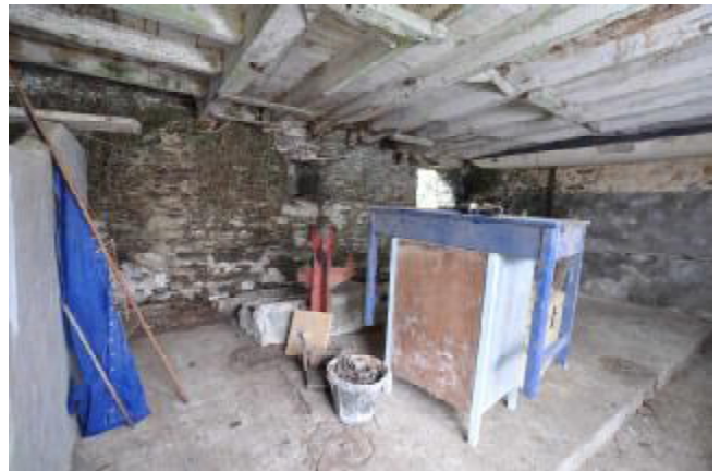
052: BUILDING 1, INTERNAL: SW WALL, NW END. W FACING.
