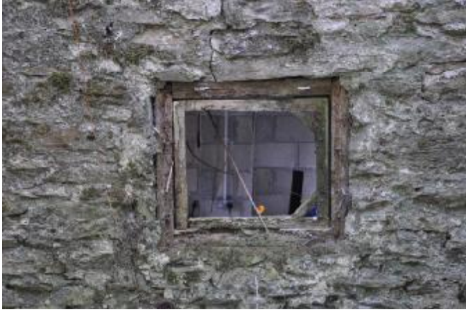
079: BUILDING 2, INTERNAL: SE WALL, WINDOW 13. SE FACING.
