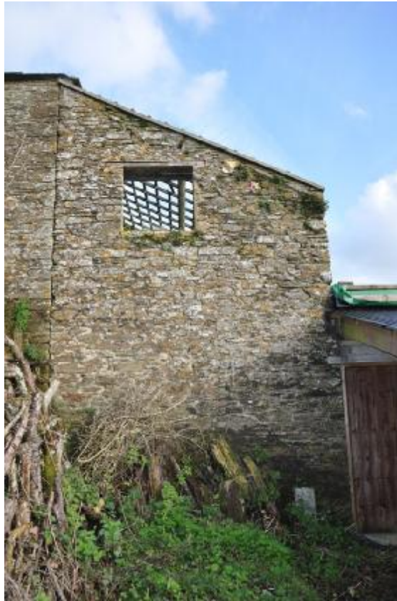
044: SOUTHWEST ELEVATION: BUILDING 2, NE FACING.
