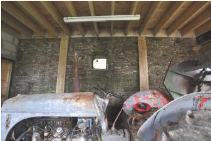
071: BUILDING 2: SE ELEVATION, NW FACING.
