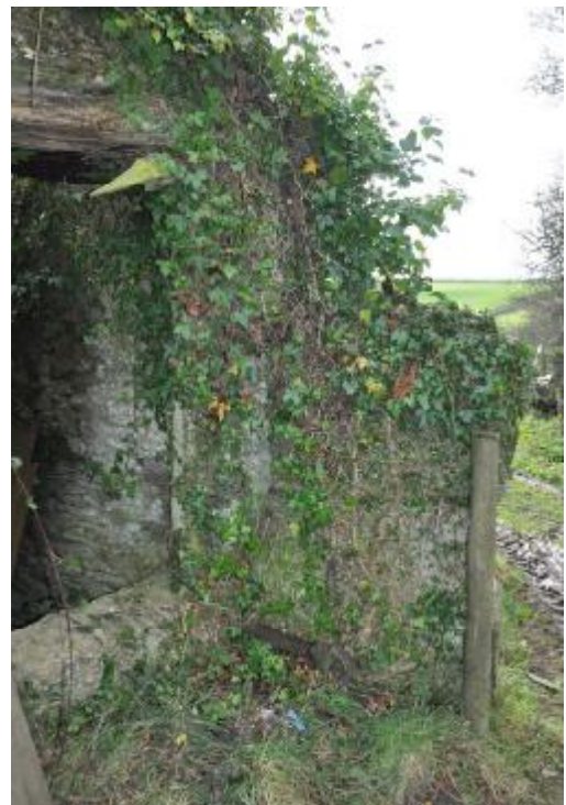
031: NW ELEVATION, EXTENSION 1: STONE WALLING ON WEST CORNER. S FACING SHOT.
