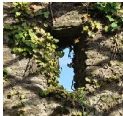
078: BUILDING 2, INTERNAL: NE WALL, WINDOW 12, NE FACING.
