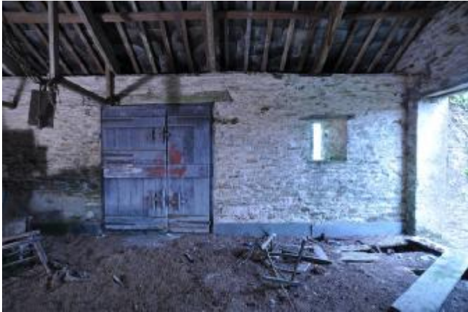
093: BUILDING 1, FIRST FLOOR INTERNAL: NE WALL, SE HALF, NE FACING.
