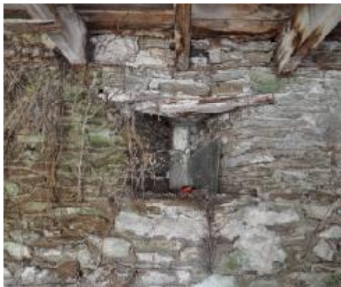
055: BUILDING 1, INTERNAL: SW WALL, WINDOW 8 DETAIL. SW FACING.
