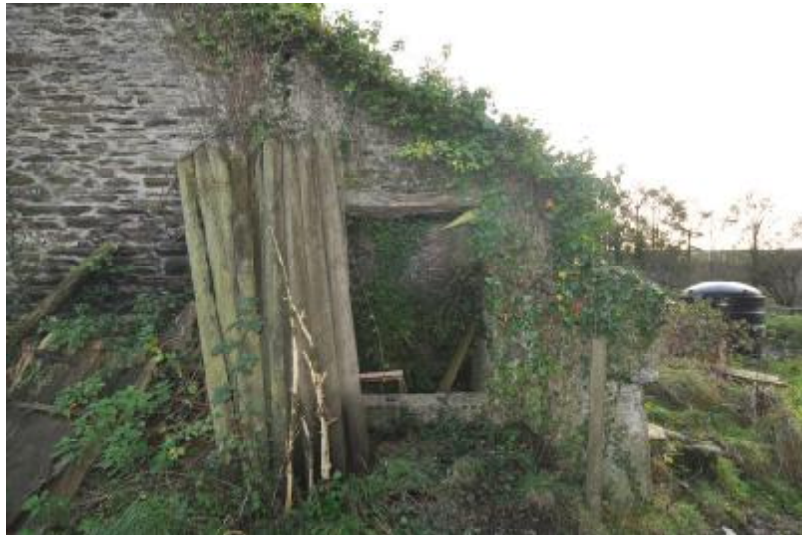
029: NW ELEVATION, EXTENSION 1. SE FACING.
