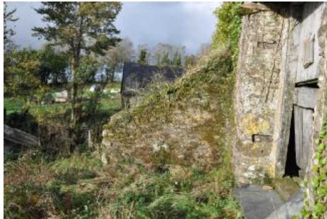
040: SOUTHWEST ELEVATION: EXTENSION 1, SE WALL. NW FACING.
