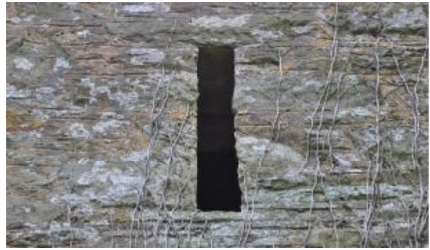
009: NORTHEAST ELEVATION: WINDOW 4, SW FACING.
