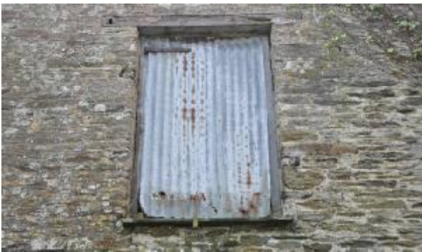
024: NW ELEVATION, BUILDING 1: WINDOW 7 DETAIL, SE FACING.
