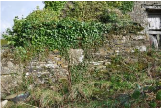
038: SOUTHWEST ELEVATION: EXTENSION 1. NE FACING.
