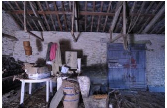
094: BUILDING 1, FIRST FLOOR INTERNAL: NE WALL, NW HALF, NE FACING.
