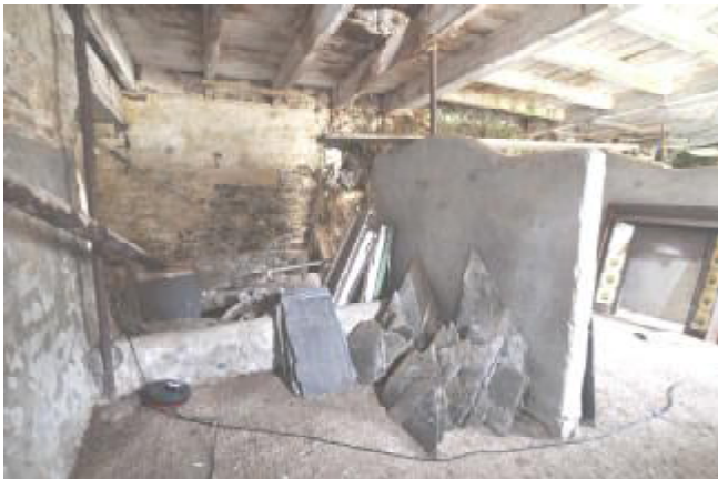
051: BUILDING 1, INTERNAL: SW WALL, SE END AND DAIRY STALL. SW FACING.
