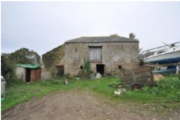
001: NORTHEAST ELEVATION: GENERAL SHOT. SW FACING.
