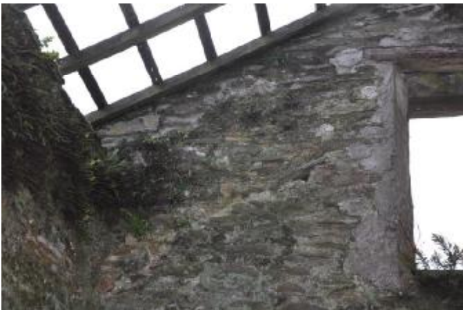
083: BUILDING 2, INTERNAL: SW WALL, ROOF DETAIL. SW FACING.
