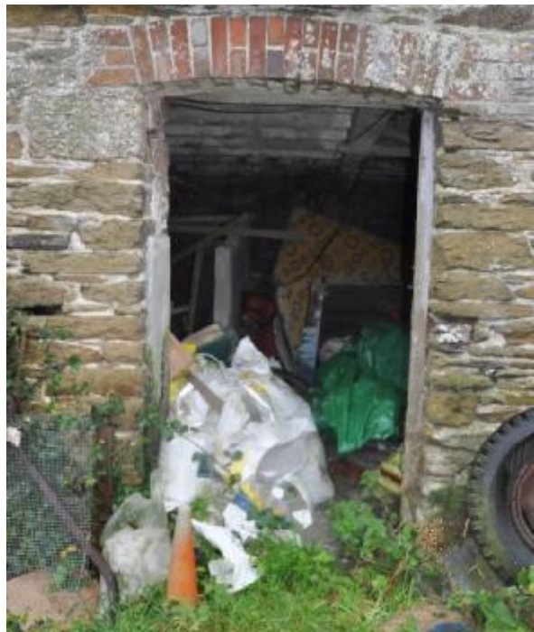
007: NORTHEAST ELEVATION: DOOR 1. SW FACING.
