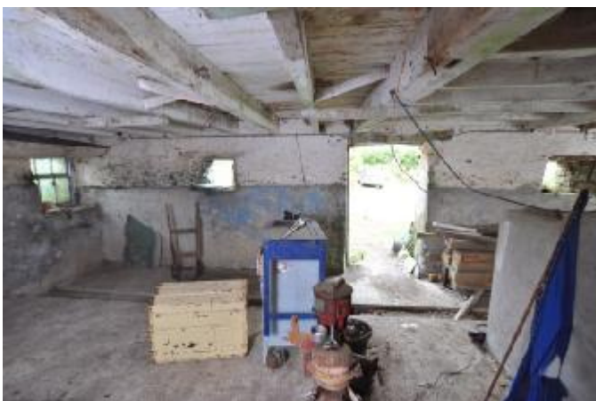
058: BUILDING 1, INTERNAL: NE WALL, NW END. NE FACING.
