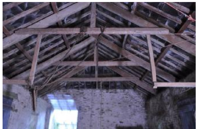
098: BUILDING 1, FIRST FLOOR INTERNAL: ROOF, SE FACING.
