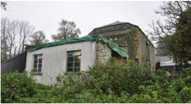
020: SE ELEVATION: W FACING SHOT.
