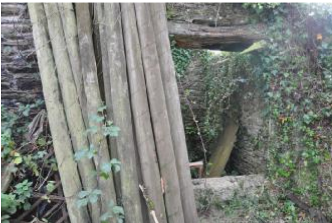
030: NW ELEVATION, EXTENSION 1, WINDOW 16. SE FACING.
