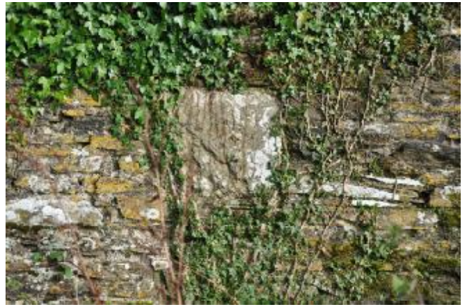
039: SOUTHWEST ELEVATION: EXTENSION 1, WINDOW 17. NE FACING.
