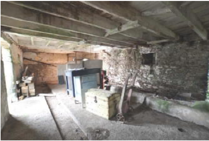
047: BUILDING 1, INTERNAL: GENERAL SHOT. SSE FACING.
