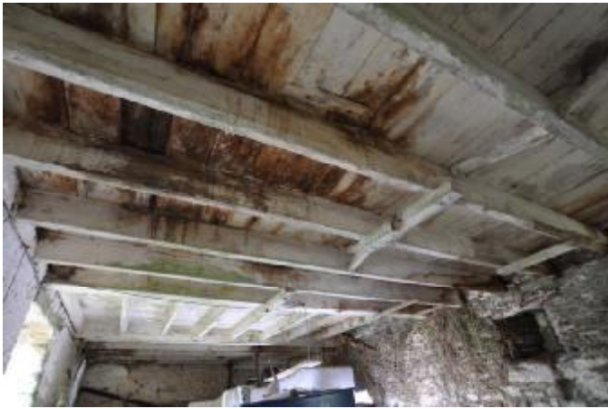
063: BUILDING 1, INTERNAL: CEILING. SE FACING.
