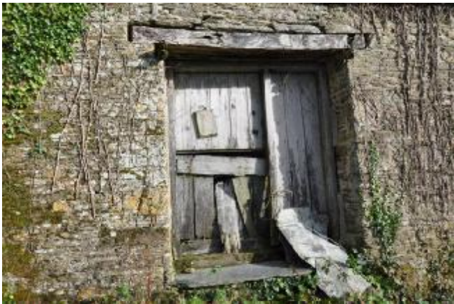
041: SOUTHWEST ELEVATION: BUILDING 1, DOOR 4 DETAIL. NE FACING.
