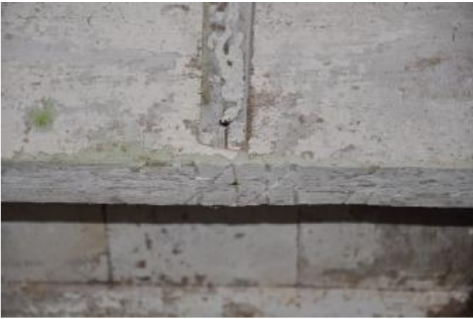
068: BUILDING 1, INTERNAL: CARPENTER MARK ON JOIST. SE FACING.
